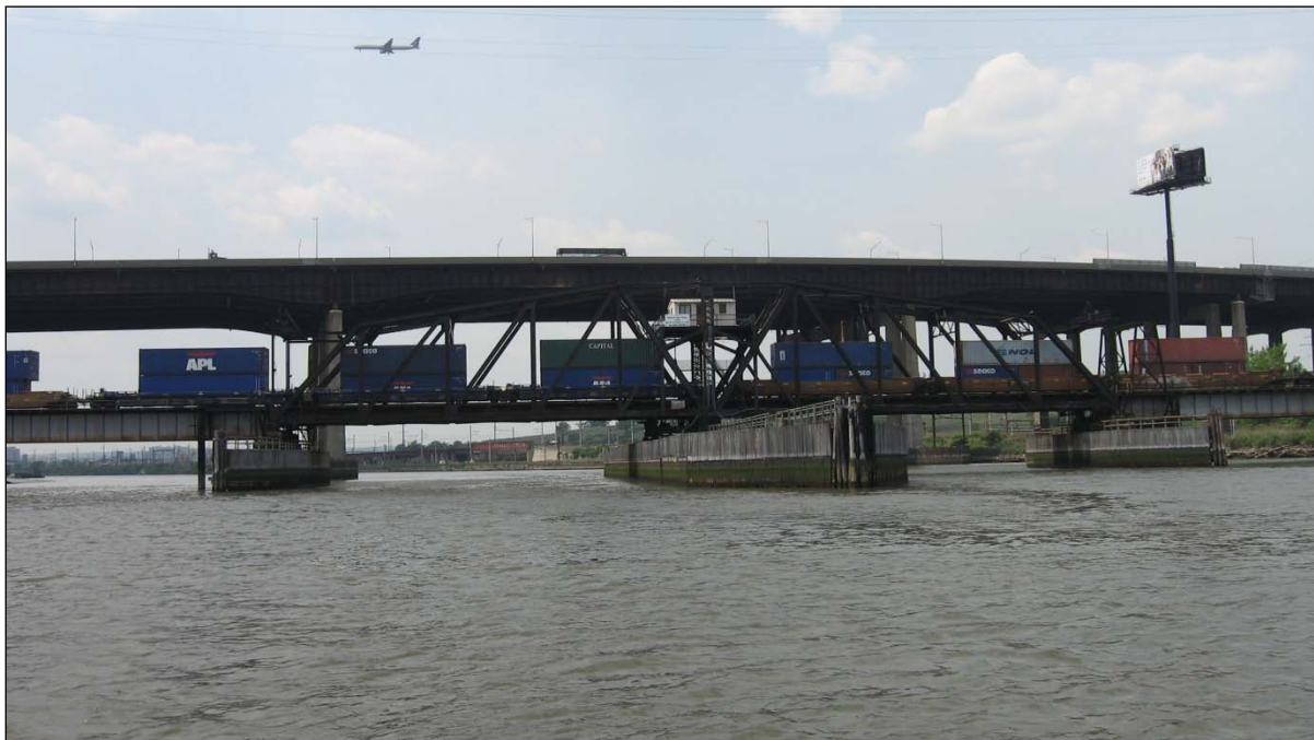
Figure 4. View Upstream to the Point-No-Point Conrail Bridge & NJ Turnpike Bridge, May 2007.
