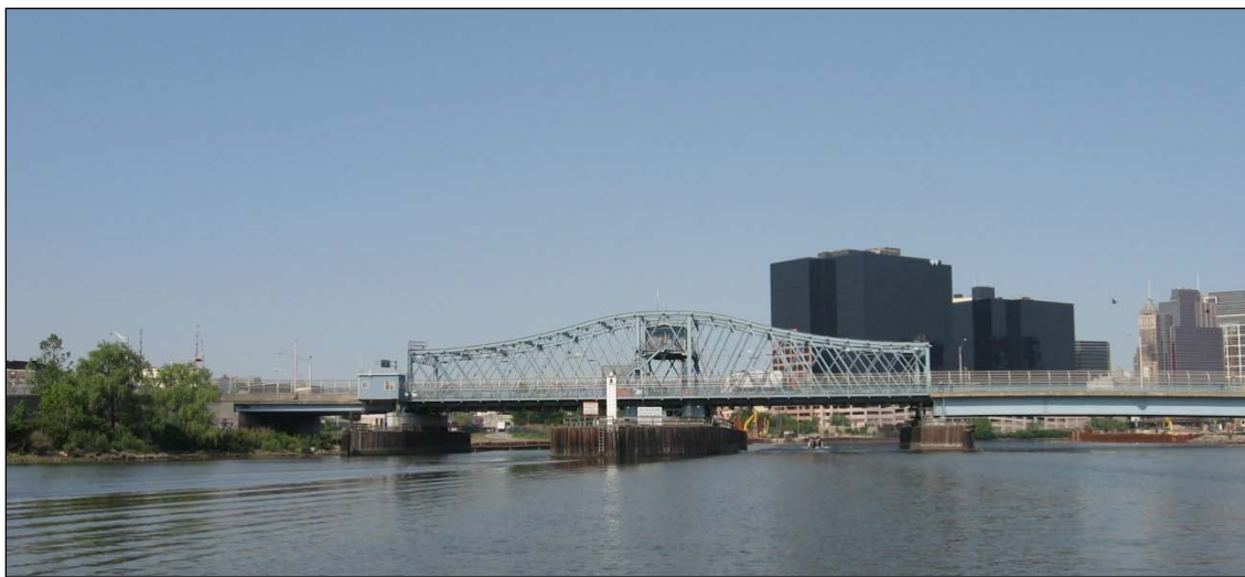
Figure 2. Downstream View of Jackson Street Bridge and the City of Newark, May 2007.
