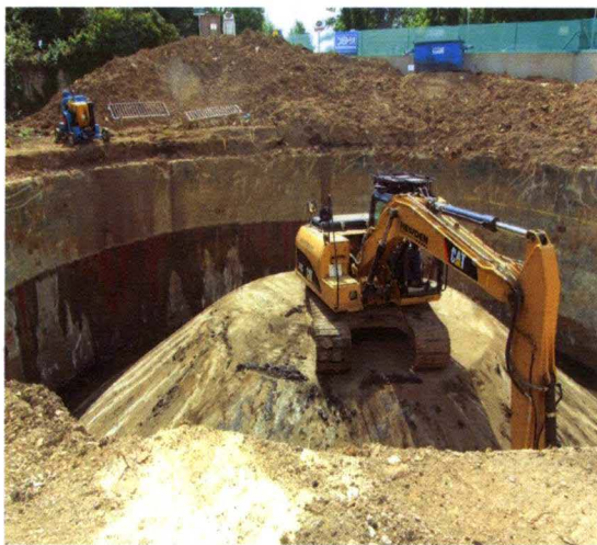
Figure 11. Excavation of a backfilled concrete gasholder tank with dumpling.
