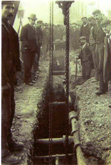
Figure 17. Repairing the gas mains in Victorian times.
