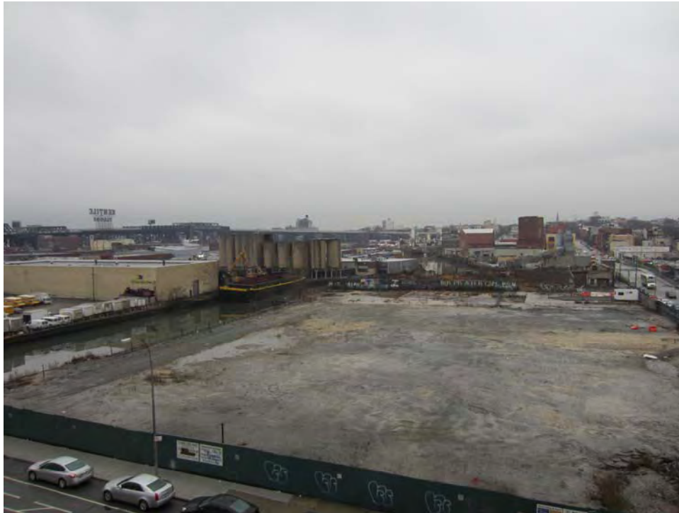
IMG 2. WFM site flooding after a typical rain storm (12/7/11)
