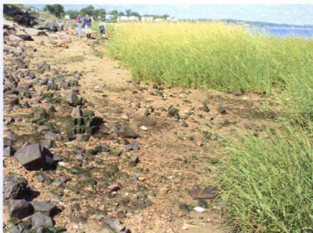
Figure 4: Intertidal Zone Along Seawall
