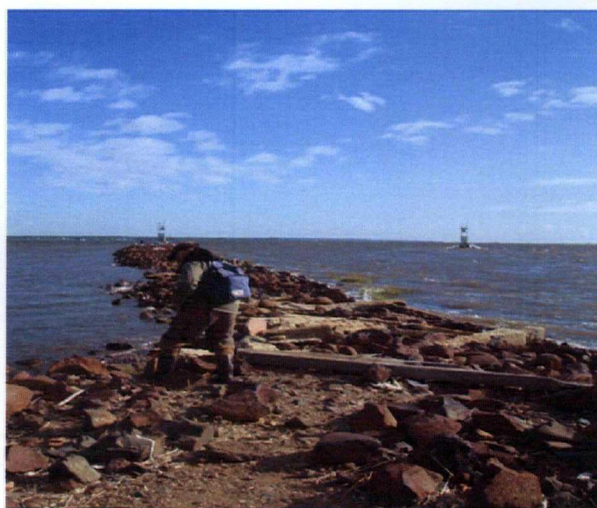
Figure 7: Cheesequake Creek Inlet Western Jetty
