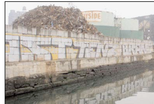
Concrete bulkheads atop timber cribwork
