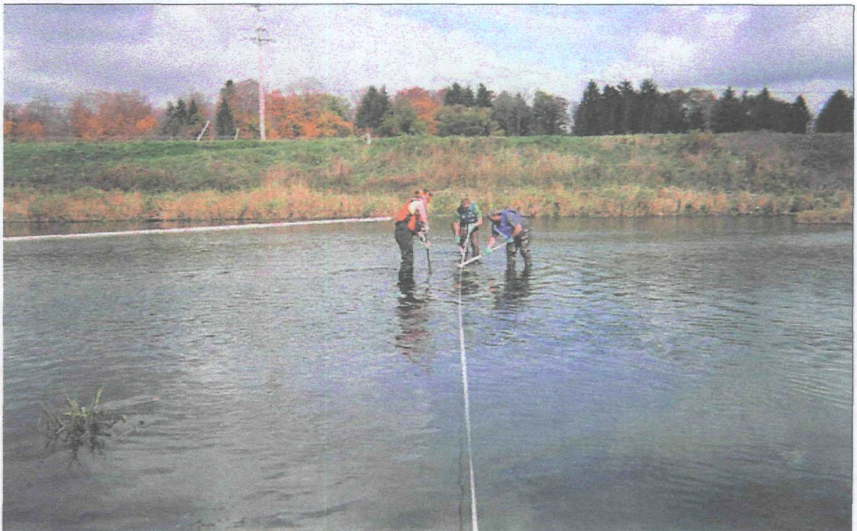
Status as of: 10/16/00 Description: View of oil absorbent booms transversing Genesee River. Photo by: Eric Mysona
