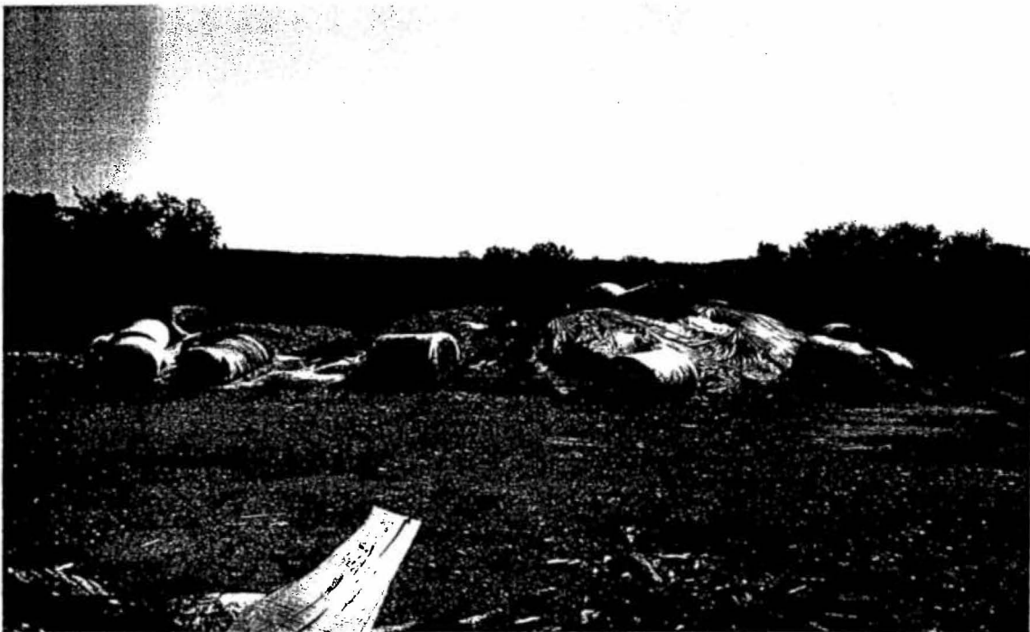
July 31, 2007: Bales of hay holding down plastic tarps which cover some of the piles of construction debris.
