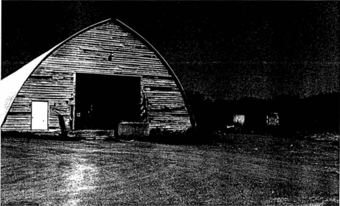
July 31, 2007: View of barn, looking west.
