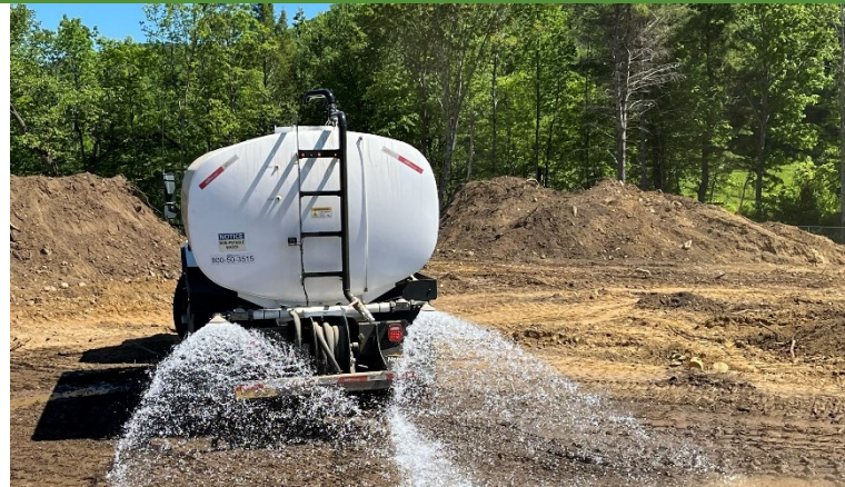
Image 1: Water truck dispersing water for dust mitigation. Lenox town water is used from an onsite fire hydrant.
