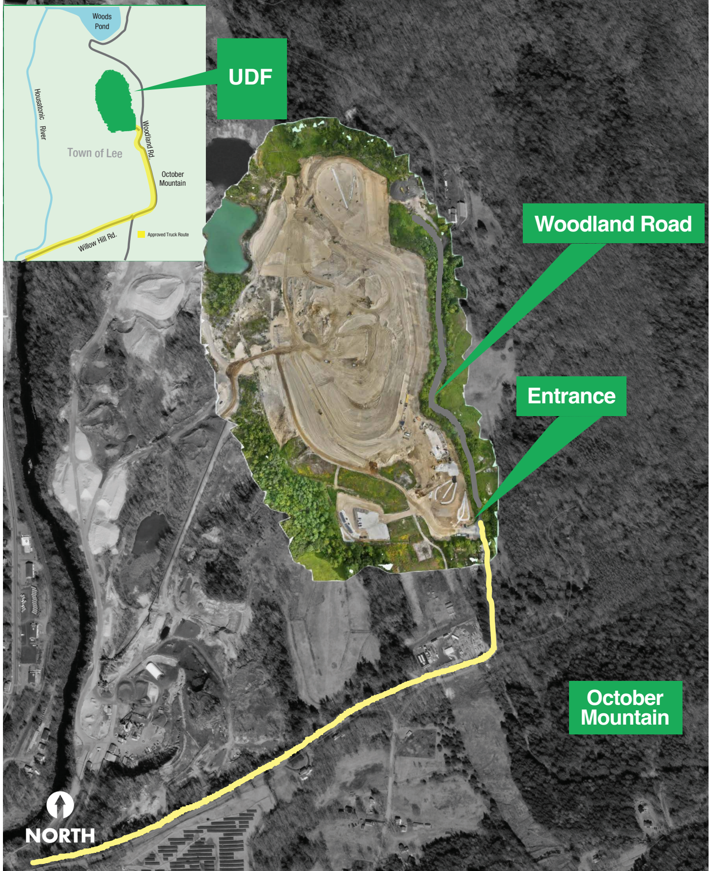
Figure1: Aerial photograph of the Upland Disposal Facility in Lee, MA. Image highlights haul roads and progress of work as of August 2026.
