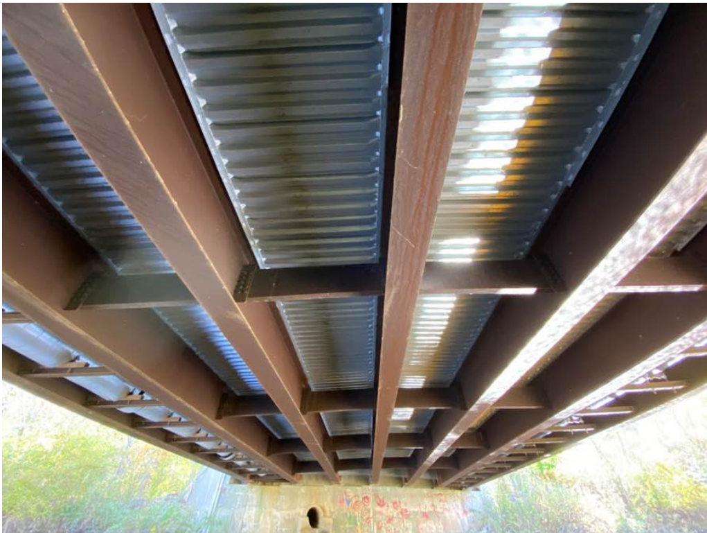
Photo 2: Typical underside, looking east.
