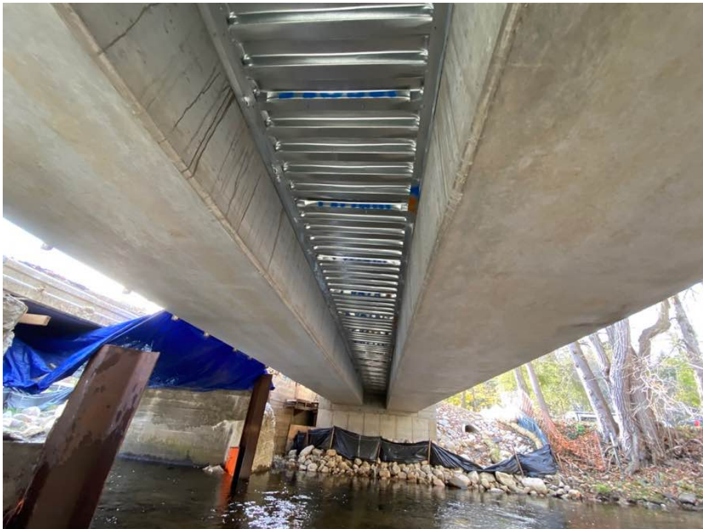
Photo 2: General underside, looking south.
