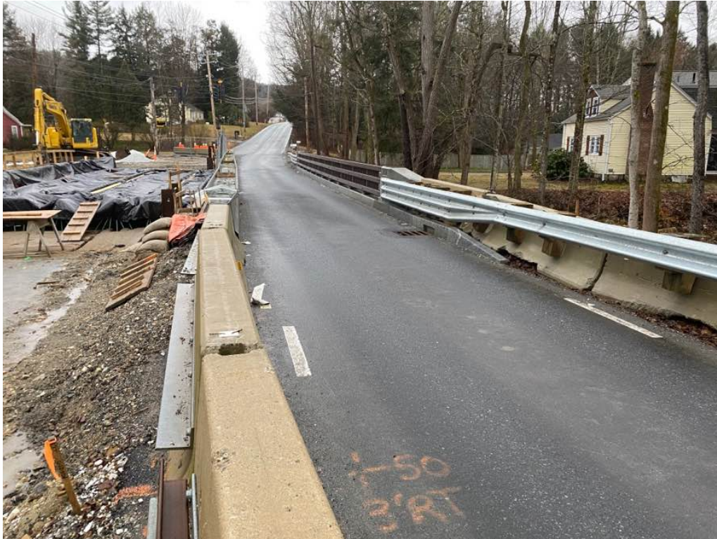
Photo 1: General topside, looking south.
