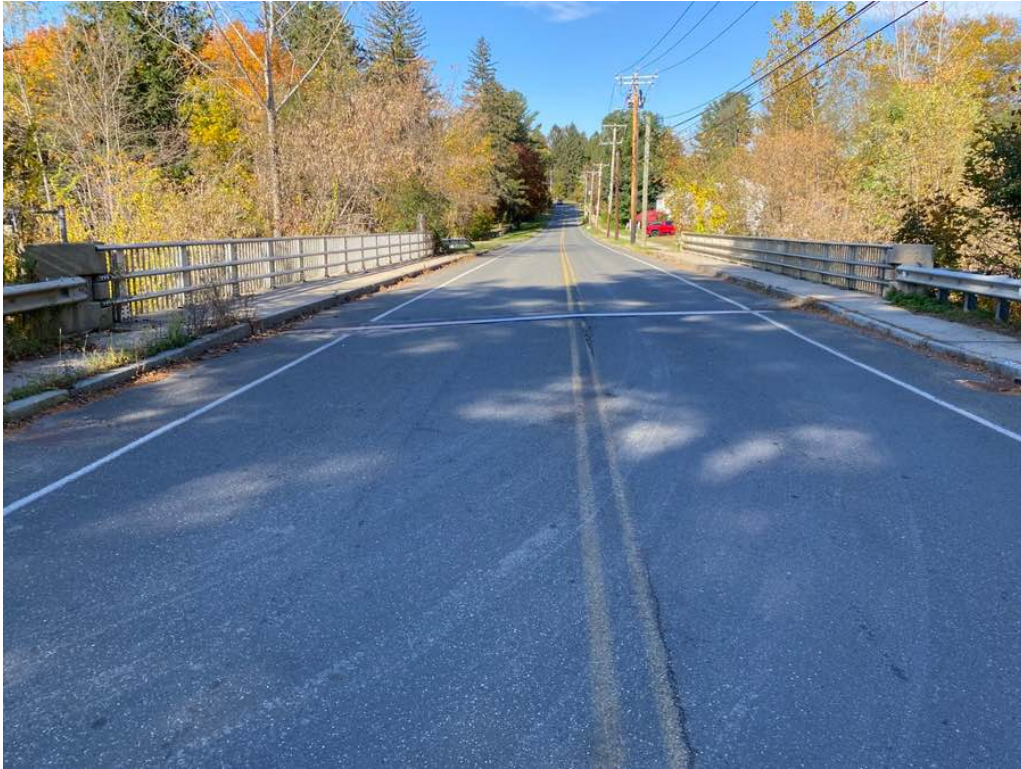
Photo 1: General topside, looking west.
