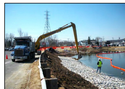
Photo 2: Installation of cap materials with an excavator
