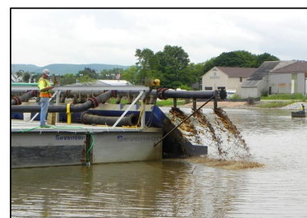
Photo 1: Installation of cap materials with the barge and spreader bar
