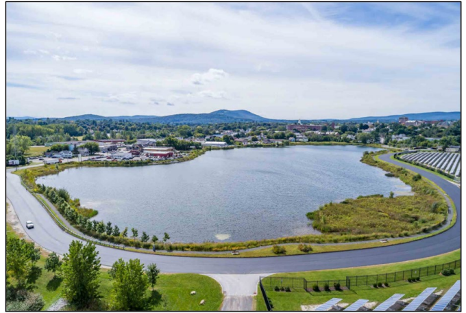
Photo: View of Silver Lake following remediation.
