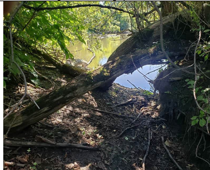
Outlet from backwater at Station 86, left bank
