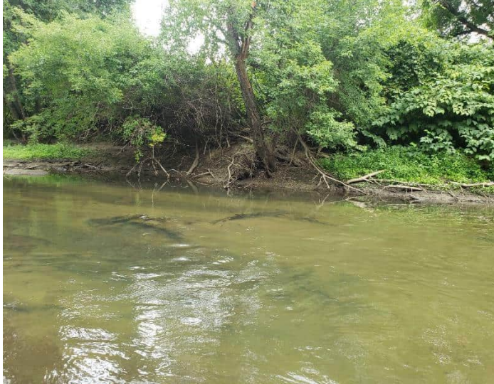
Left bank near Station 222
