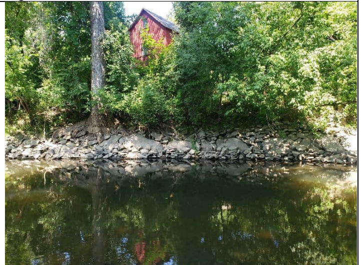
Left bank at Station 55
