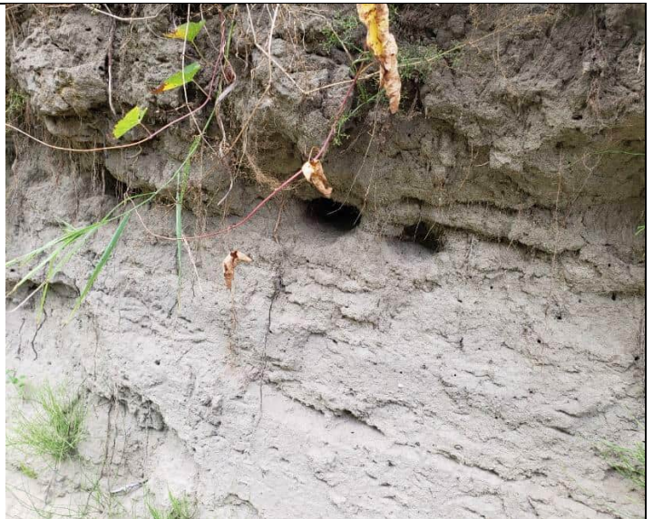
Left bank near Station 233; bank swallow cavities
