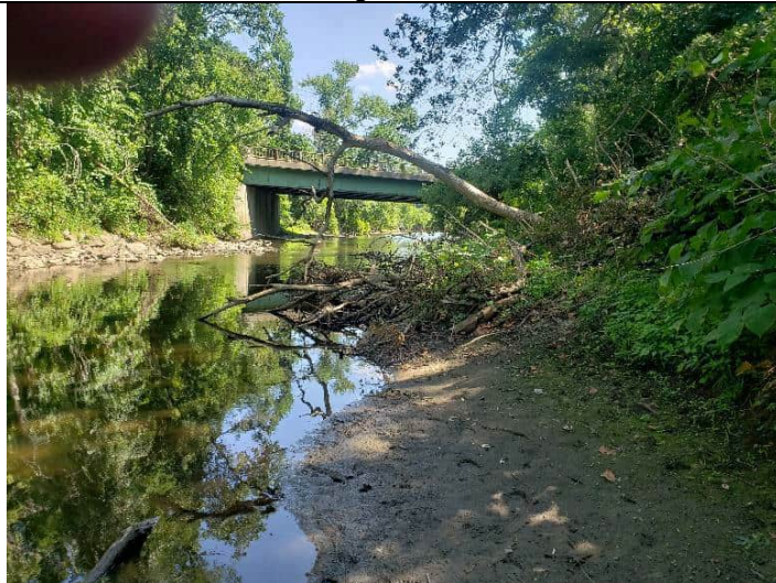
Right bank from Station 55 looking downstream
