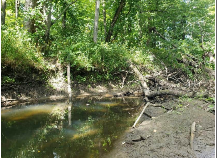
Right bank around Station 174
