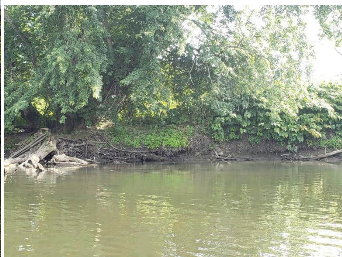
Right bank near Station 245
