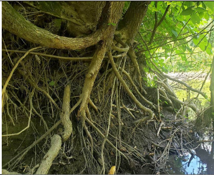
Right bank, looking upstream
