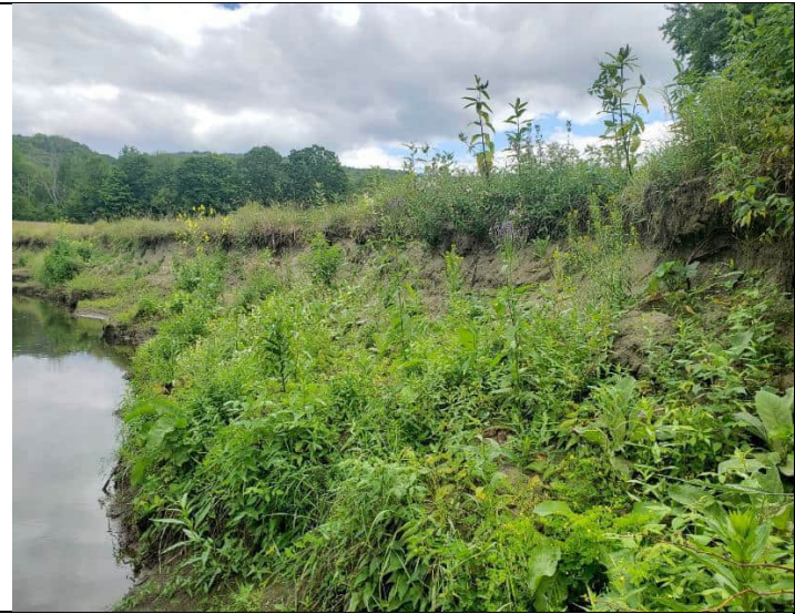
Left bank looking upstream around Station 234
