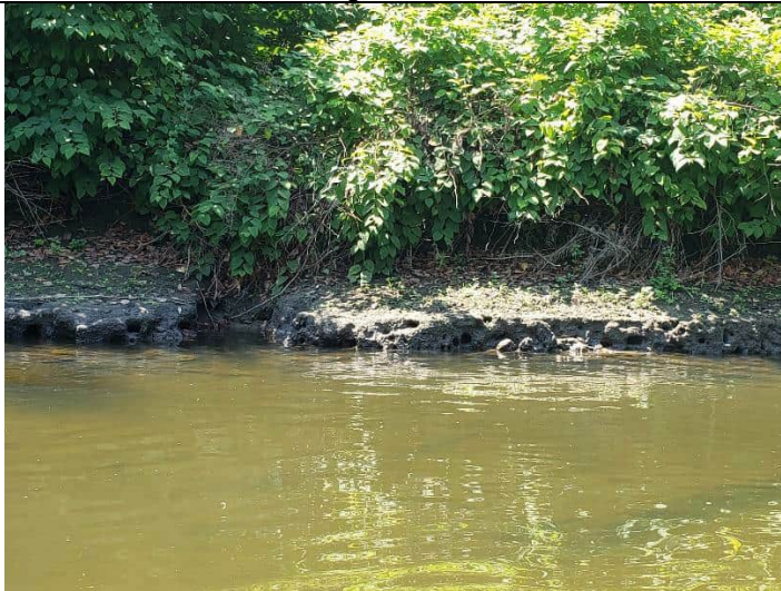
Right bank just below Morewood tributary
