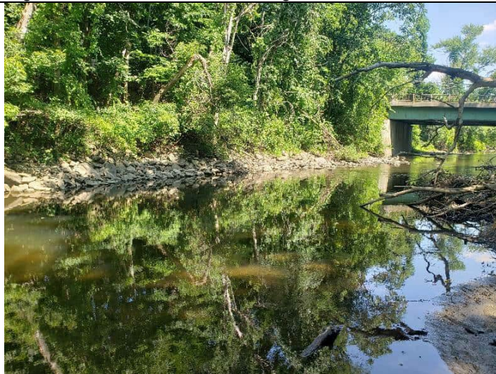
Left bank at Station 55-56
