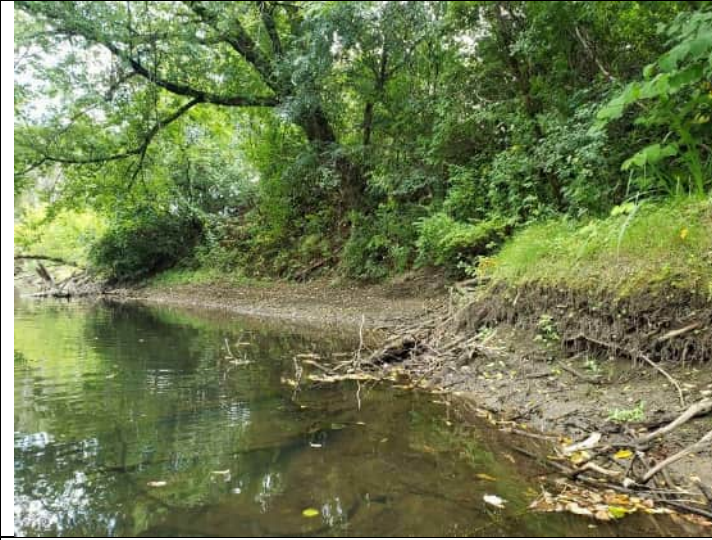
Left bank around Station 108
