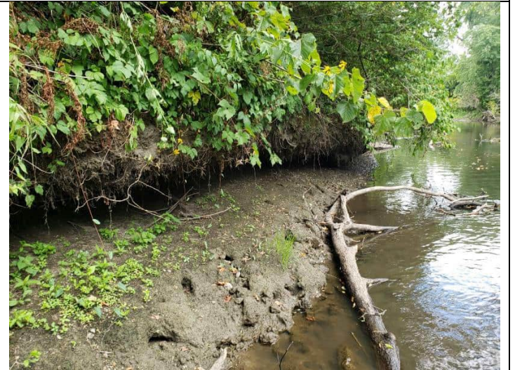
Left bank undercutting
