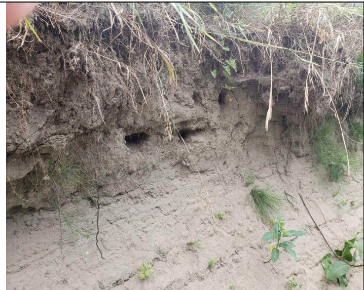
Left bank near Station 233; bank swallow cavities
