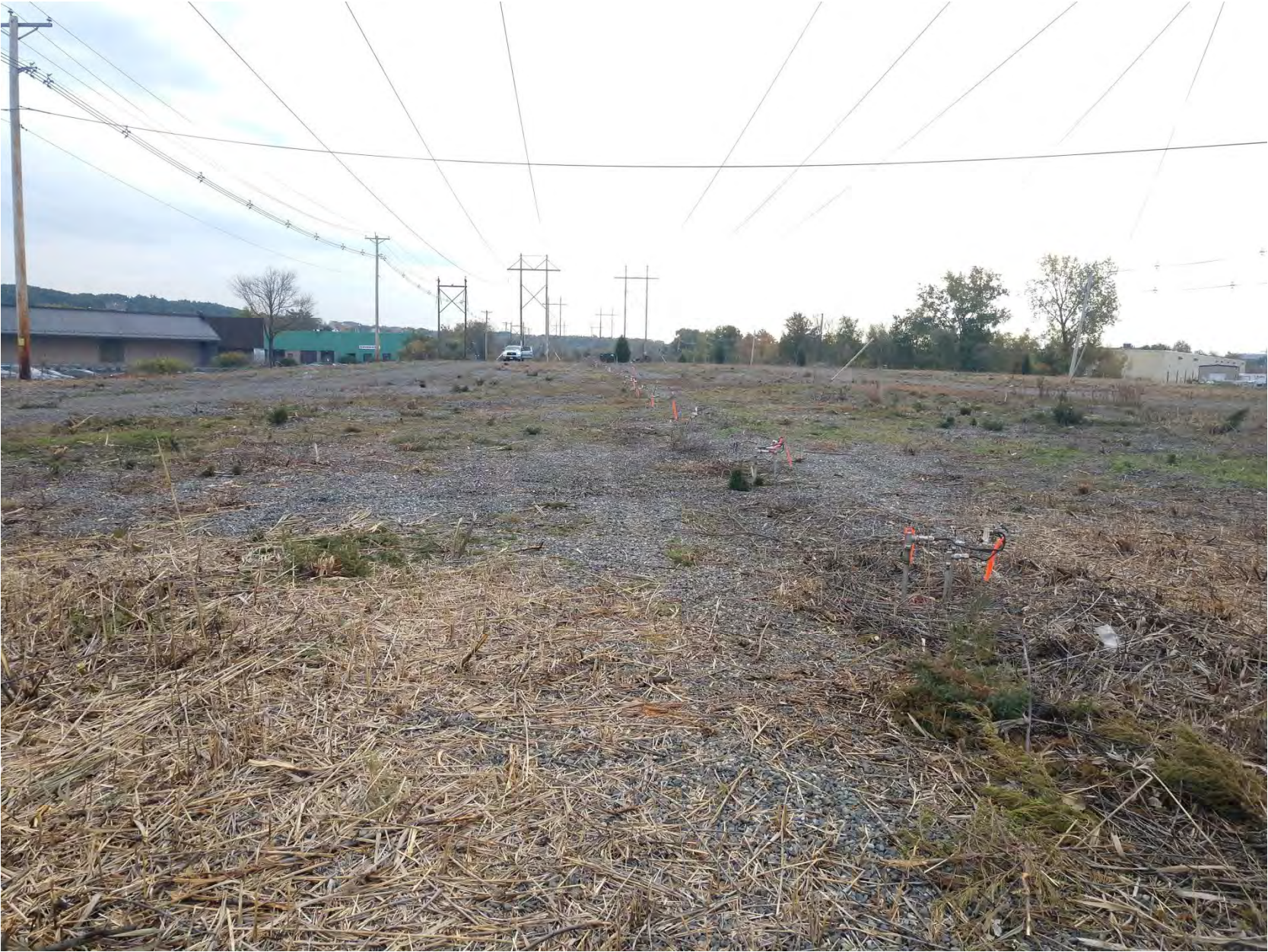
Boston Edison (NSTAR) Right of Way – typical engineered gravel cover system.
