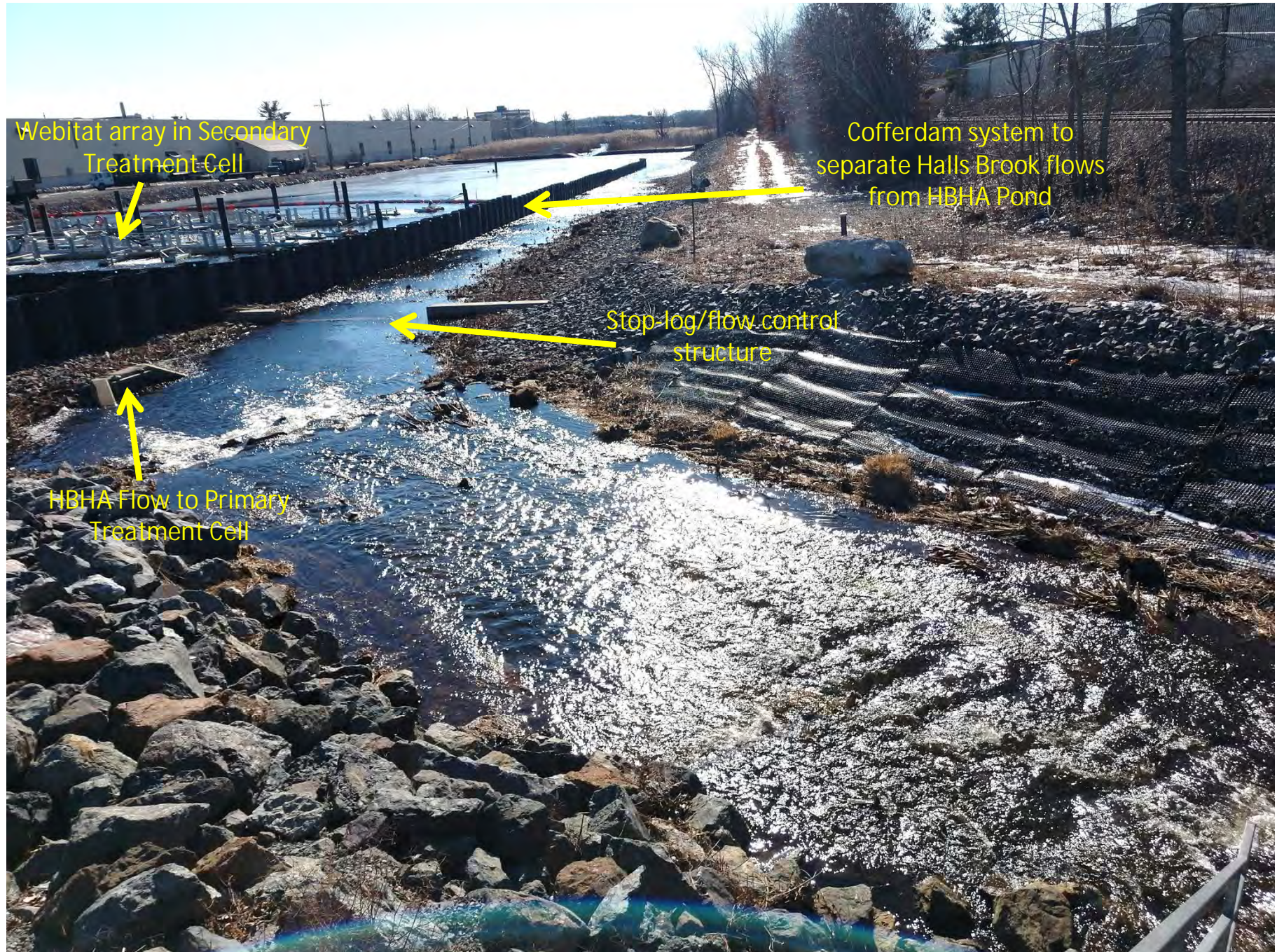
Halls Brook Storm By-Pass structure
