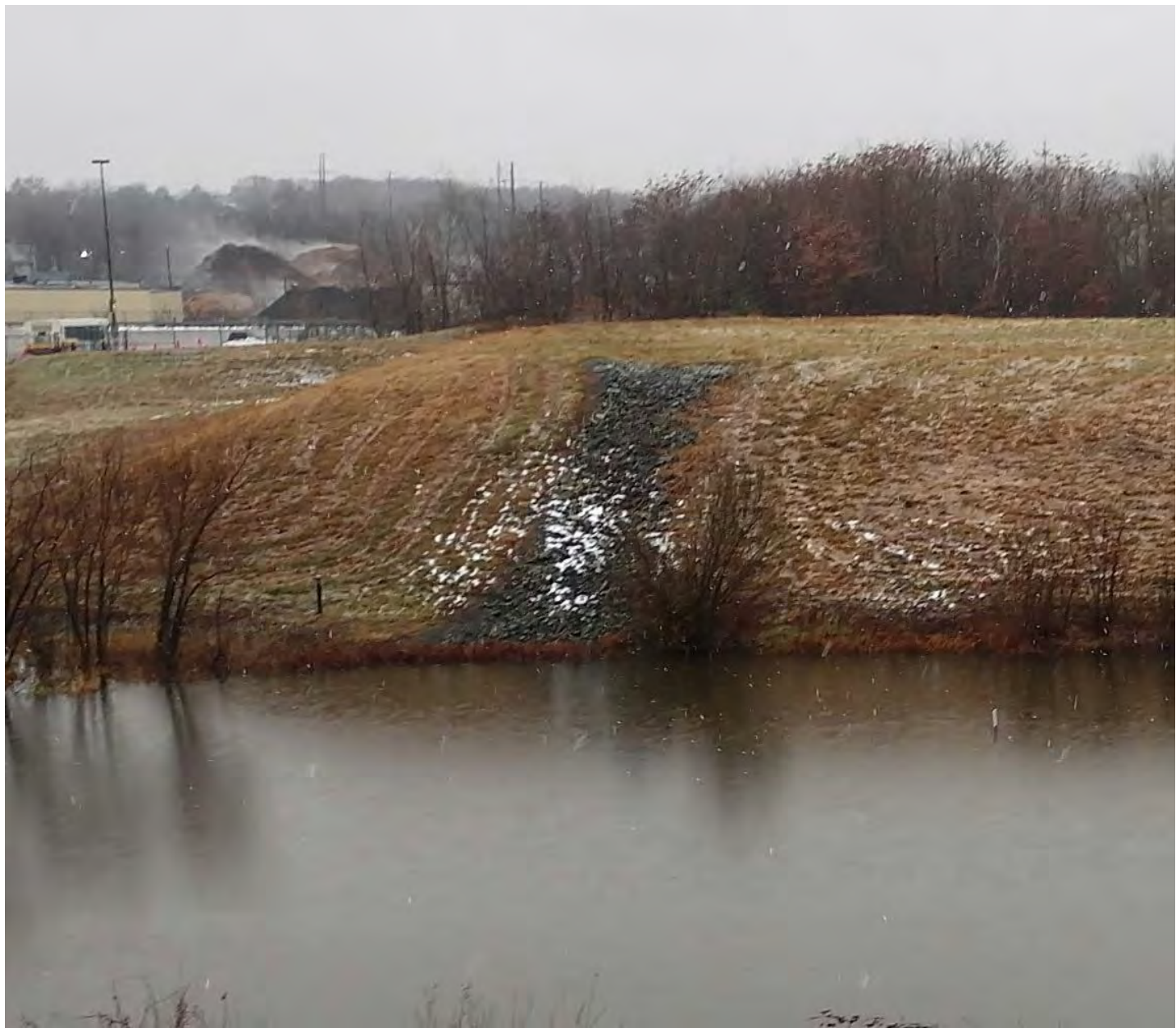
West Hide Pile armored slope drain on eastern slope.
