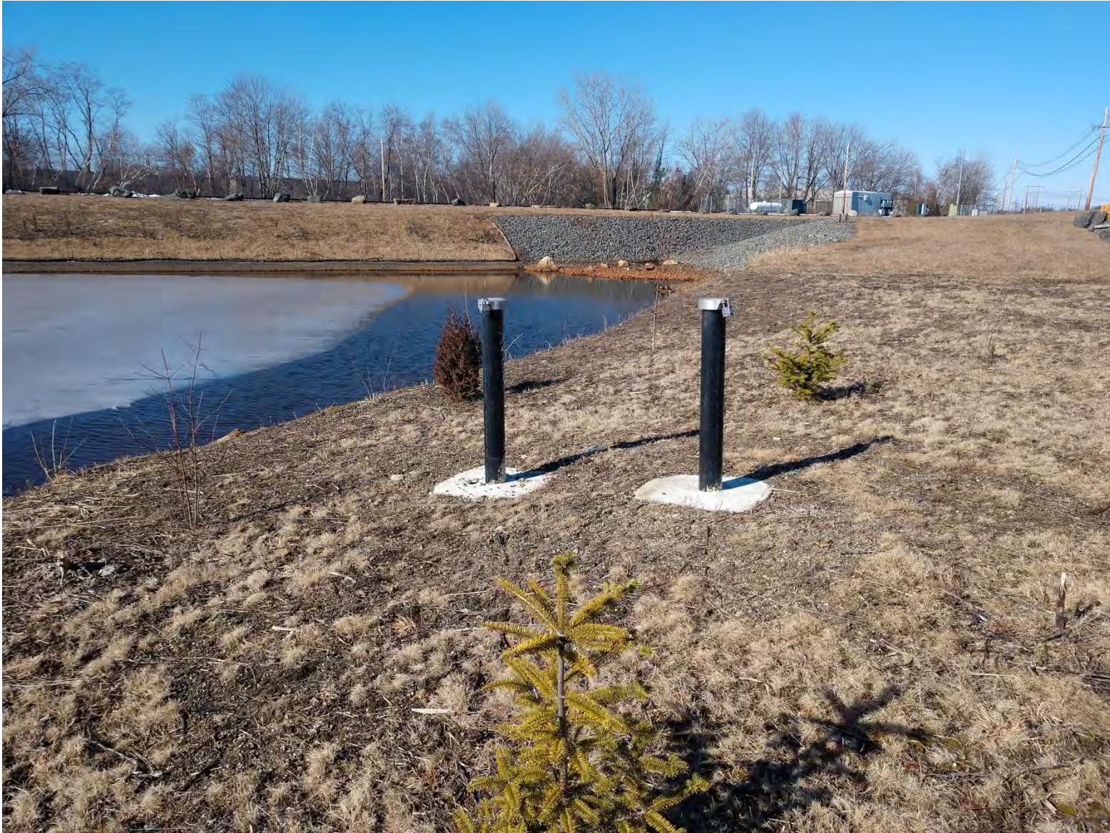
Typical Long-term Groundwater Monitoring Well Installation
