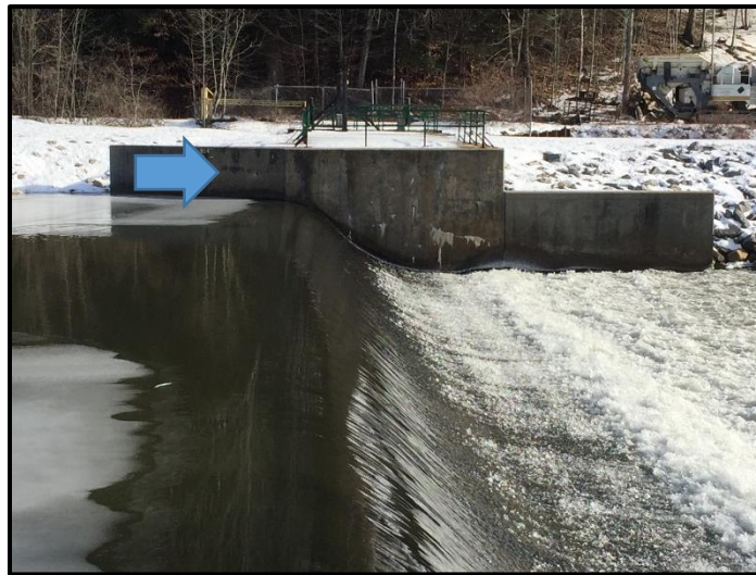
Photo 1 : Reservoir (headwater) measuring point on left training wall.
