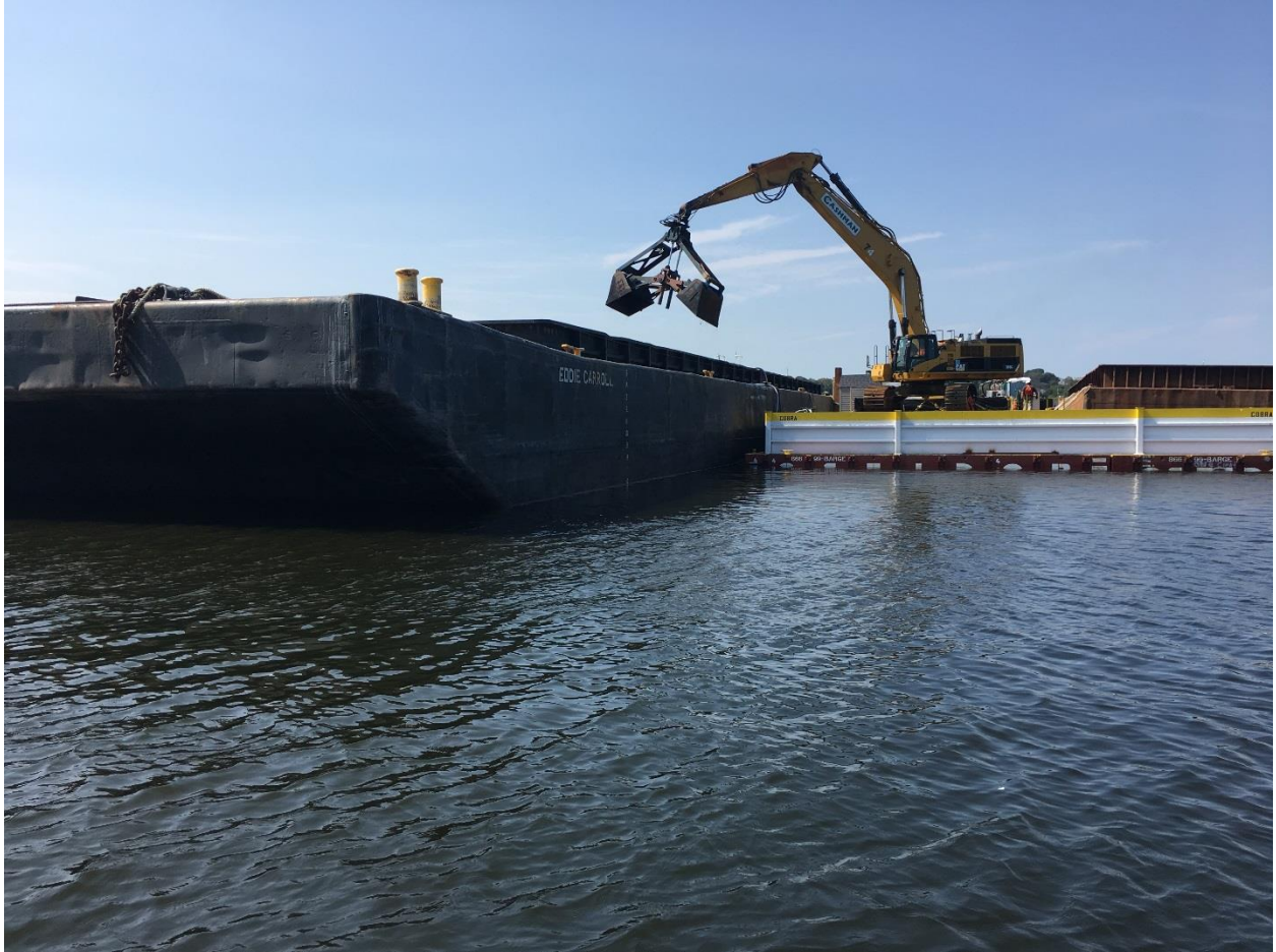
Caption for photo below: Sediment dredged from the Lower Harbor is loaded aboard a split hull scow for transport and placement in the Lower Harbor CAD Cell. September 2017
