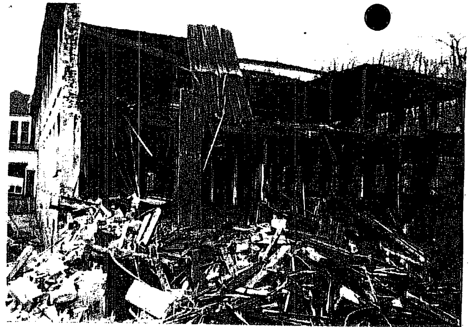
3.) Brunswick Mill building remains, looking west from debris piles
