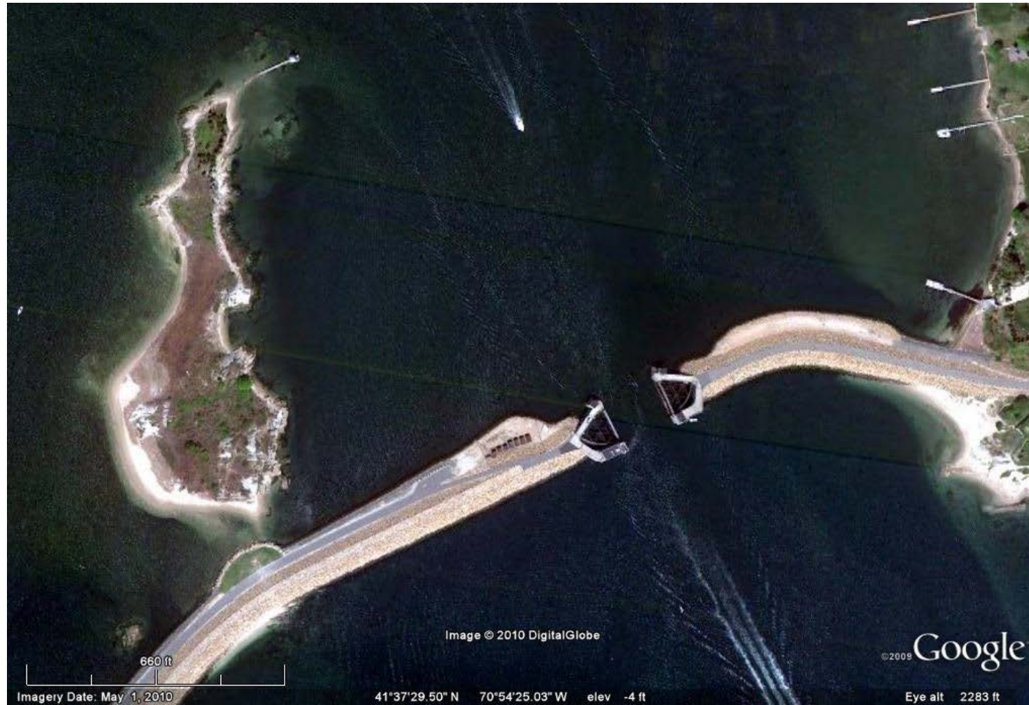
Figure 1-4. Hurricane Barrier and Entrance Channel to New Bedford Harbor.
