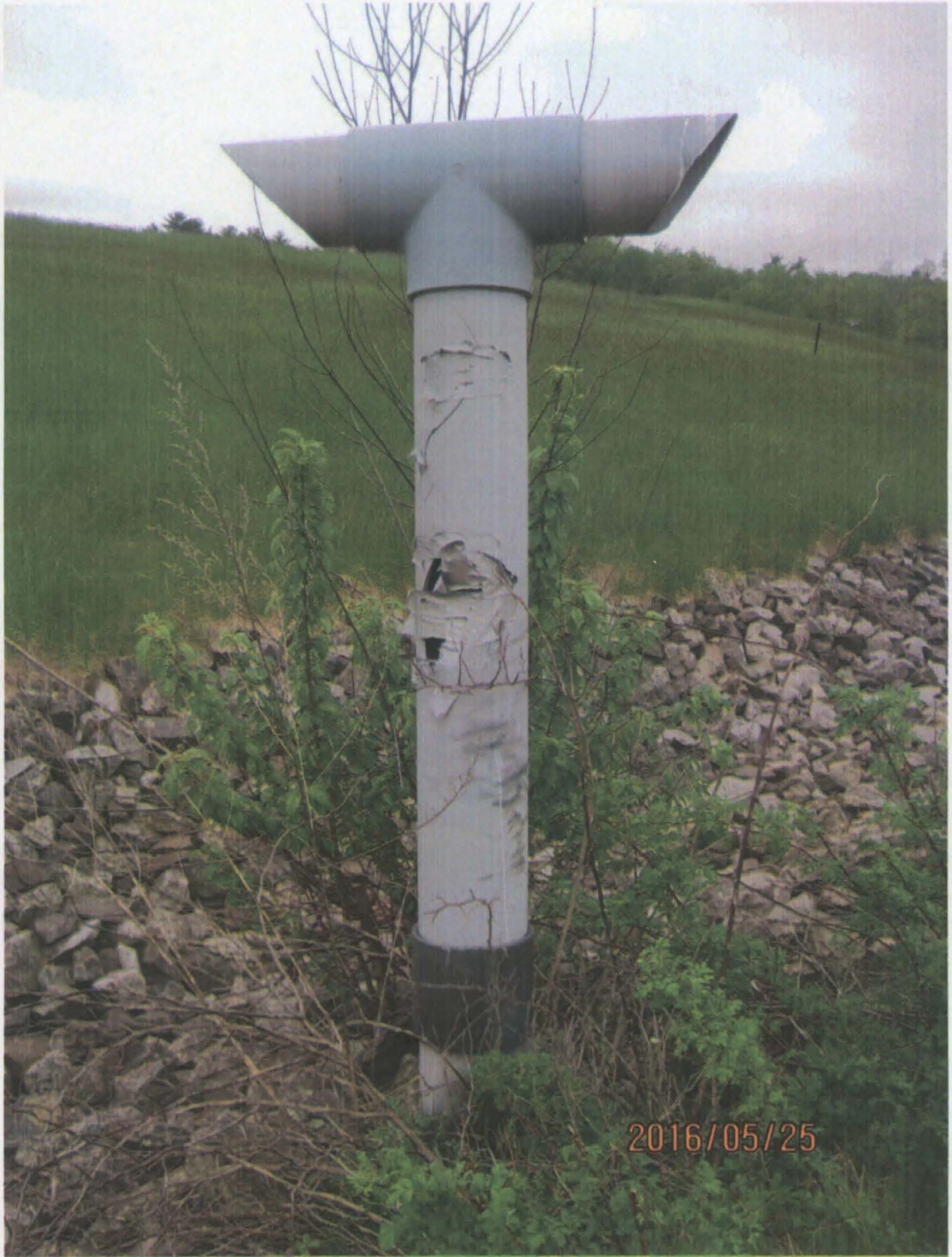
View of damaged gas vent (second vent left of the dirt road going east to west).
