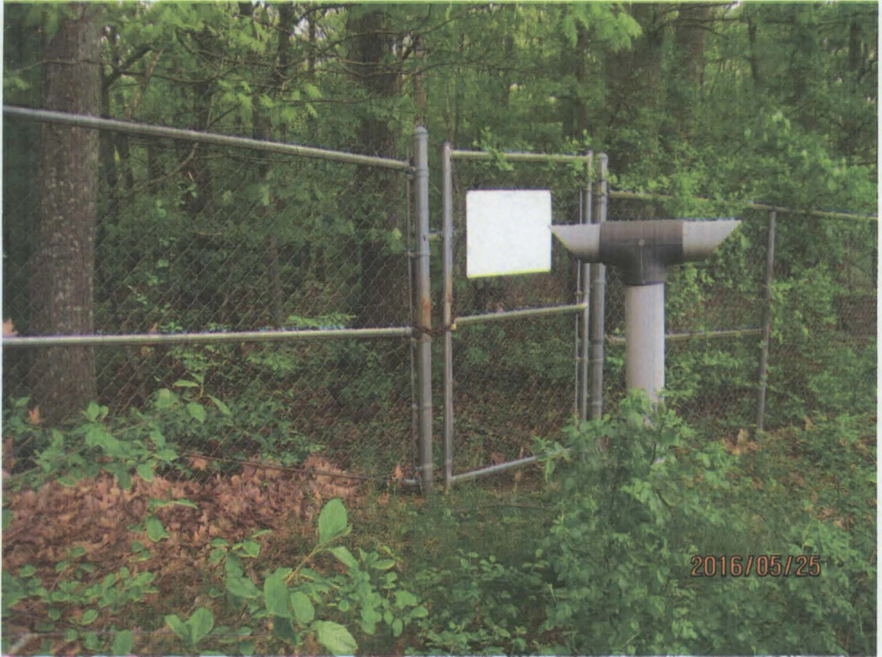
View of the gate at the southeastern corner of the fence, looking to the southwest.
