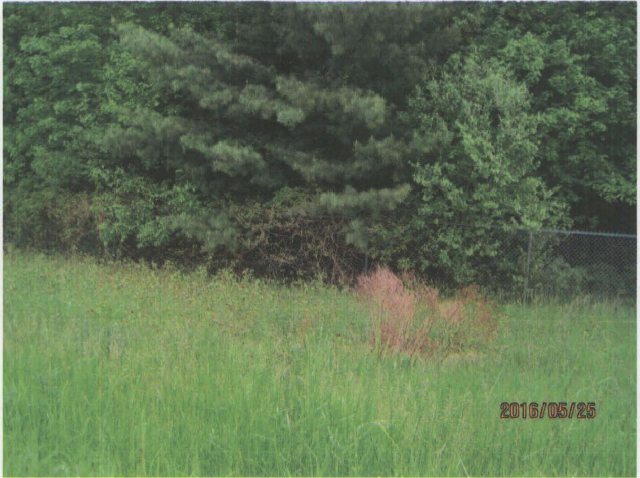
An example of vegetation that has grown too close and into the fence.
