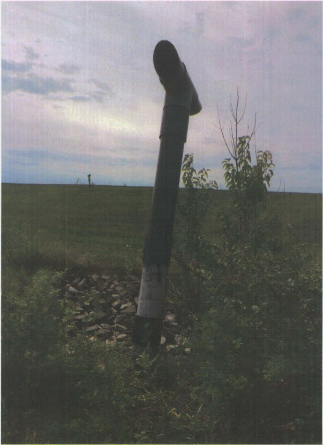
Photograph sent by the PRP in August 2016 documenting the repairs (new PVC couplings) to a broken gas vent.
