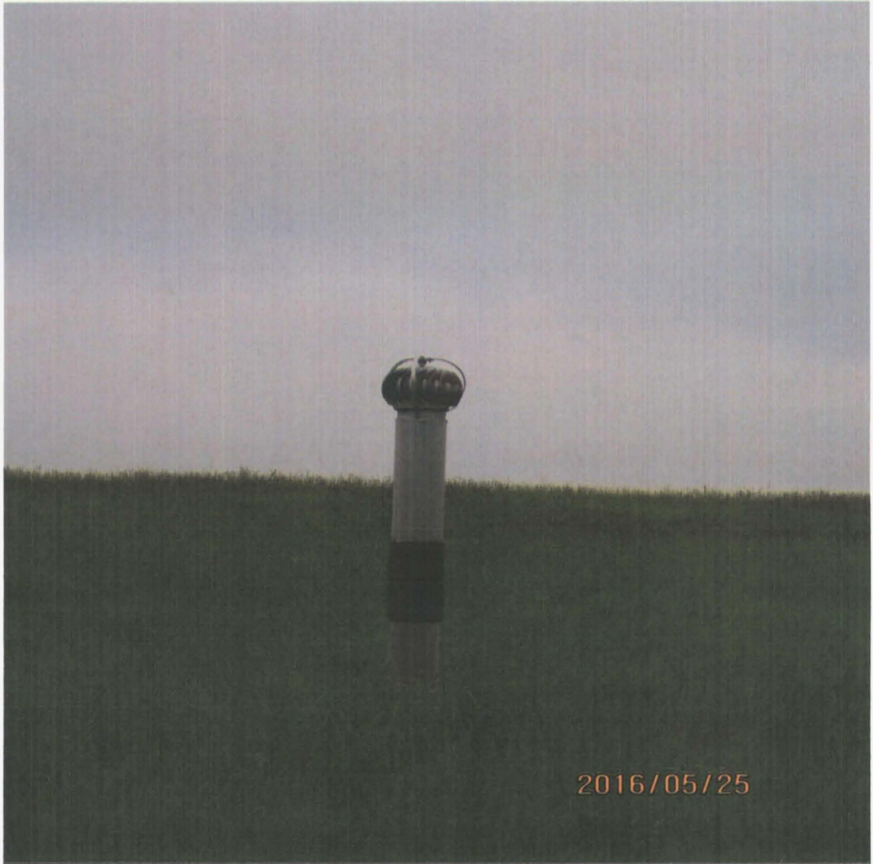
View of one of the gas vents with the whirly-wind cap not turning. Note the corrosion on the cap.
