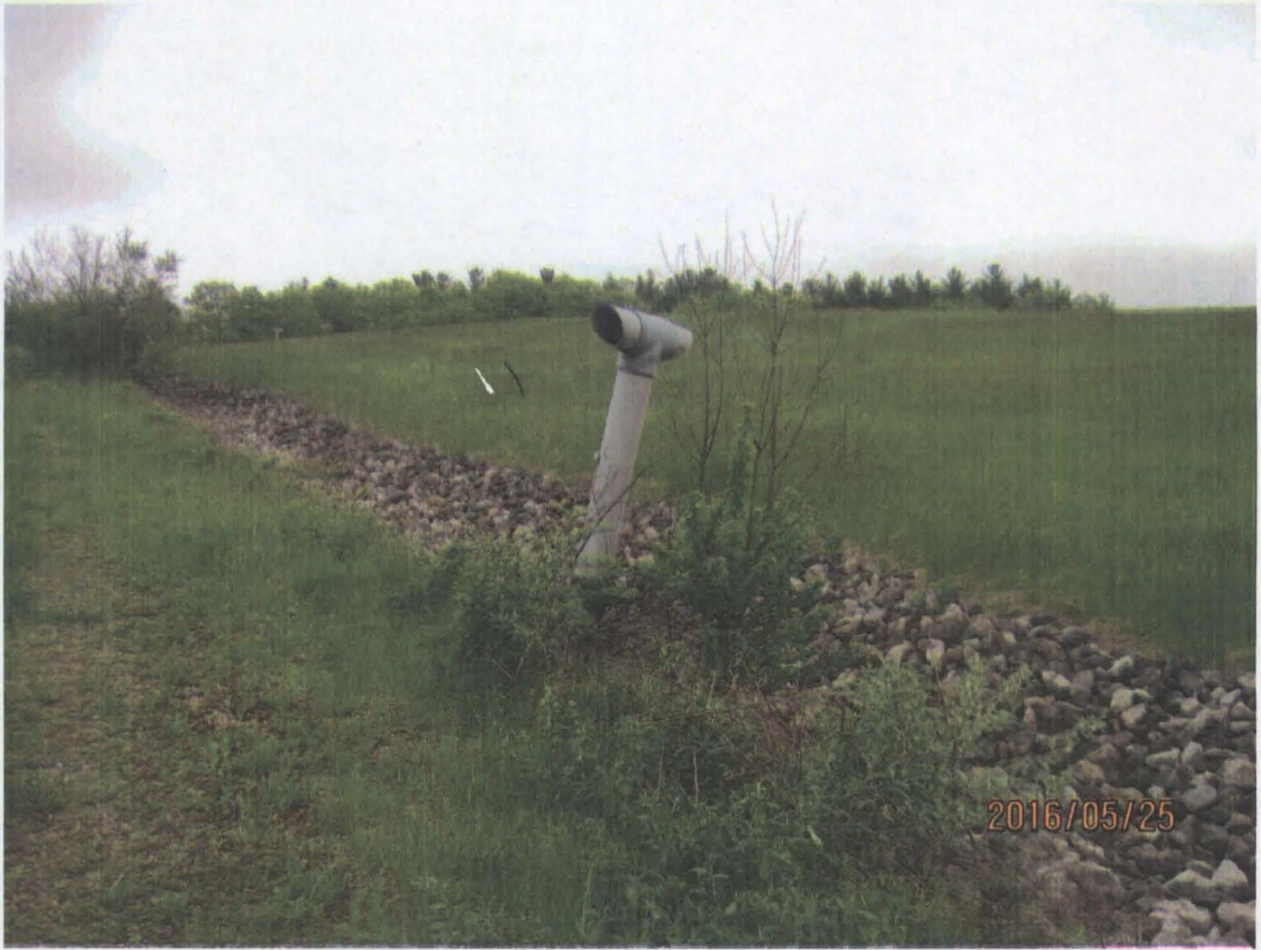
View of the damaged gas vent on previous figure looking south. Note that it is at an angle; also note overgrown vegetation within the rip-rap.
