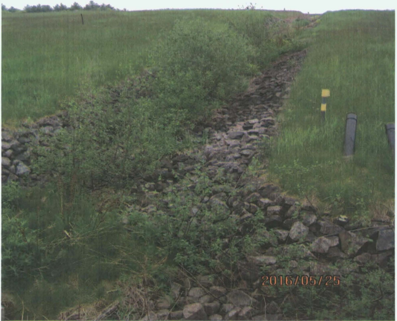
View of overgrown vegetation in one of the drainage channels, looking to the southwest.
