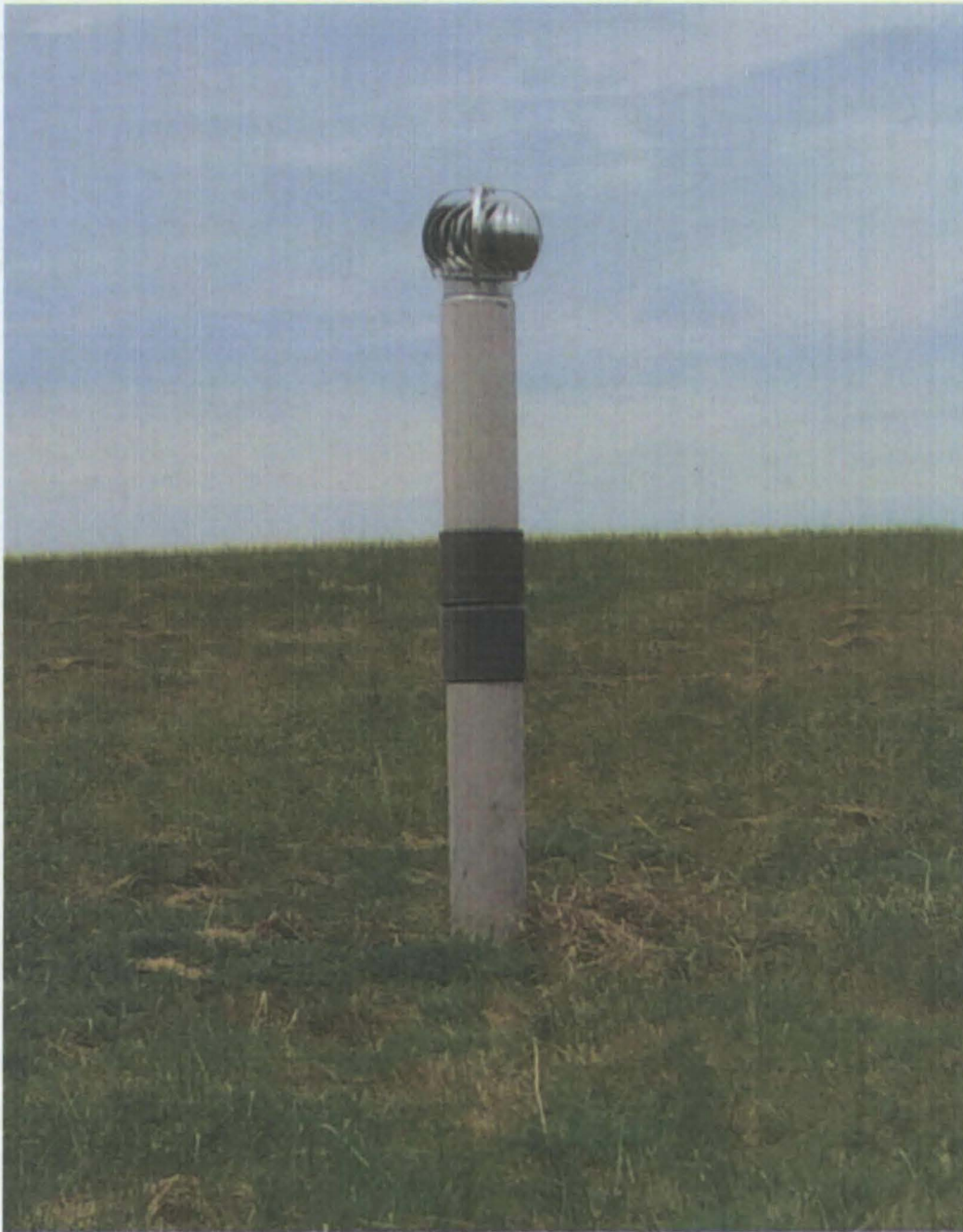
Photograph sent by the PRP in August 2016 documenting the repair (new whirly-wind cap) to a gas vent.
