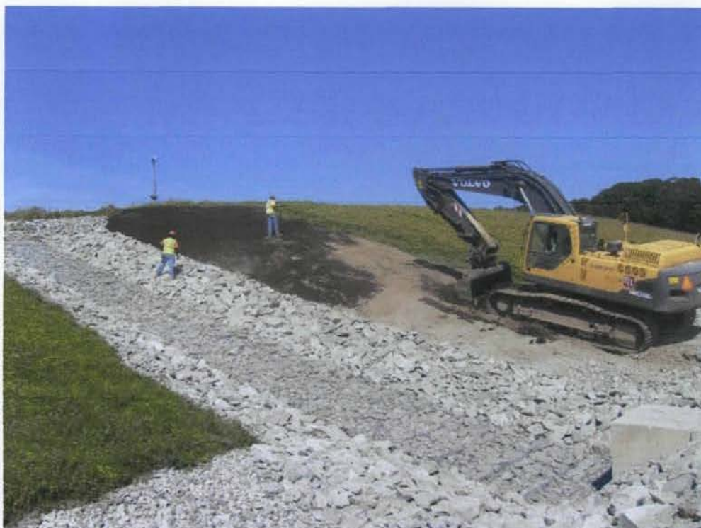
16) Placing plantable soil layer along north side of downchute. 8/28/08
