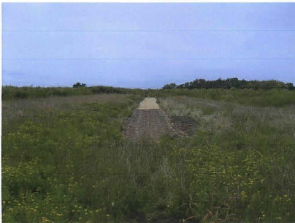
20) Repaired rill covered with erosion control blanket, top of landfill. 8/28/08
