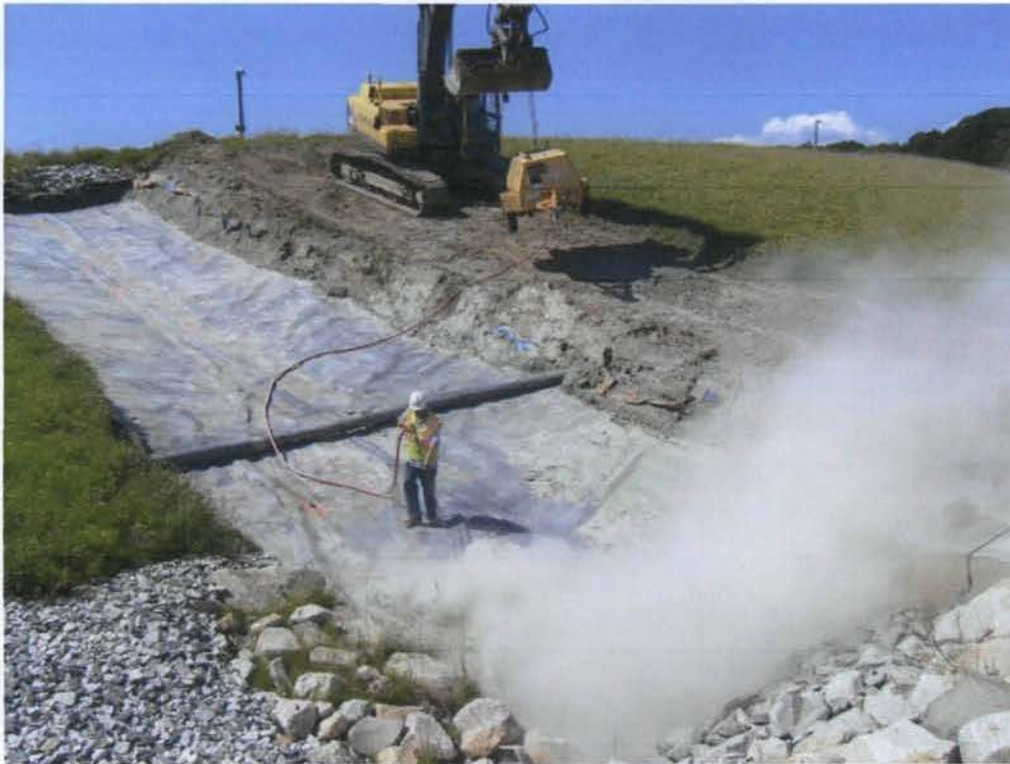
5) Air compressor cleaning of VSL soil from landfill liner. 8/22/08
