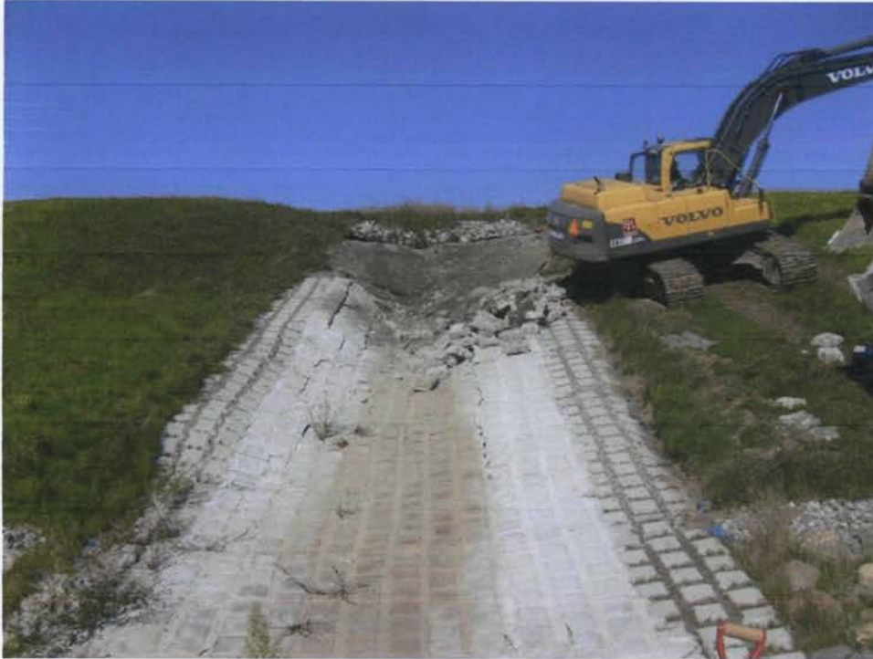
1) Start of articulating concrete block removal in downchute. 8/21/08
