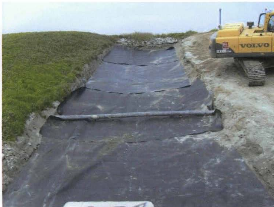
8) Placement of top sacrificial liner in downchute, shingle style. 8/25/08
