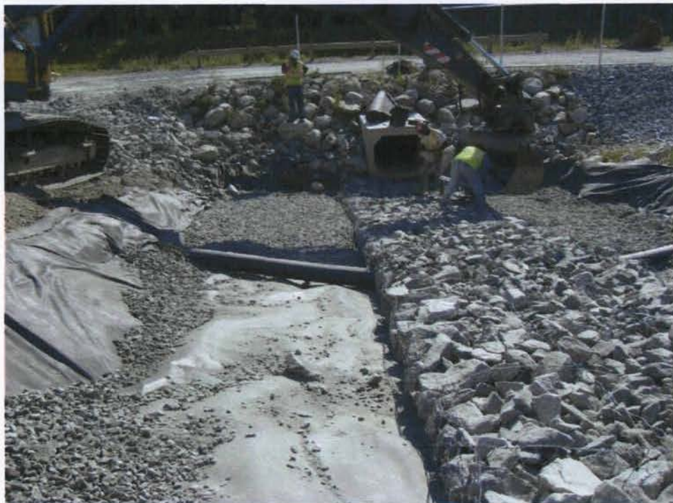
9) Gabion basket construction continued. 8/26/08
