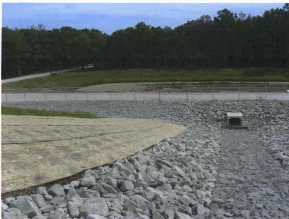
19) Side slope seeded and protected with erosion control blanket. 8/28/08
