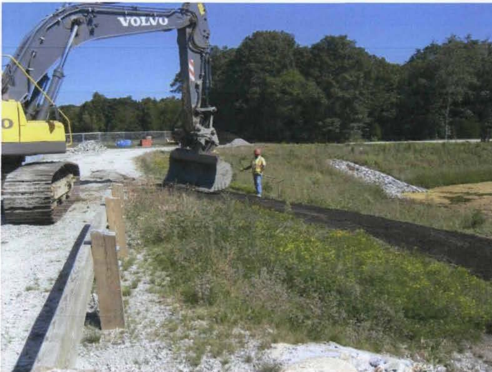
15) Repairing excavator tracks from cleaning out forebay in South Pond. 8/28/08
