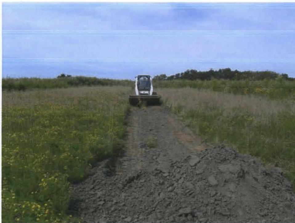
18) Repairing rill in center swale, top of landfill. 8/28/08
