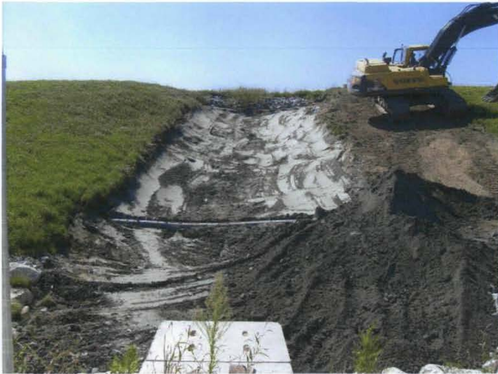
3) Removal of VSL soil layer under articulating concrete block. 8/21/08
