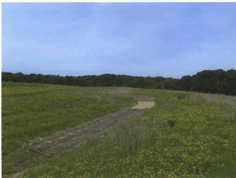
21) Repaired rill covered with erosion control blanket, top of landfill. 8/28/08
