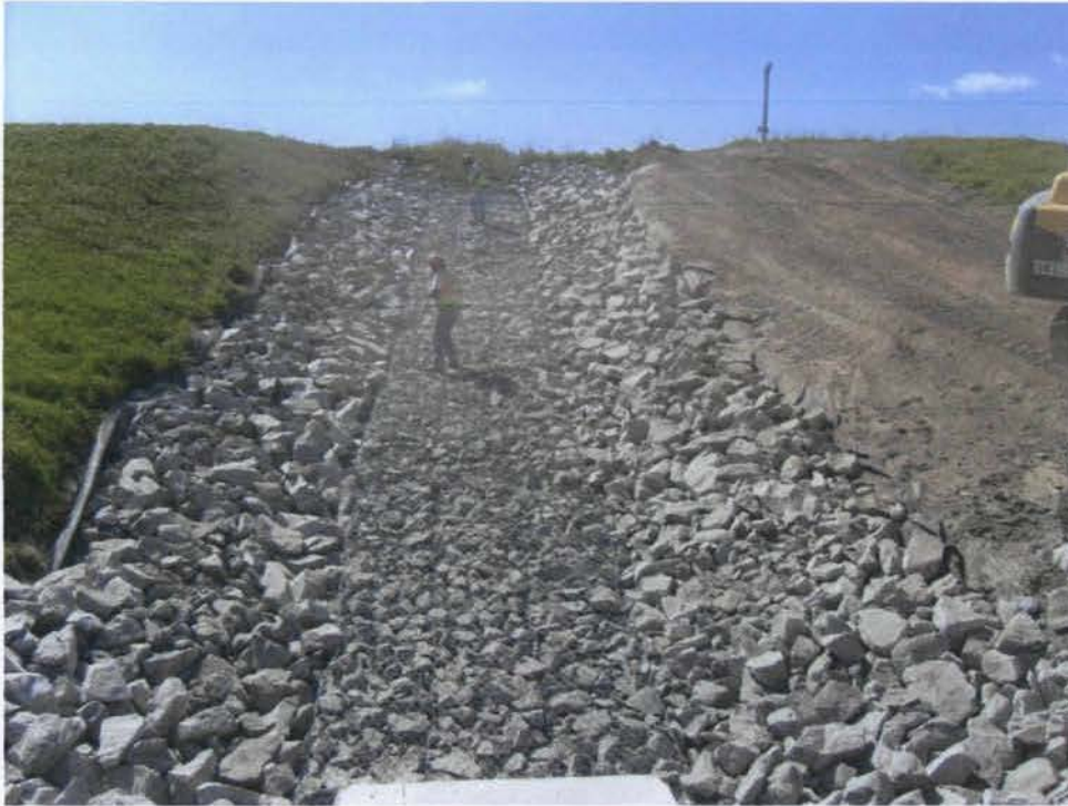
12) Placement of R-5 riprap in downchute complete, top of baskets attached. 8/26/08
