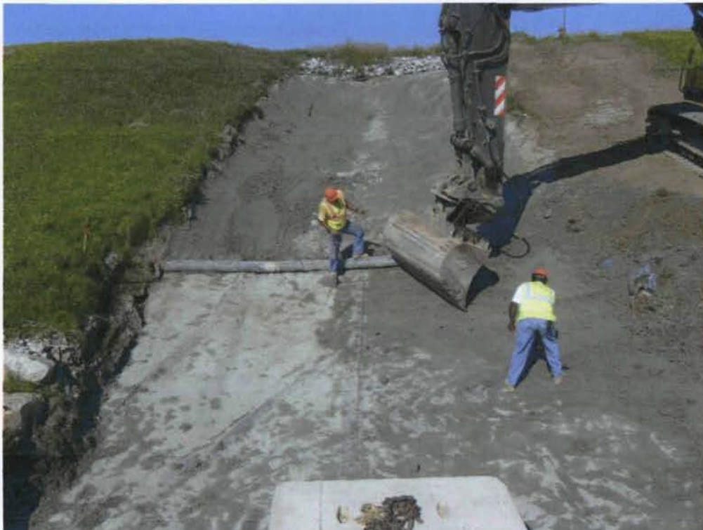
4) Removal of VSL soil layer under articulating concrete block. 8/21/08
