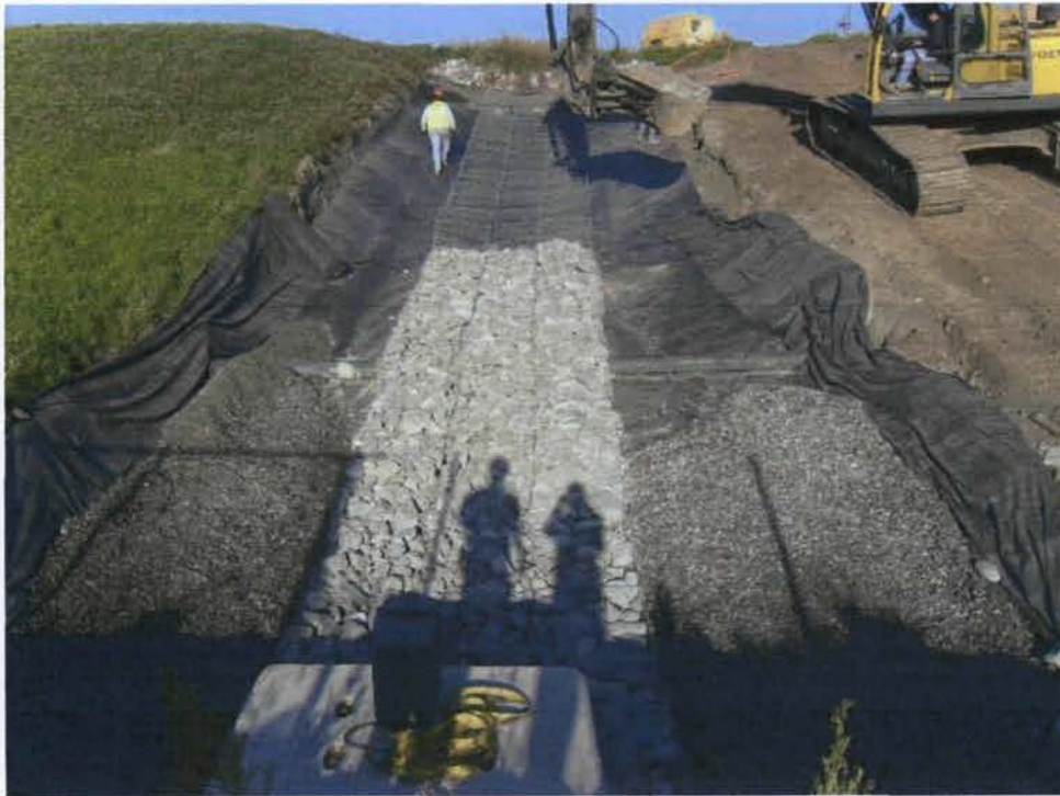
9) Placement of gabion baskets in center, 1-1/2" stone on sides of downchute. 8/26/08
