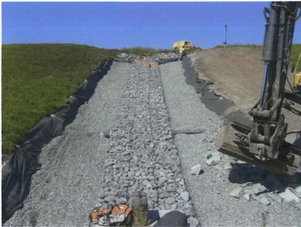
11) Placement of R-5 riprap on sides of downchute. 8/26/08
