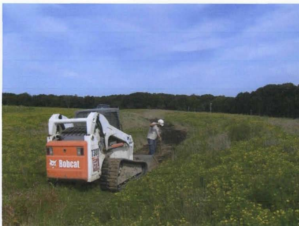
17) Repairing rill in northeast swale, top of landfill. 8/28/08
