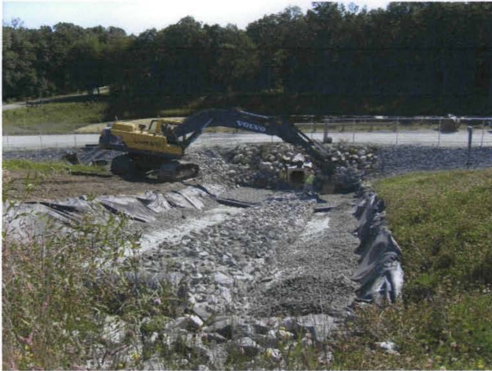
10) Gabion basket construction continued. 8/26/08
