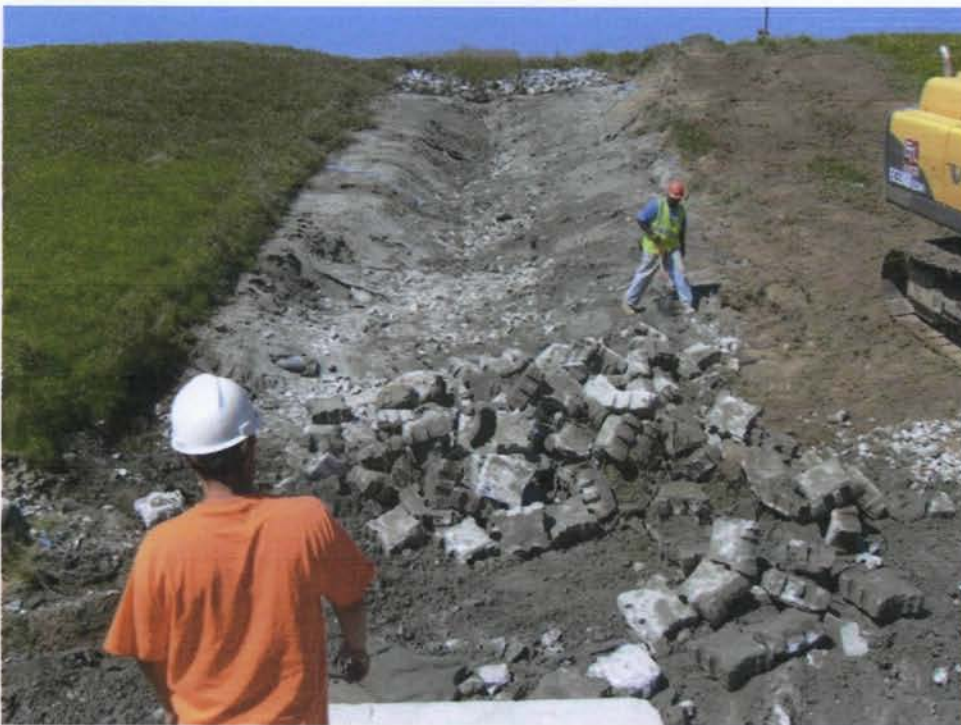
2) Continued removal of articulating concrete block in downchute. 8/21/08
