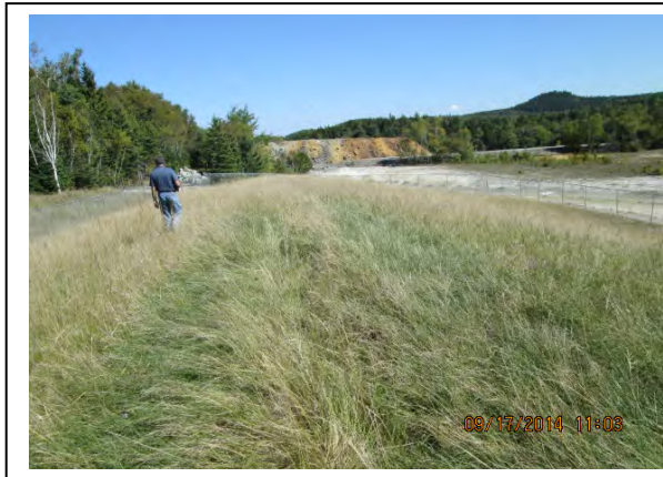
Grass growth on top of PCB storage area
