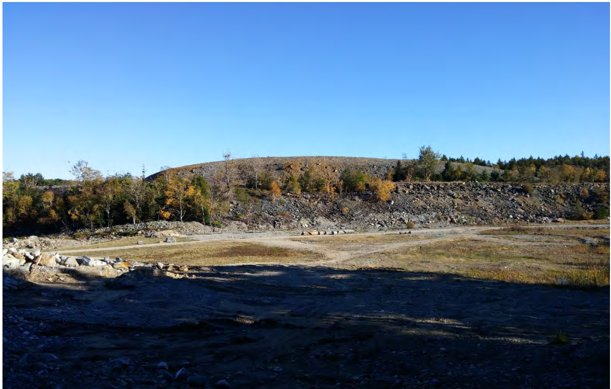
Photo 3 - Mine Operations Area looking S
