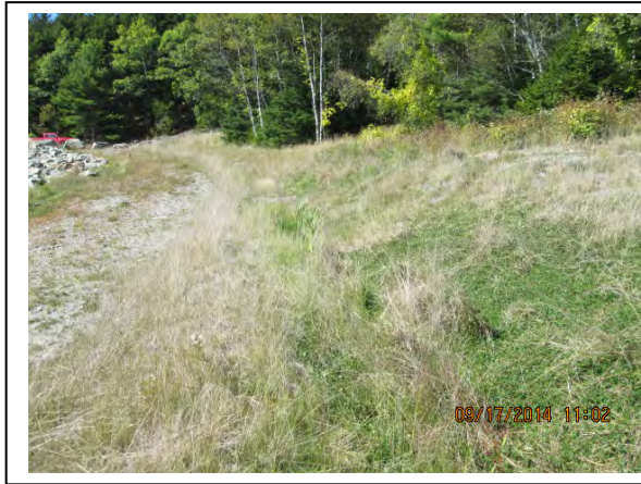
Drainage swale along tailings access road
