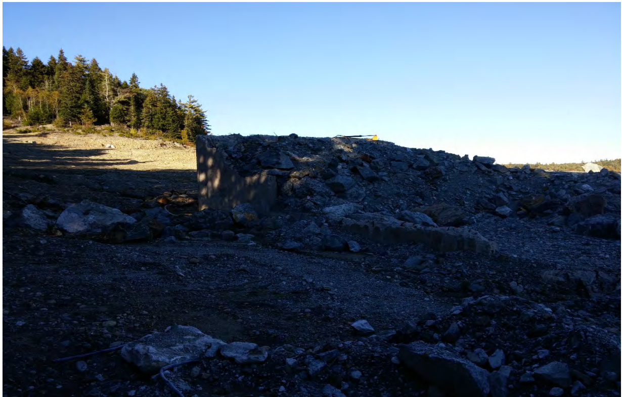
Photo 5 - Ore Pad Building Foundation looking NE
