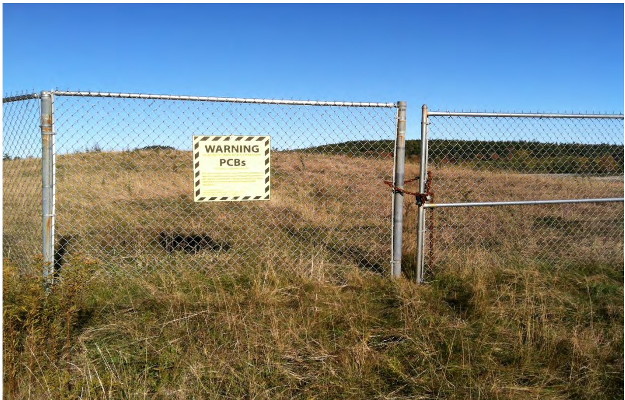
Photo 8 - PCB Cap Sign
