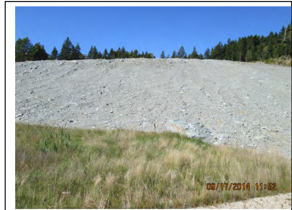
Sideslope of Waste Rock Pile #2
