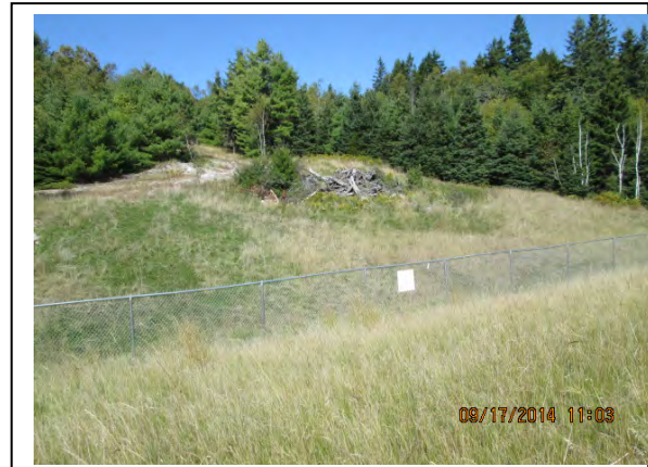
Western backslope adjacent to PCB storage area
