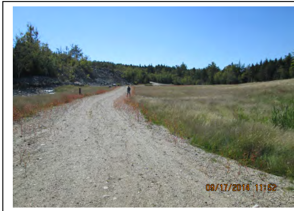
Access road surface dividing Zones 3 & 4
