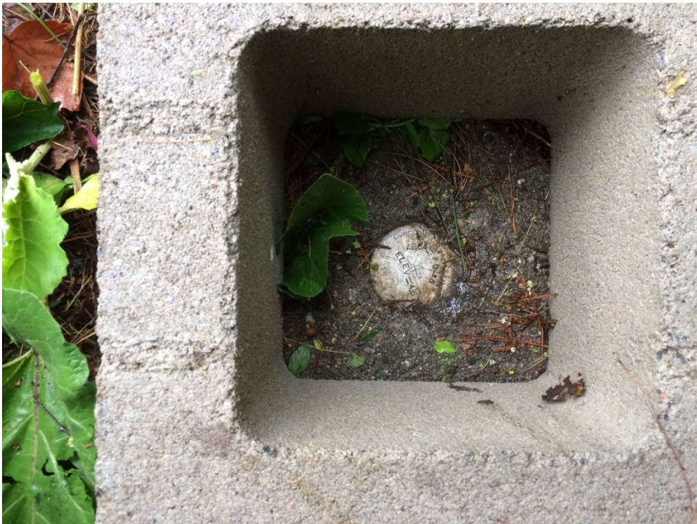
Photo 5: Placement of AUL Marker at CRPP Open Area
