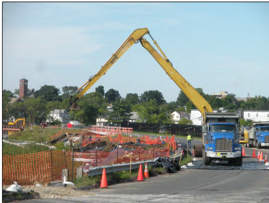
Photograph 6: Soil removal activities (Polygon 5) (8/20/12)
