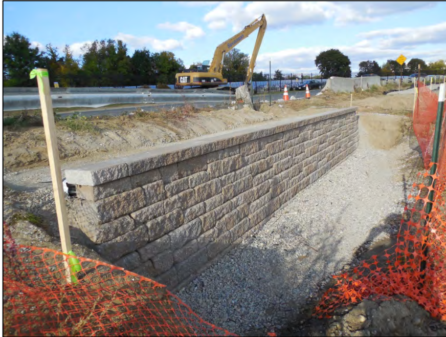
Photograph 55: Installation of retaining wall along walking path (9/26/13)
