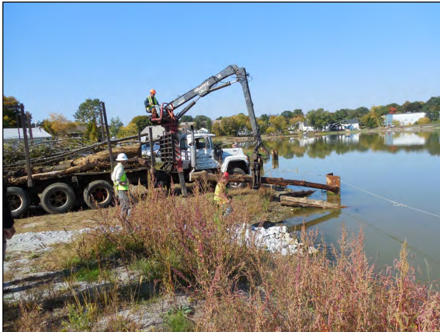
Photograph 56: Installation of large woody debris (10/1/13)
