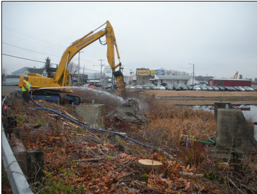
Photograph 20: Removal of debris (Target 14) (12/4/12)
