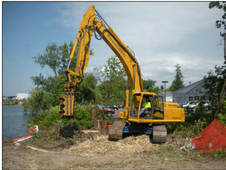
Photograph 2: Installation of sheetpile weir/stop log structure Housatonic River Outfall (7/18/12)
