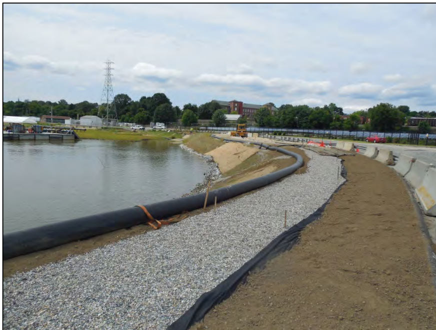
Photograph 52: Walking path subgrade preparation (7/25/13)
