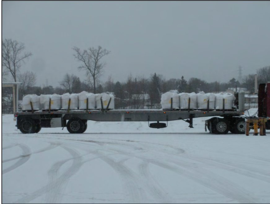
Photograph 31: Delivery of super sacks of Lime Kiln Dust to Bldg.65 (2/27/13)
