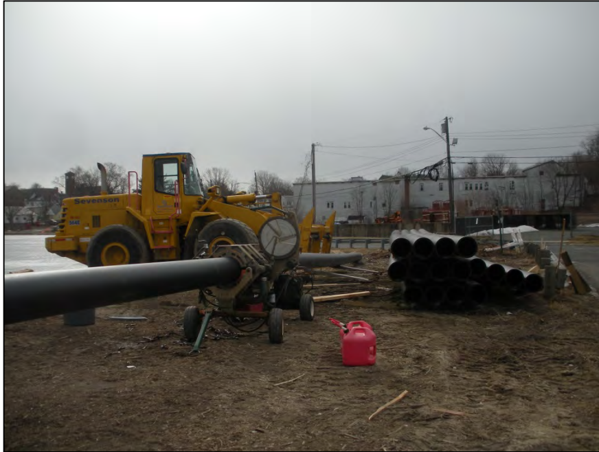
Photograph 35: Fusing of HDPE Pipe in preparation for hydraulic capping activities (3/14/13)
