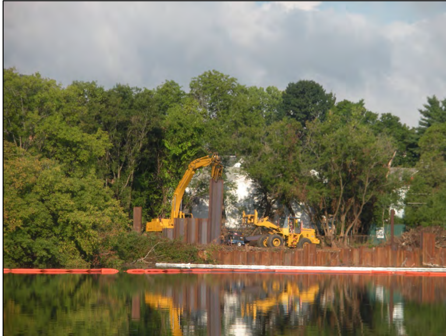
Photograph 5: Installation of sheetpile for soil removal activities (8/16/12)
