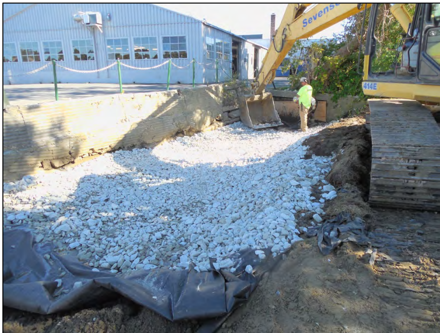
Photograph 54: Installation of geotextile fabric and armor stone in channel (9/19/13)
