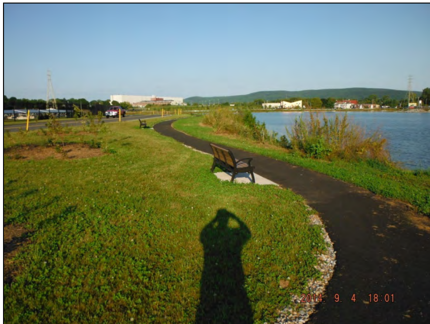
Photograph 72: Walking path and bank vegetation in northwest portion of lake (9/4/14)
