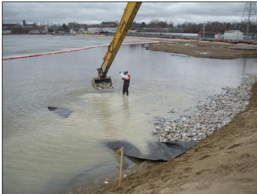
Photograph 40: Installation of armor stone layer in near-shore area (3/28/13)
