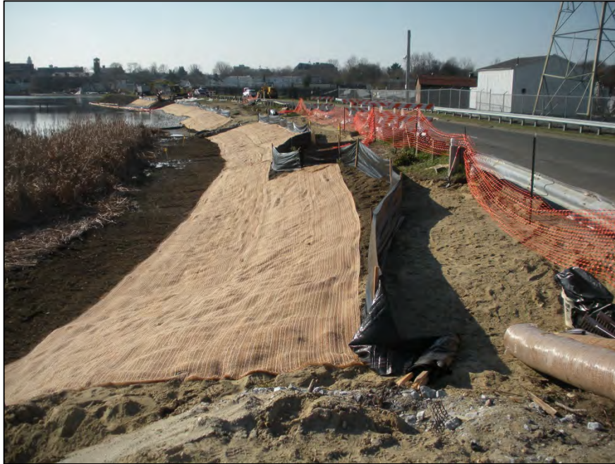
Photograph 15: Installed erosion control blanket in restored Recreational Areas (11/10/12)
