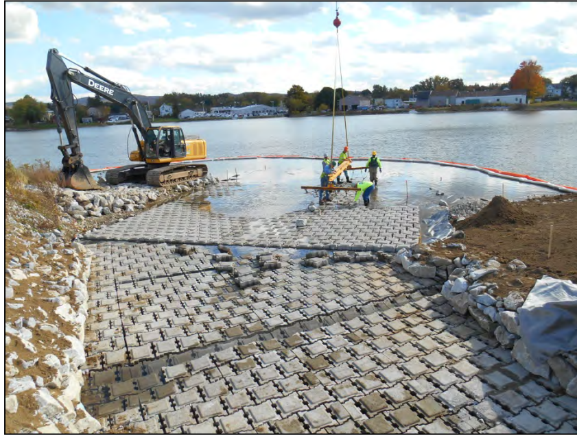
Photograph 77: Restoration of Fourth Street Outfall Channel (10/9/14)
