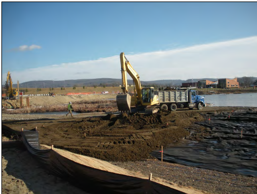
Photograph 24: Installation of cap and topsoil material on Shrub-Scrub Island (12/12/12)
