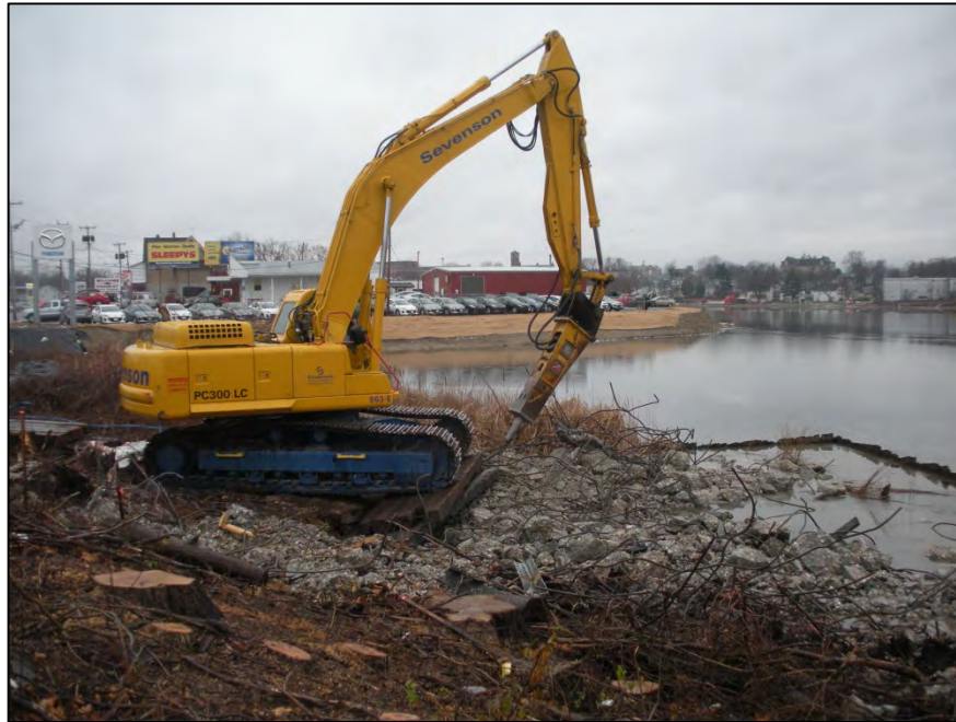
Photograph 21: Removal of debris (Target 14) (12/7/12)
