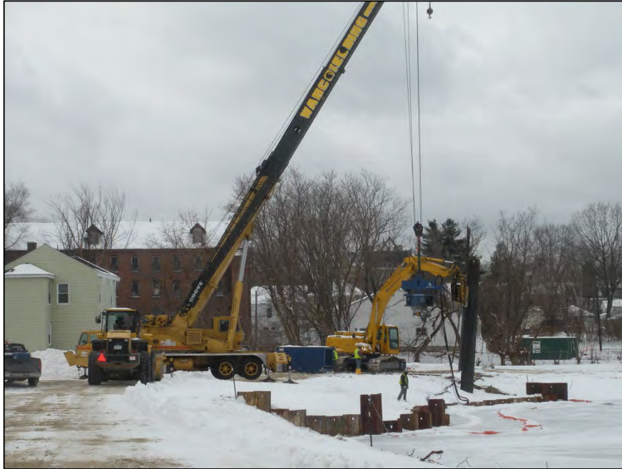
Photograph 25: Removal of sheetpile (1/2/13)
