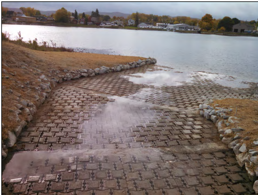
Photograph 78: Restored Fourth Street Outfall Channel (10/15/14)
