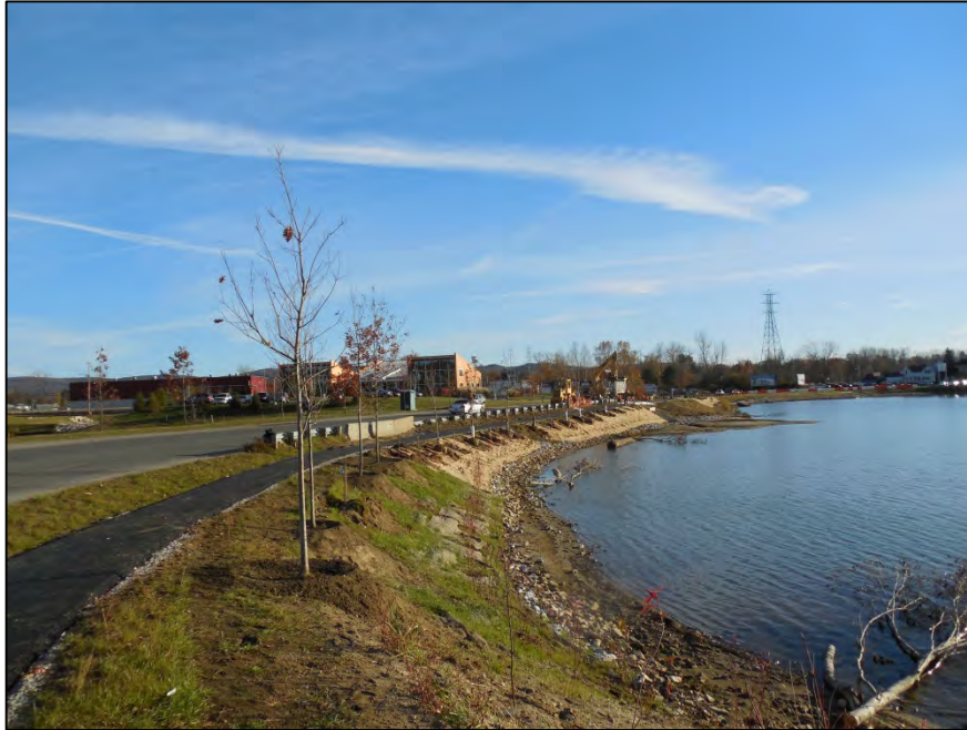
Photograph 63: Installed plantings along the walking path (11/4/13)
