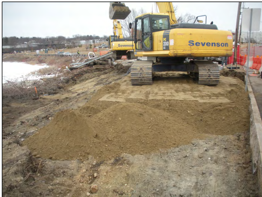
Photograph 36: Backfill activities (Polygon 9B) (3/18/13)
