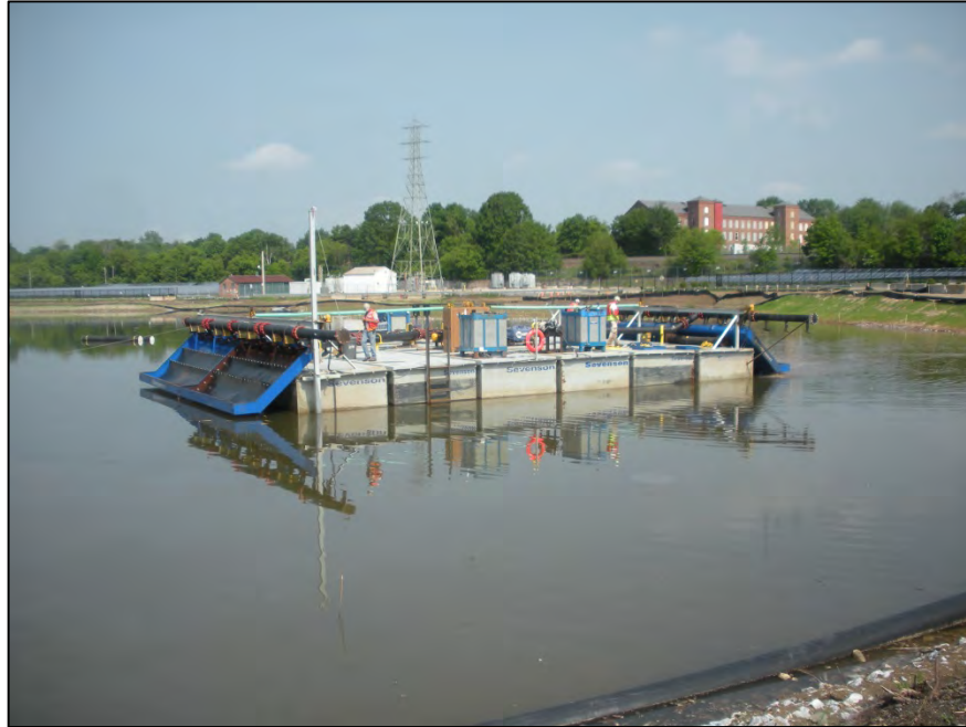
Photograph 47: Hydraulic capping activities (5/30/13)
