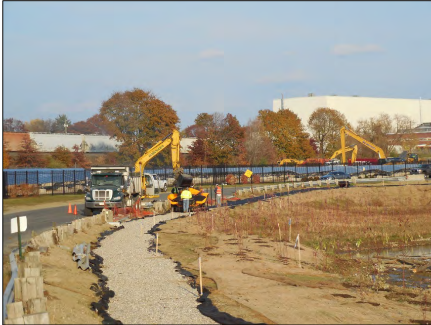
Photograph 59: Paving of the walking path (10/30/13)
