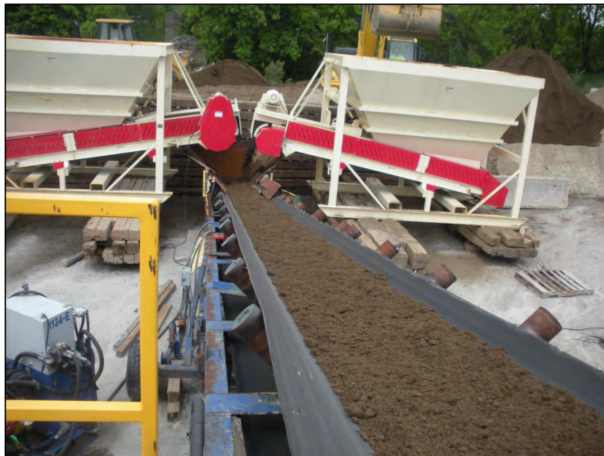
Photograph 48: Cap material on conveyor belt to hopper (5/30/13)
