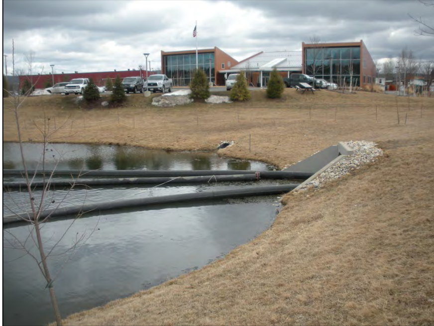
Photograph 41: HDPE pipe installed through PEDAs Outfall in preparation for hydraulic capping activities (3/28/13)
