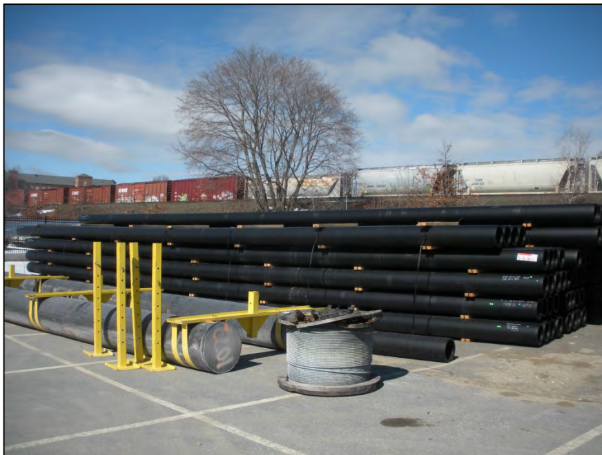
Photograph 32: Staged HDPE pipe for hydraulic capping activities (3/5/13)
