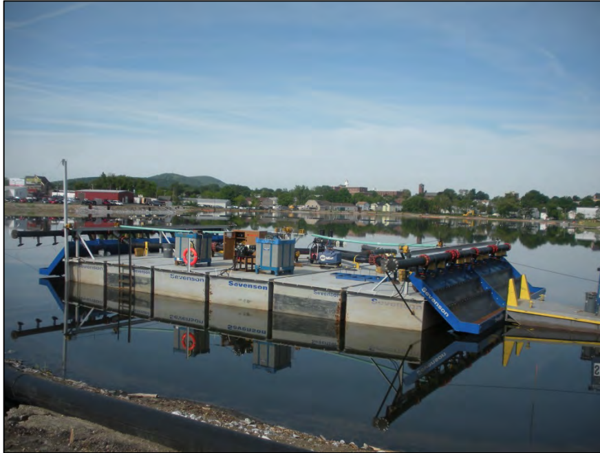
Photograph 45: Hydraulic capping barge fully assembled (5/28/13)
