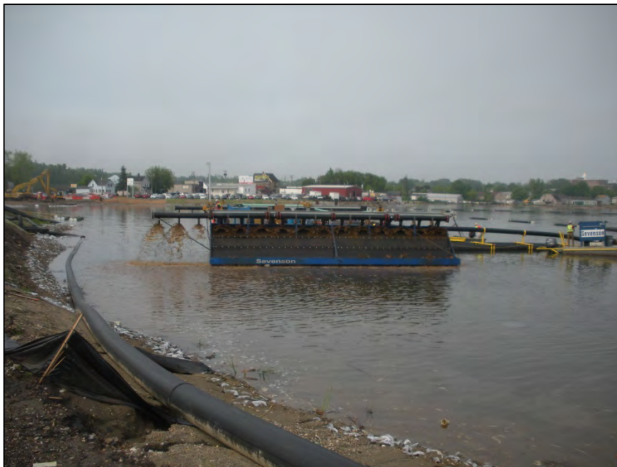
Photograph 46: Hydraulic capping activities (5/30/13)
