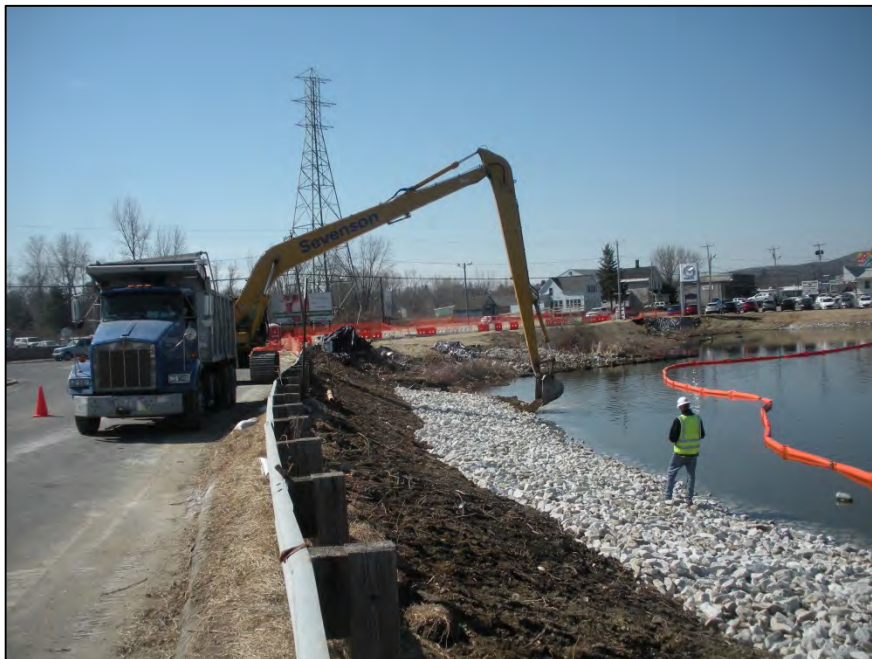
Photograph 42: Installation of near-shore area Gravel Habitat Layer (4/5/13)
