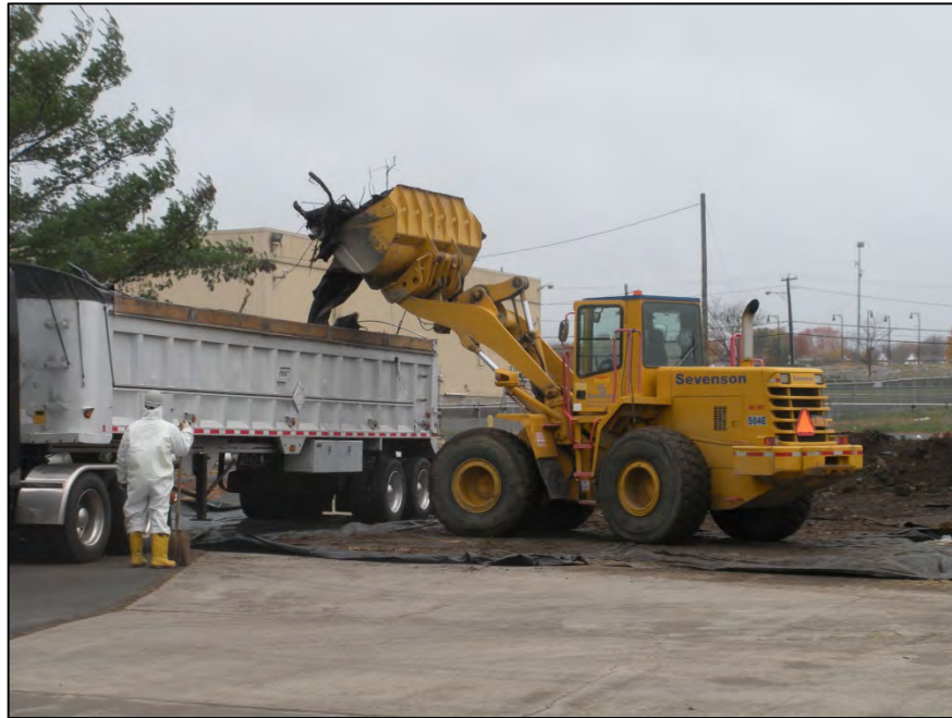
Photograph 13: Soil/debris material handling at temporary stockpile (10/31/12)
