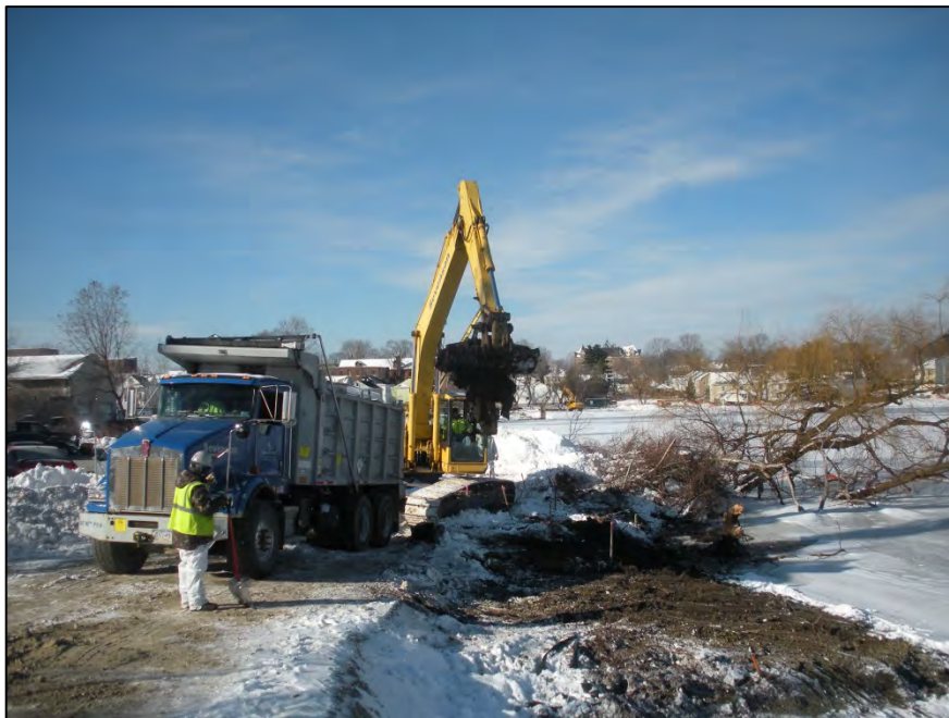
Photograph 26: Direct loading of cleared and grubbed vegetation (1/3/13)
