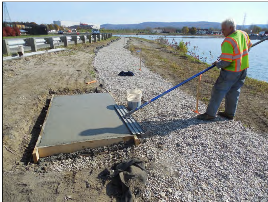
Photograph 58: Construction of pad for benches along walking path (10/21/13)
