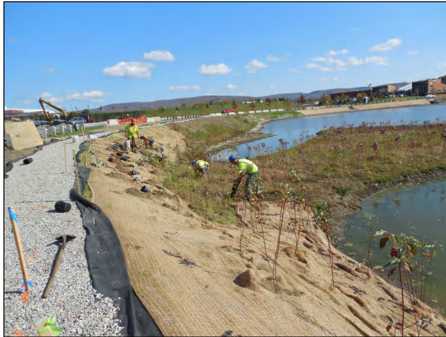
Photograph 57: Installation of plantings on Shrub-Scrub Island (10/17/13)
