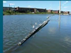
Floating and submerged pipelines
