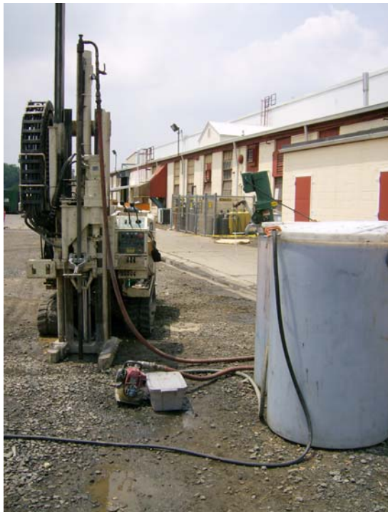
Figure 2 - Direct Injection of Iron NPs in the Field at the Trenton Facility, New Jersey (Photo courtesy of Geosyntec Consultants)
