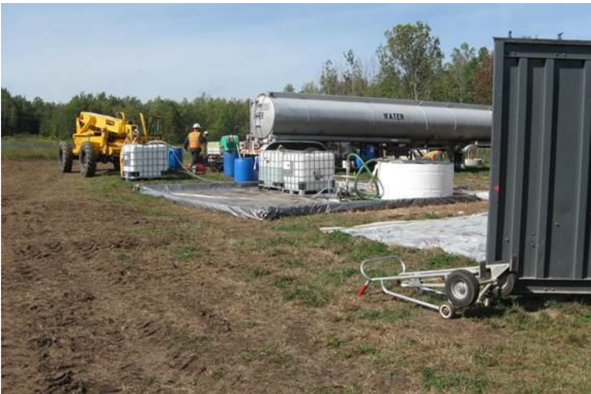
View of Oxidant Staging Area During ISCO Injections, Fall 2010
