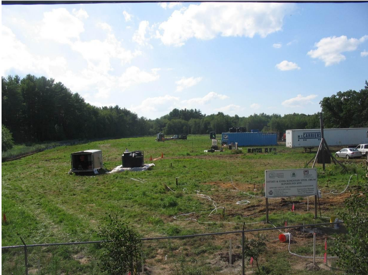
View from Route 125 During ISCO Injections, Fall 2008
