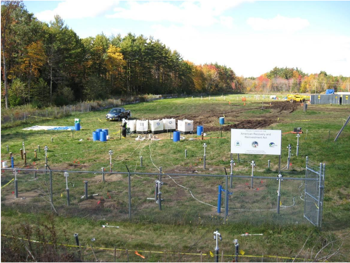
View from Route 125 During ISCO Injections, Fall 2009
