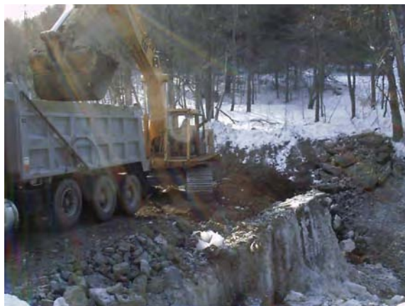
Silk Mill Dam during removal, February 2003. Fill was brought in for access road. Excavator is removing dam and sediment. Water was diverted through the culvert under the road (not in photo). Demolition and excavation took approximately 2 weeks.
