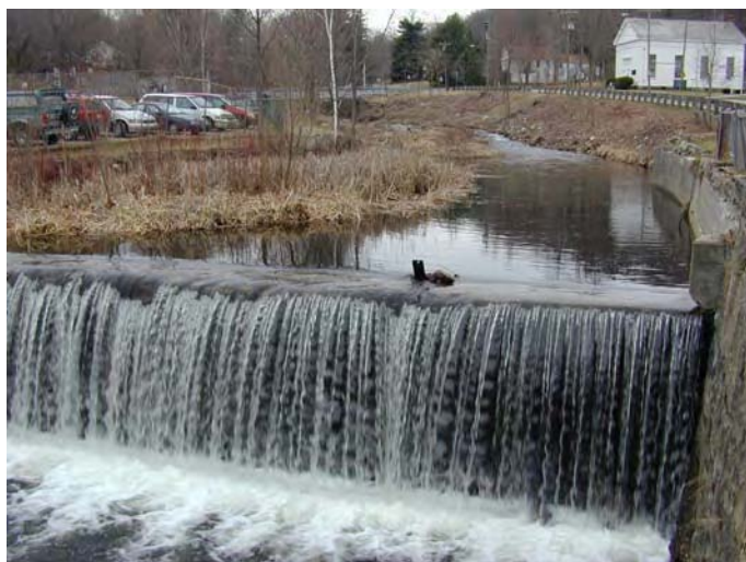
Final designs for the breaching of Ballou Dam are being discussed. The town uses this as an emergency fire water source and the design will incorporate a dry hydrant and storage tank.
