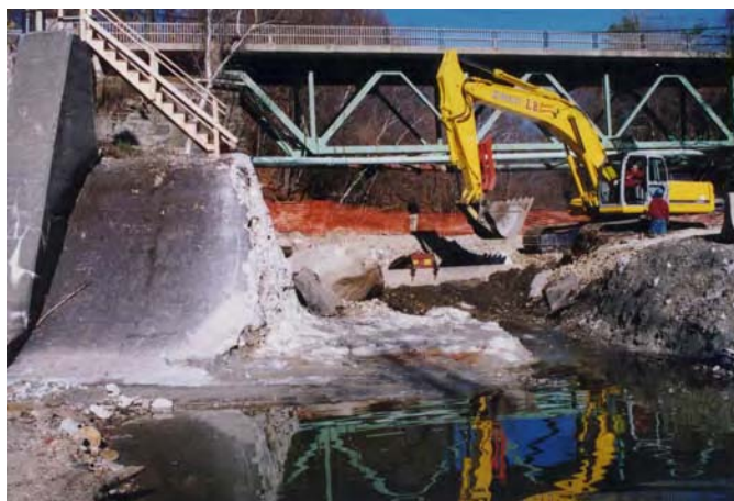
Deconstruction of Old Berkshire Mill Dam in November 2000. Photo is looking upstream at the dam.
