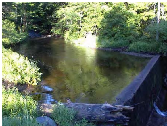
Silk Mill Dam and impoundment, June 2002. No water flowing over the dam, but back towards newly opened culvert (out of view in the lower left of photo). Note the depositional island on the river right and the sediment which almost fills the impoundment.
