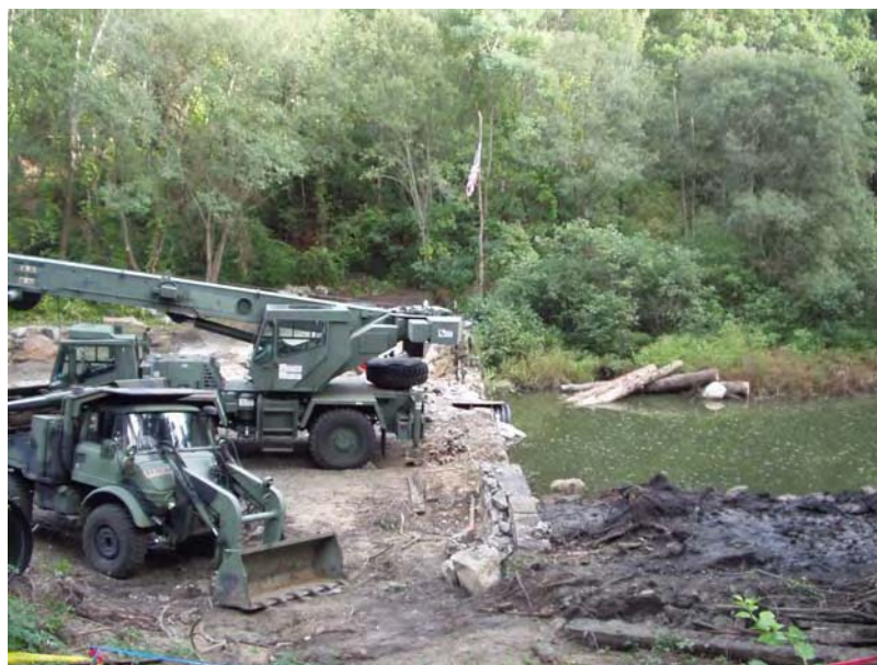
U.S. Army Reserves prepare to excavate and remove the earthen dam and sediment in the impoundment. Town Brook flows to the left through culvert under earthen dam.
