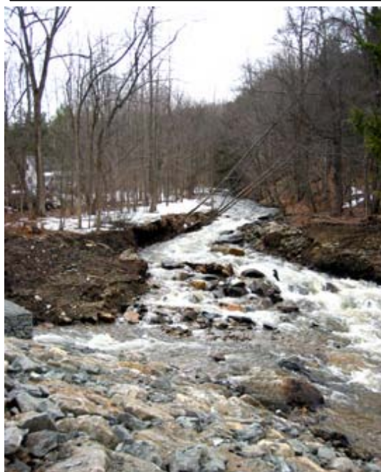
Yokum Brook after removal of Silk Mill Dam, February 2003. Note that as the newly restored stream channel adjusts to the proper channel proportions some more sediment from the depositional island will be eroded. The amount of sediment eroding at the site will be monitored, but fisheries biologists expect the short term impacts of this sediment to be negligible relative to the long term benefits of the restored stream.
