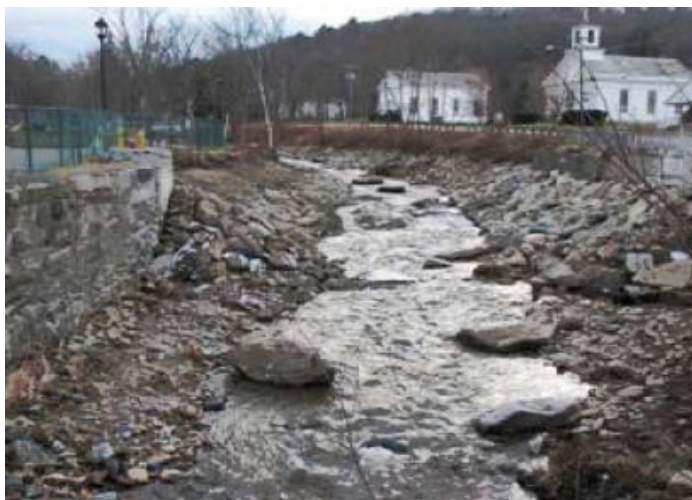
Boulders placed along the edge of restored stream channel to enhance fish passage upon removal of Ballou Dam in Becket, MA
