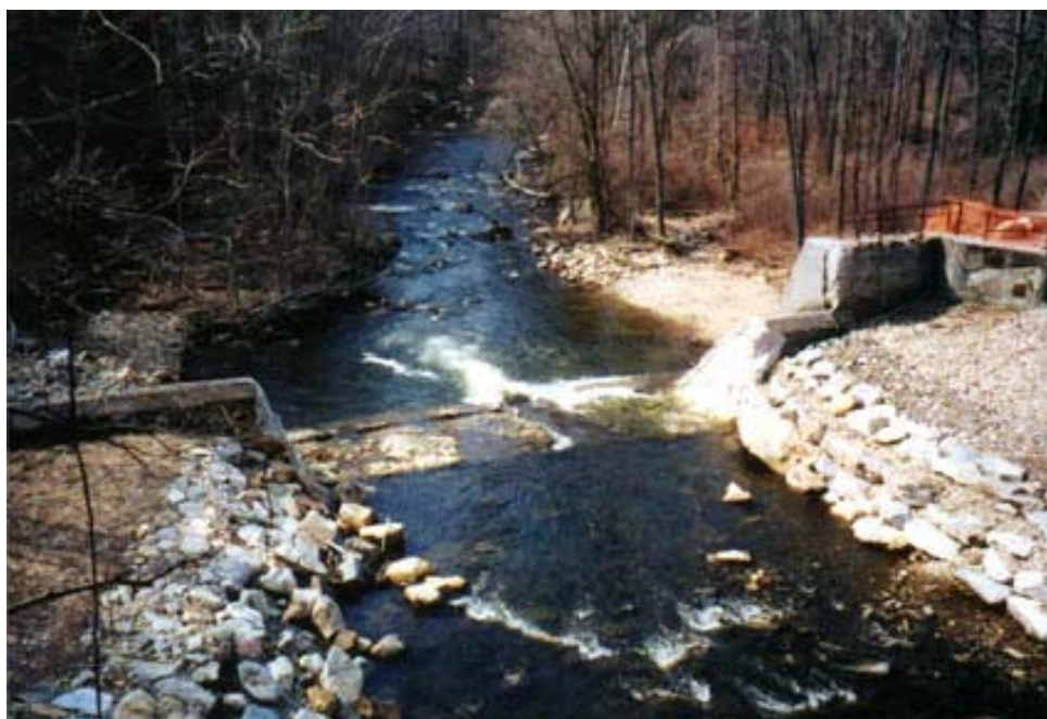
Fully breached site on the East Branch of the Housatonic River. Portions of the dam still remain. The sill of the dam is expected to degrade slowly and be replaced by a more natural stream bottom.
