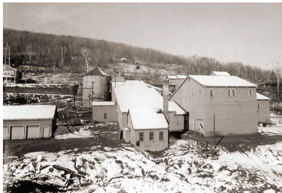
Two views of the World War II-era mine plant taken about 1960, shortly after the mine closed. Buildings were made according to wartime emergency temporary construction standards. Photo at right shows the cylindrical ore storage bin, flotation mill, and thickener/dryer building. The mill buildings were constructed using heavy timbers salvaged from a Bethel, Vermont, granite-cutting shed. Source for both photos: Collamer Abbott Collection, University of Vermont Library.
