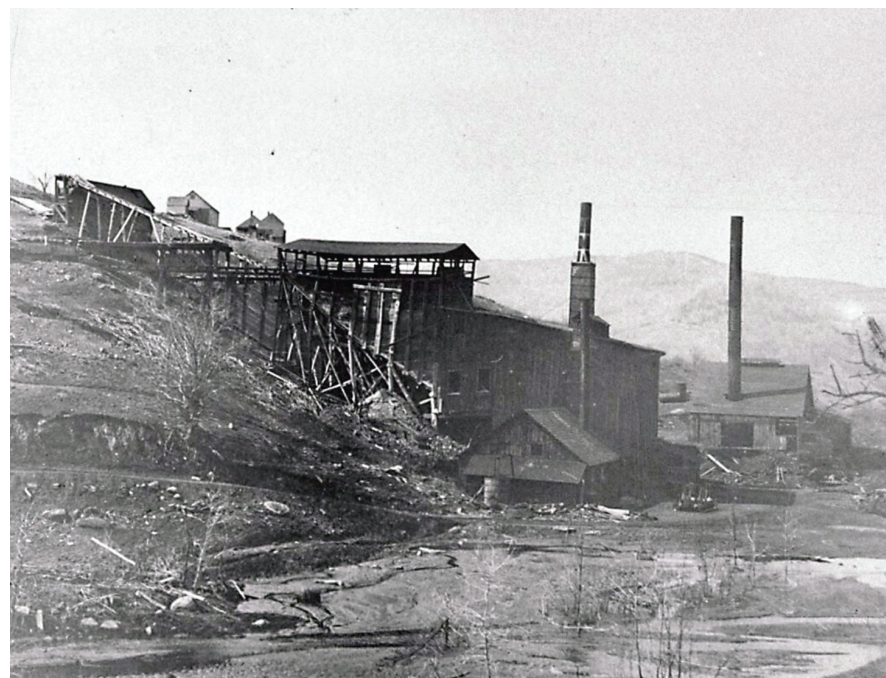
Tyson mill and roast beds, about 1900. The mine railroad trestle was used for delivering ore to roast beds. Sulfur fumes can be seen rising from roasting ore. Source: Collamer Abbott Collection, University of Vermont.
