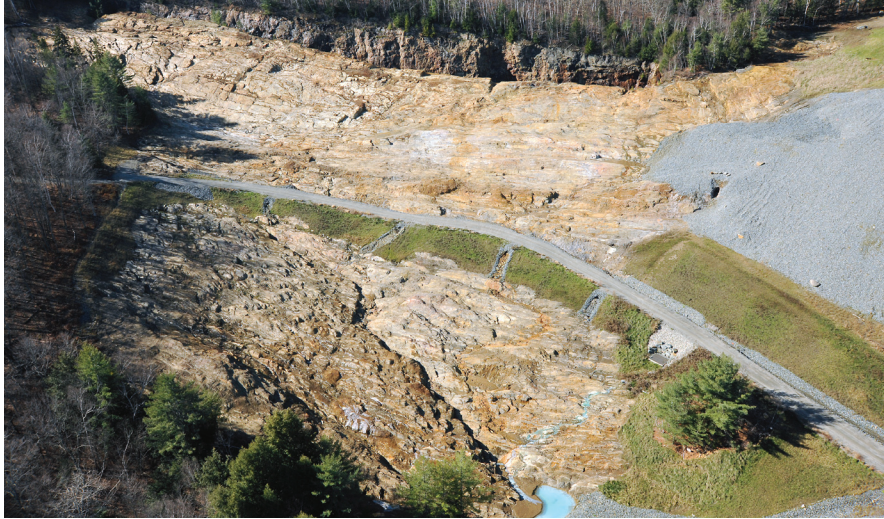
Once TP-3 was scraped clean, Copperas Road was reconstructed across it, and rock-lined drainage culverts were installed. Historic diagonal bedrock trench made to direct weak liquid copperas to the factories is clearly visible below the road. Waste removal resulted in over 95 percent reduction in copper discharge from the hillside. Source: U.S. Environmental Protection Agency.
