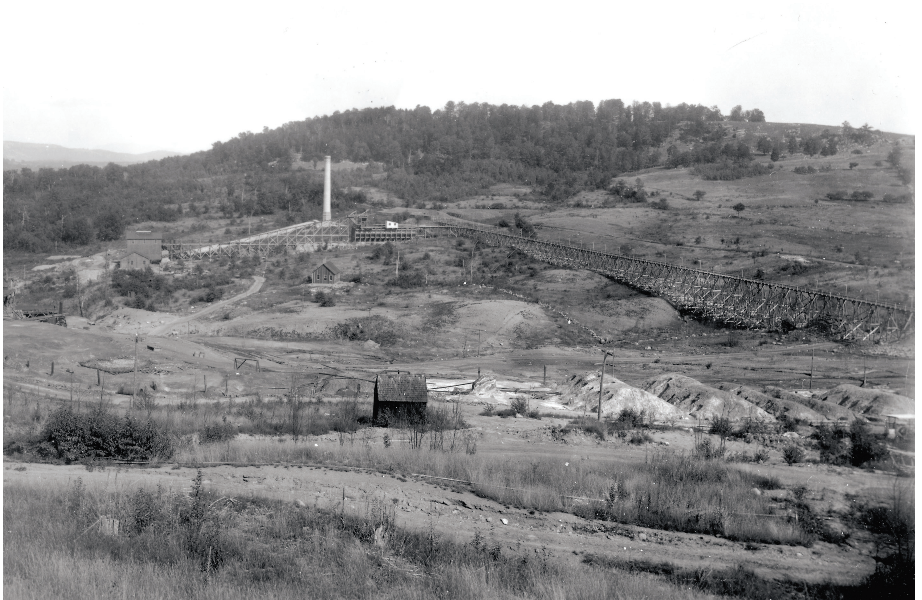
August Heckscher's Vermont Copper Corporation smelting plant about 1908. Ore was transported over the trestle at right and across to the smelter at left. Flue and chimney were for dispersing smelter fumes. Ore roast beds from the Tyson family's previous Elizabeth Mining Company smelting operation are in foreground. Source: Strafford Historical Society.
