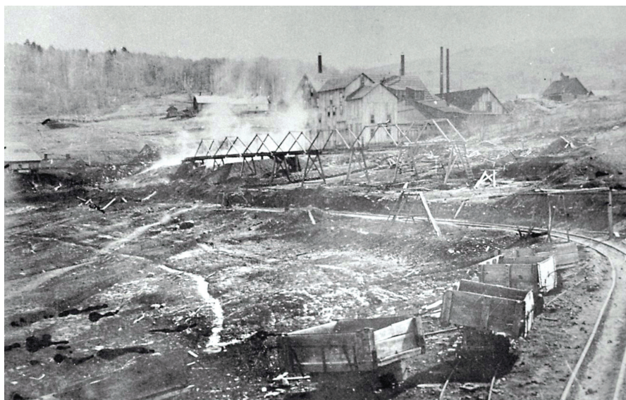
Tyson mill and roast beds, about 1900. The mine railroad trestle was used for delivering ore to roast beds. Sulfur fumes can be seen rising from roasting ore. Source: Collamer Abbott Collection, University of Vermont.
