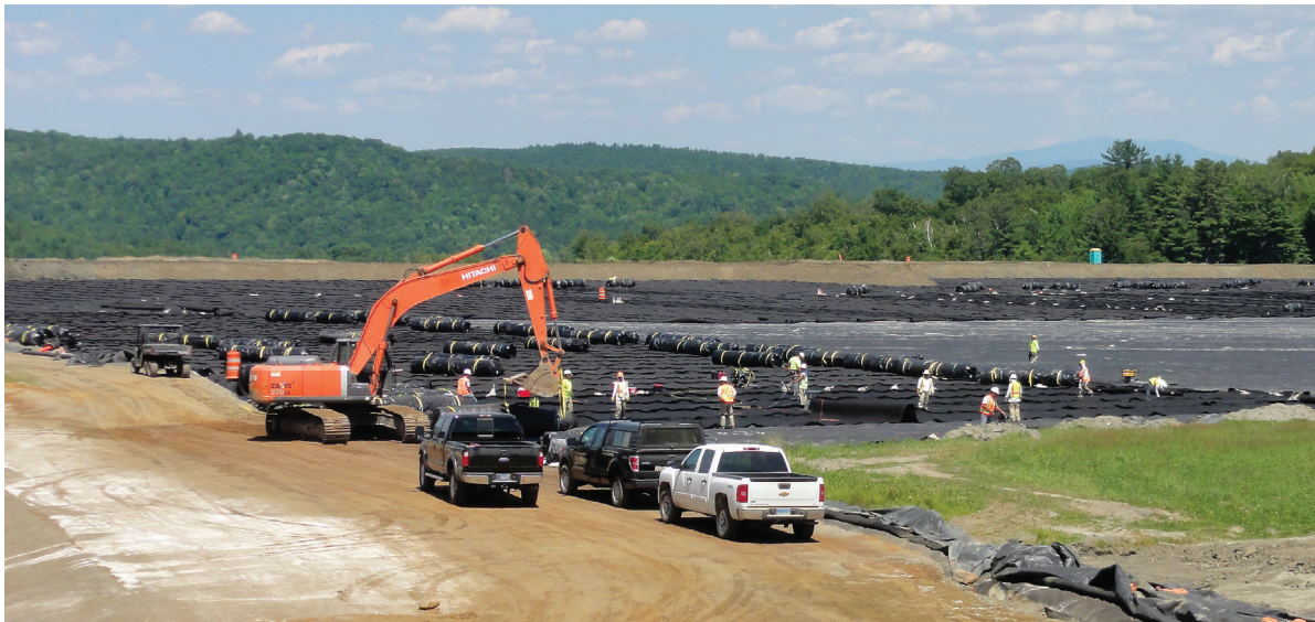
Once mine waste was consolidated on the tailings pile area, it was graded to shed water, and covered with an impermeable plastic barrier, which is being unrolled and sealed in this view across the top of the capped waste. The plastic barrier was then buried under two feet of soil. Source: U.S. Environmental Protection Agency.
