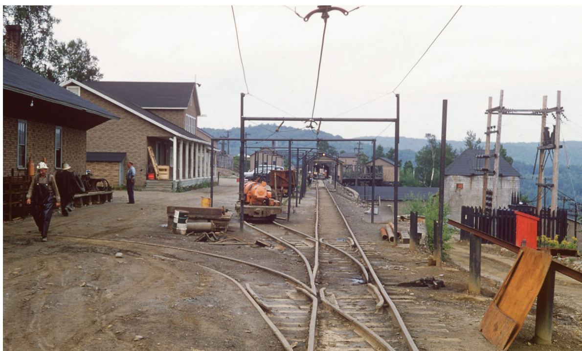
View looking north along the mine surface railroad, in the 1950s. Spur track at left leads into the machine shop, where mine locomotives, ore cars, and heavy equipment were serviced and repaired. The round concrete ore storage bin for the processing mill is at right. Source: Strafford Historical Society.
