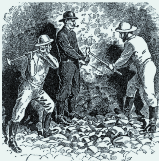
Miners using a manual drill and sledgehammers to bore a hole in rock. Source: International Correspondence Schools, 1907.
