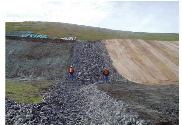
The top and sides of the sealed cap were covered with over two feet of soil, which was treated with lime, fertilized, and planted with grass. Rock-lined trenches divert surface runoff off and around the cap. Water filtration has been reduced so that the tailings now discharge less than 100 pounds of dissolved iron per day — about 88 percent less than the peak discharge of 800 pounds per day. Source: U.S. Environmental Protection Agency.
