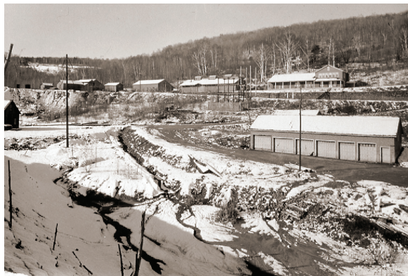
Two views of the World War II-era mine plant taken about 1960, shortly after the mine closed. Buildings were made according to wartime emergency temporary construction standards. Photo at right shows the cylindrical ore storage bin, flotation mill, and thickener/dryer building. The mill buildings were constructed using heavy timbers salvaged from a Bethel, Vermont, granite-cutting shed. Source for both photos: Collamer Abbott Collection, University of Vermont Library.
