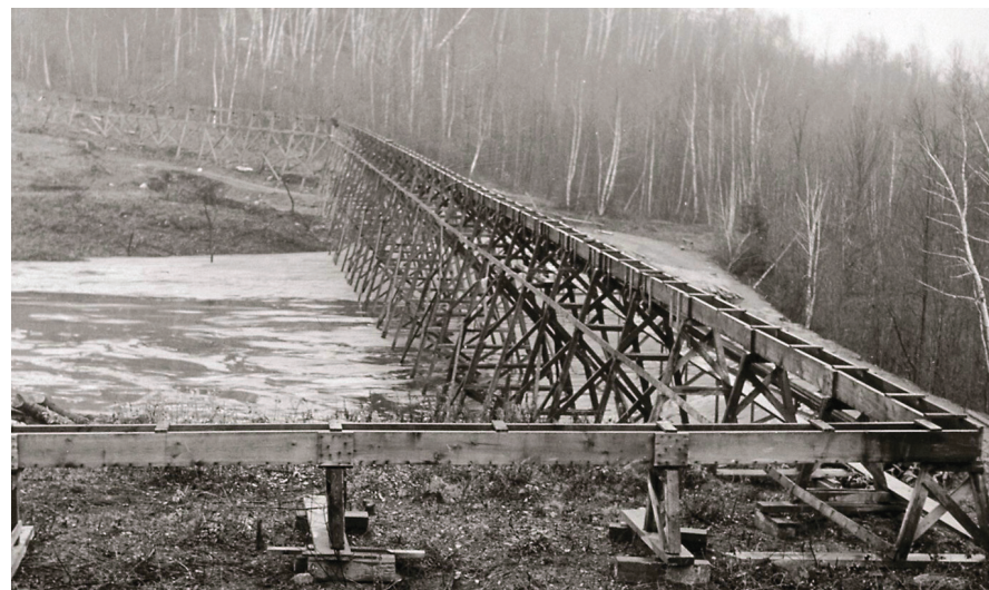
The unwanted ground waste tailings were pumped away from the flotation mill in a liquid slurry through a "launder"—a series of pipes and troughs that led out to the tailings pile. Source: Strafford Historical Society.
