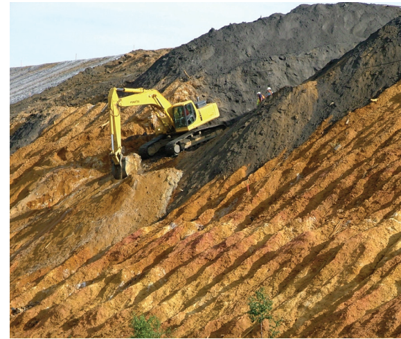
To prepare TP-1 for the waste repository, its steep, eroded sides were regraded for stability. Excavation revealed the unoxidized black pyrrhotite (iron sulfide) under the weathered outer orange layer of tailings. Source: U.S. Environmental Protection Agency.
