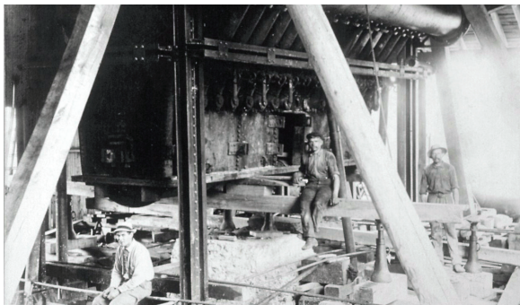
Vermont Copper Corporation blast furnace under construction, about 1908. The main air blast pipe and row of individual blast nozzles are visible above the detachable hearth. Source: Strafford Historical Society.
