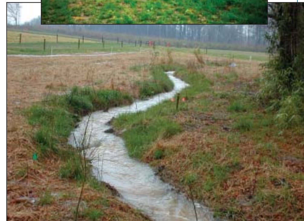
Figure 5.7 Yates Mill Pond tributary-restoration project after construction
