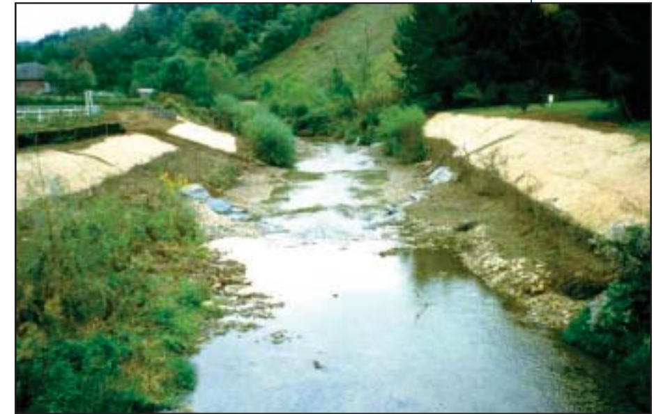
Figure 11.6 Cove Creek after restoration
