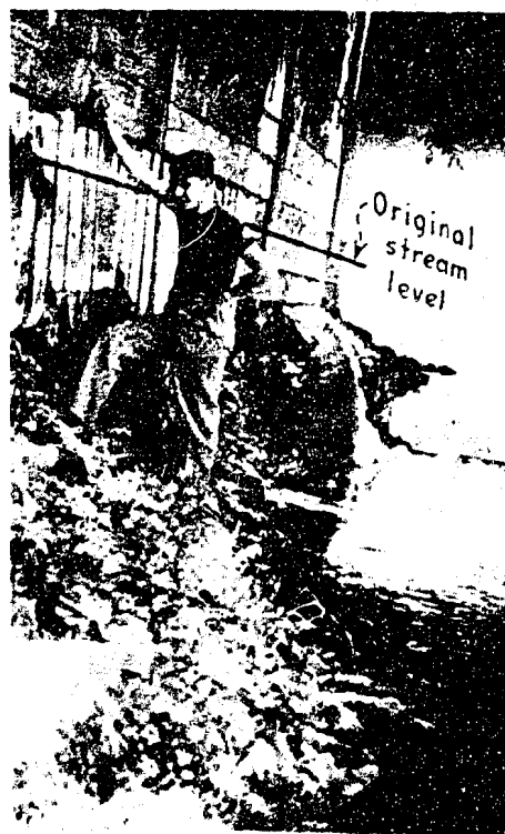
Figure 5. Bed Lowering in Cherry Creek, Denver, Colorado, Caused by Reduction of Sediment Load
