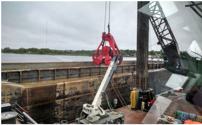
The dredge plant Dale Pyatt loading the scow Mighty Quinn
