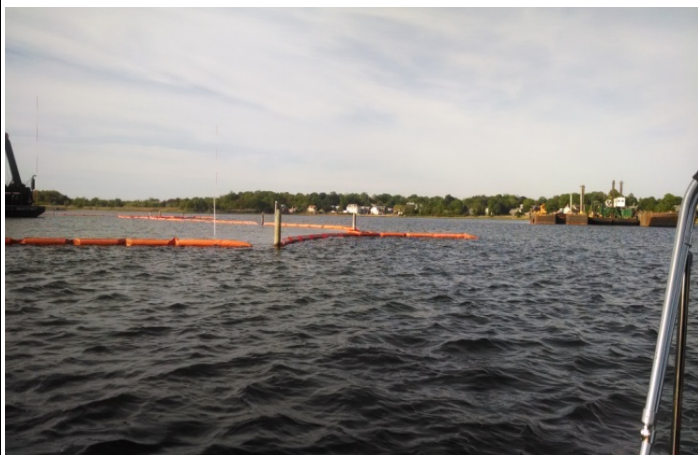
Silt curtain reattached to the pylon
