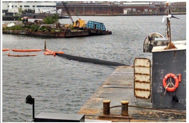
The northern silt curtain being lifted by the wind.
