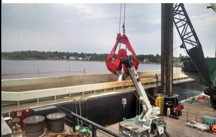
The dredge plant Dale Pyatt dredging into the scow M.E.R.C. Shevlin.
