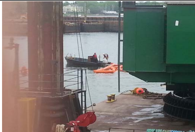
Dale Pyatt crew repairing damaged silt curtain.
