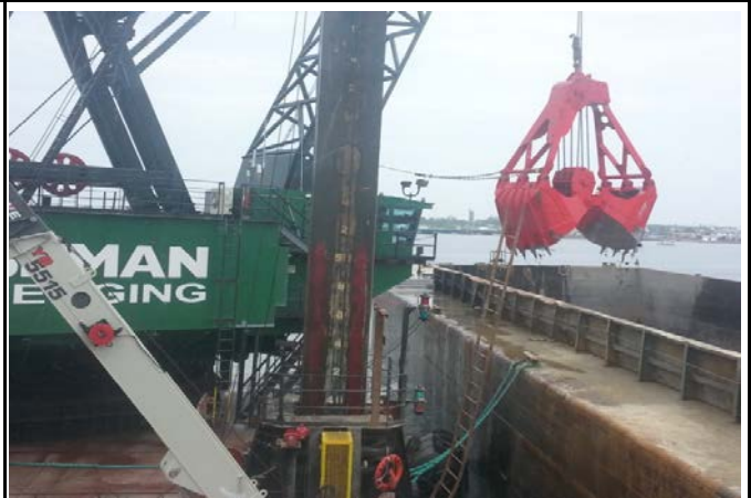
Dale Pyatt placing material from LHCC into the Mighty Quinn
