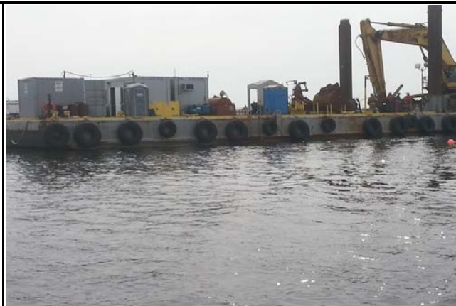
Photo 2: The crew on the Bobby D changes the bucket on the new excavator.
