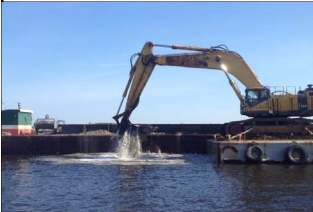
Bobby D. Dredging in Cut 6 in the Northeast corner of the CAD Cell.
