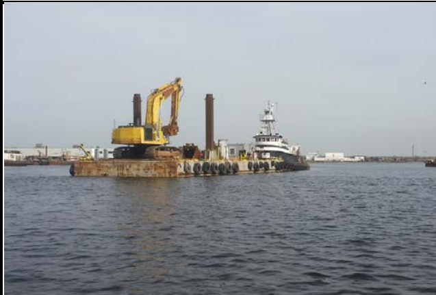
Photo 1: The Bobby D with a new excavator on board.
