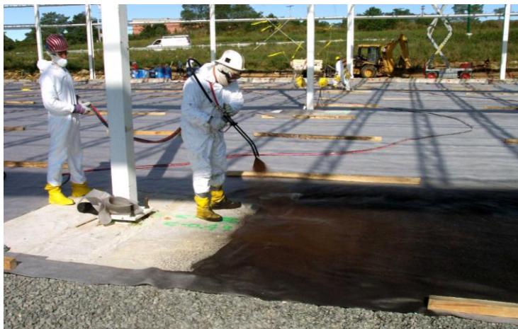
Figure 4-1. Liquid Boot® being applied during construction. Courtesy LBI Technologies, Inc.
