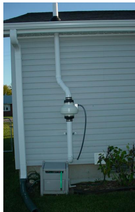
Figure 4-3. Active subslab depressurization system.
