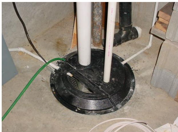
Figure 4-2. Passive sump mitigation system.
