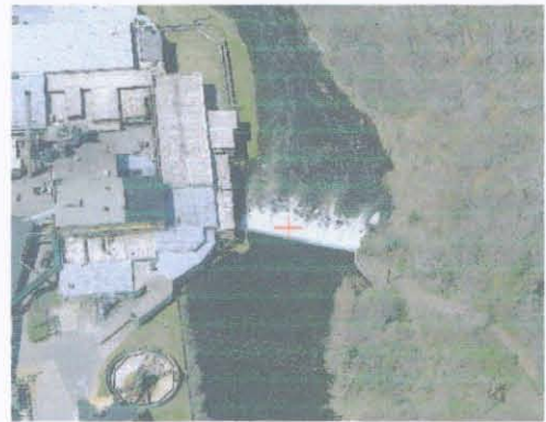
Columbia Mill Complex and Dam
