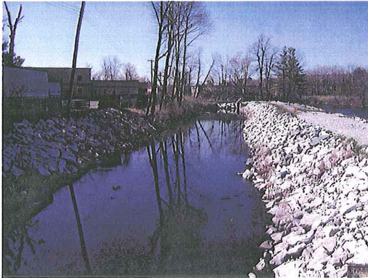
Woods Pond Dam Quarterly Inspection – April 27, 2006 Raceway Channel Looking Downstream
