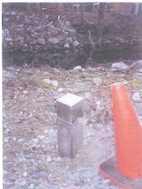
Photo 12 Orange cone identifying piezometer locations on crest.
