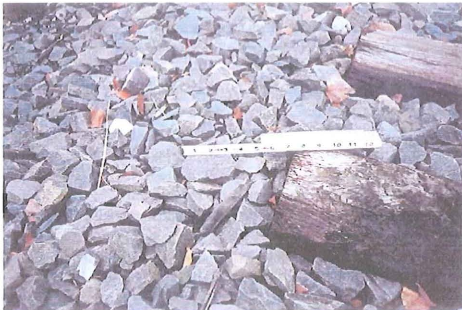
Photo C1 - Typical Railroad Ballast
