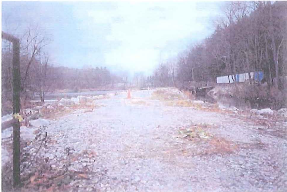
Photo 13 View of crest of raceway embankment from downstream (south) end near raceway sluice structure looking upstream (north). Orange cone shows indicates location of crest piezometer.
