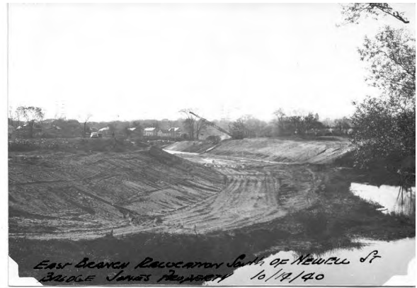
Channelization of the East Branch in Pittsfield (Source: City of Pittsfield Department of Public works & Utilities)
