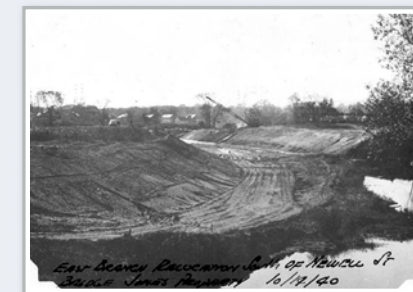
Channelization of the East Branch in Pittsfield
