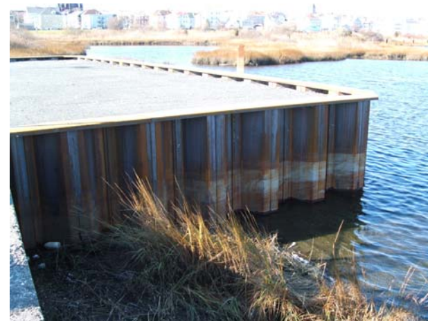
Figure 5.2-4 Completed East side of landing, after grading.
