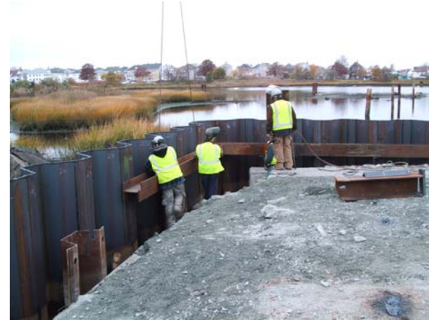
Figure 5.2-2 Installing H Beams
