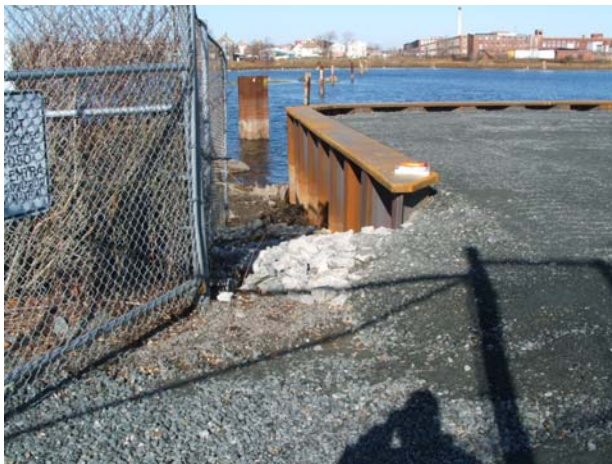
Figure 5.2-3 Completed West side of landing, after grading.
