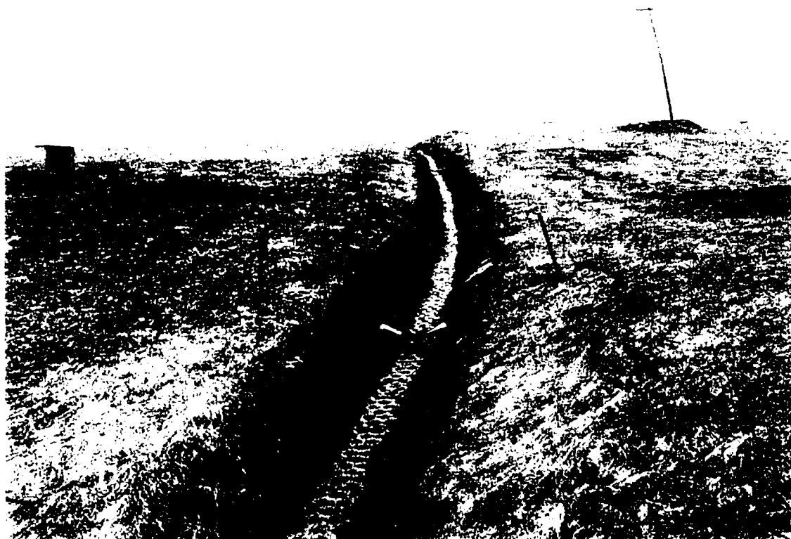
Photo 5: Middle Fabri-Form ditch, facing west.
