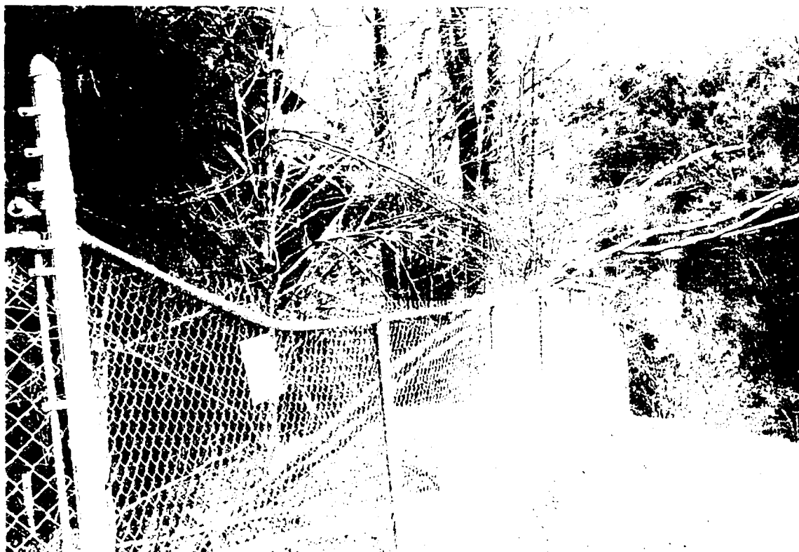
Photo 13: Damaged barbed wire fence near north Fabri-Form ditch, east of Gate C.
