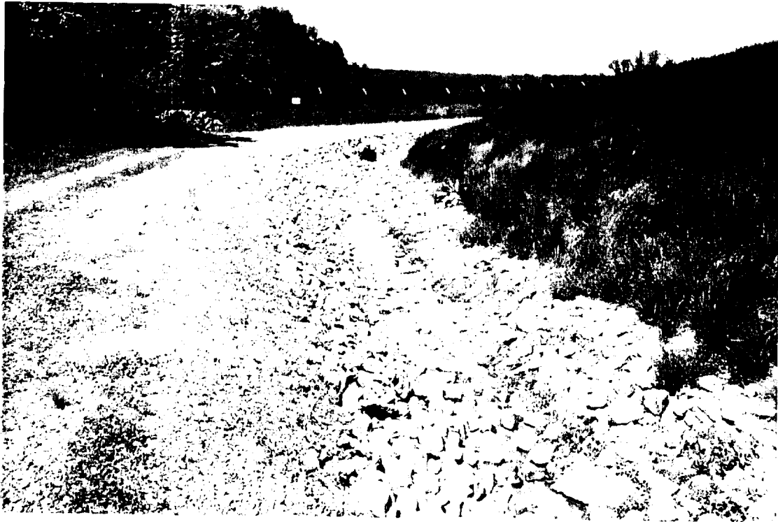
Photo 7 Sedimentation in southern perimeter ditch near manhole MH-1E, facing west.
