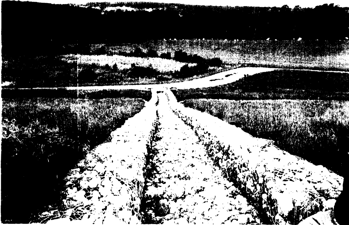
Photo 5 Downchute #4, from top facing west.
