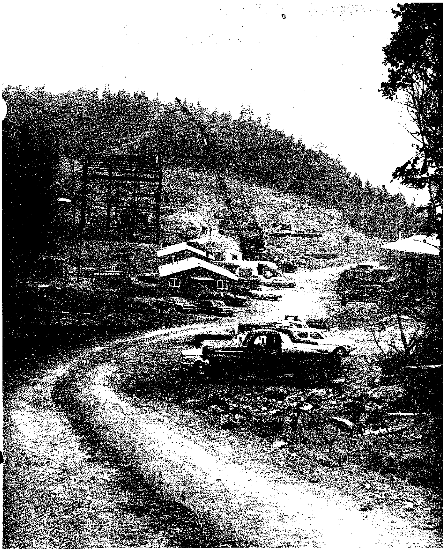
road leading to the mill. The building in the foreground is the office, at right the machine shop. Behind the office, a mill building takes shape as the steel framework is swung into place, girder by girder.--Packet photo.
