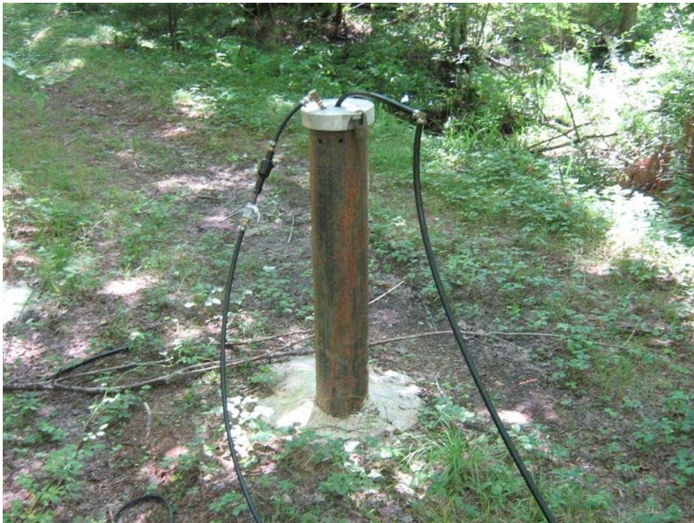
6. Pumping well MW-206(I).
