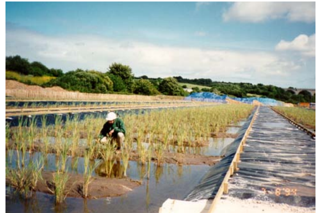
Figure 2. Aerobic cell at the Wheal Jane Mine, Cornwall, UK
