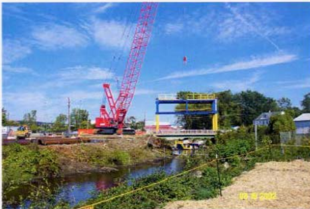
Photograph 2 – Placement of Sheet Pile Driving Platform in River
