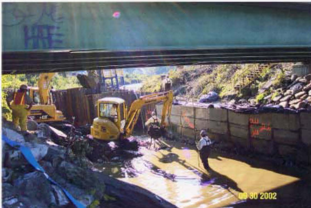
Photograph 4 – Excavation of Sediments at Cell 1A Beneath Lyman Street Bridge
