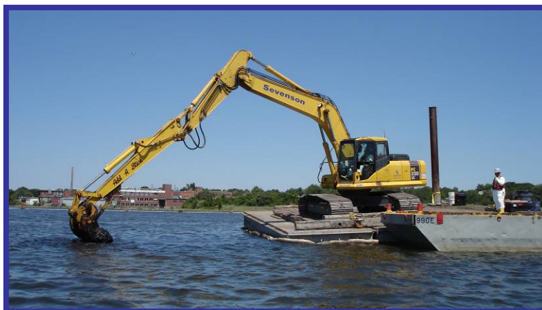
Figure 10. Debris Removal Excavator
