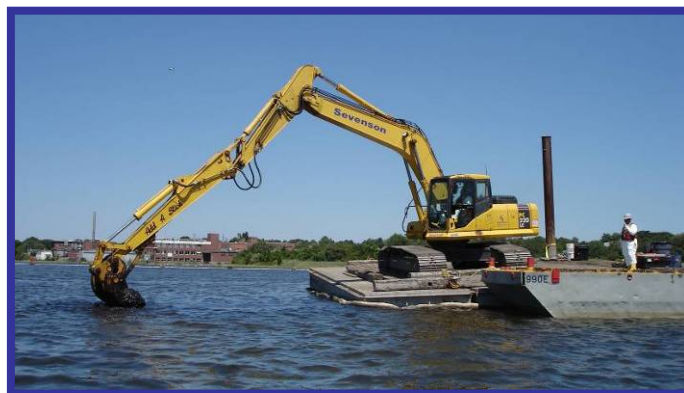
Figure 10. Debris Removal Excavator.
