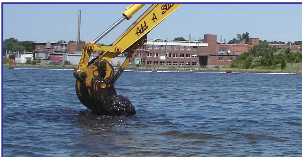
Figure 16. Debris Removal Generated the Majority of Turbidity Plumes
