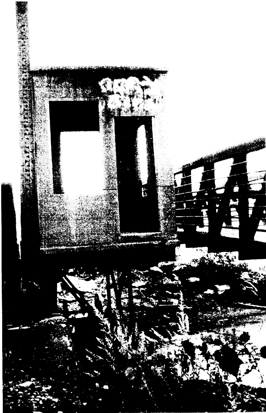
Plate 12. View of bridge operator's house to south.
