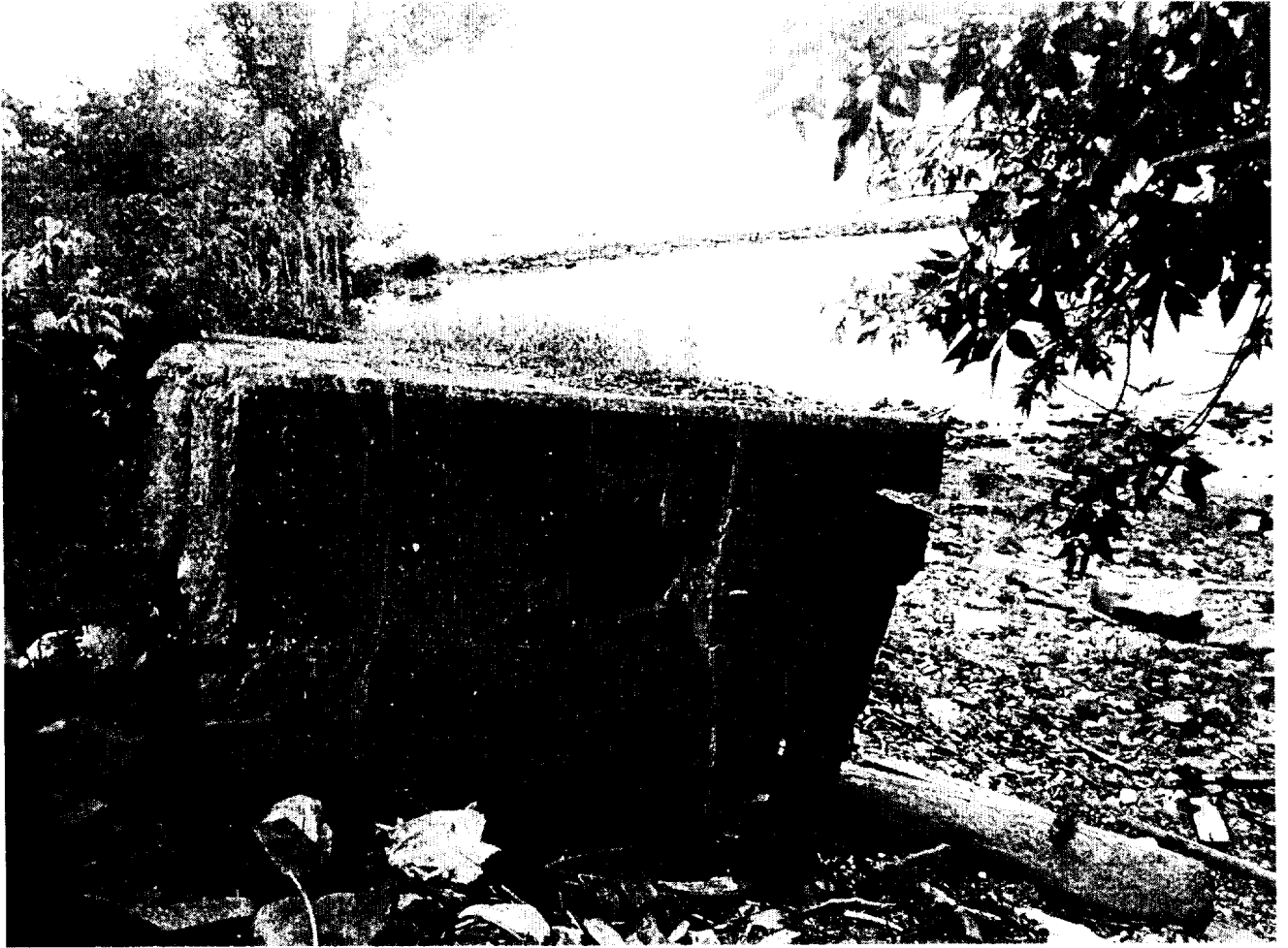
Plate 13. Portion of concrete bridge counterweight lying on ground next to bicycle path bridge. View to southwest. Note breakwater in background.
