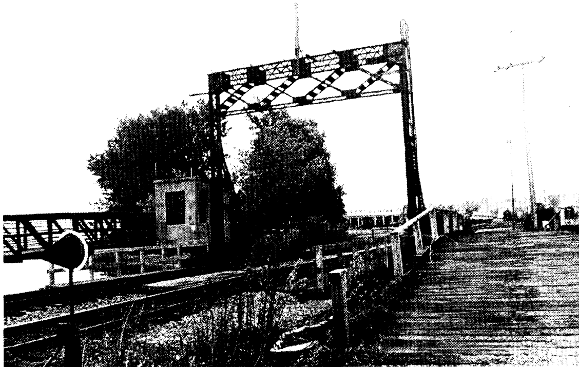
2) Barge canal railroad bridge. Toward north.
