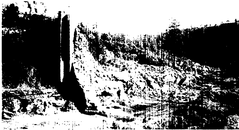
Figure 1.12 The 1933 collapse of Castlewood Dam on Cherry Creek in Colorado is an example of the result of unsafe dam construction and maintenance. Courtesy of the Denver Public Library, Western History Collection; photograph by Harry Rhoads.
