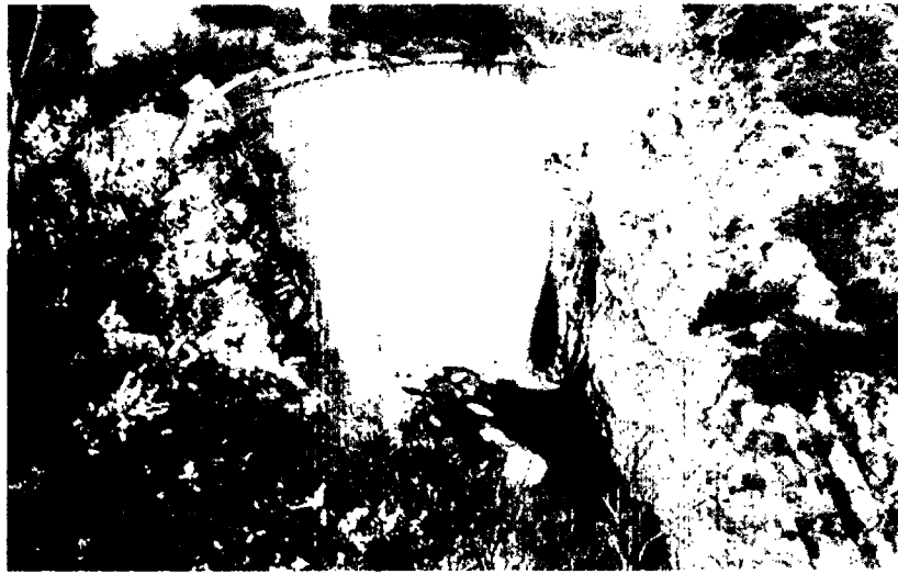
Figure 1.6 Rindge Dam, built in the 1920s on Malibu Creek in California, is an example of a concrete arch dam. Courtesy of Sarah Baisn.
