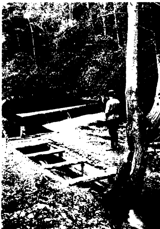
Figure 1.2 Forge Creek Dam in Cades Cove, in eastern Tennessee, is an example of a small, run-of-river structure. This view looks upstream from the west bank of the head-race and shows the main and diversion dams. A small diversion canal that supplied water to a mill is on the left. Courtesy of the Library of Congress, Prints and Photographs Division, Historic American Buildings Survey, Reproduction Number 5-CADCO, 1-24.
