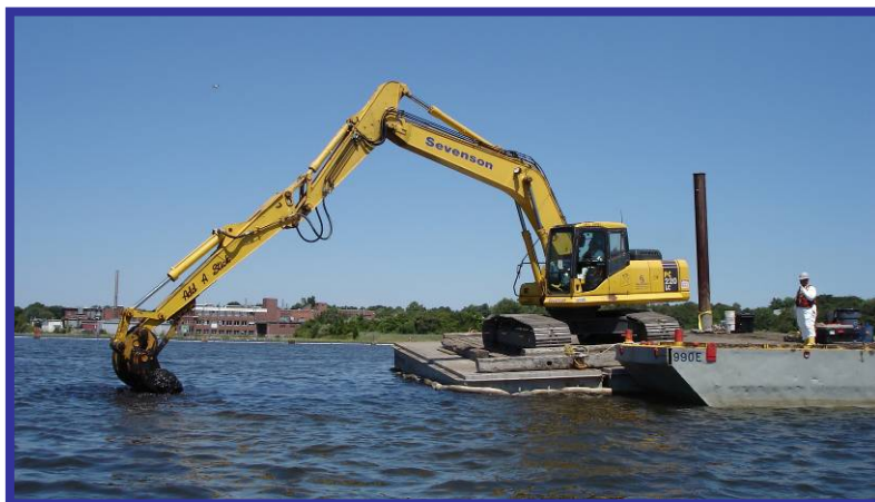
Figure 10. Debris Removal Excavator
