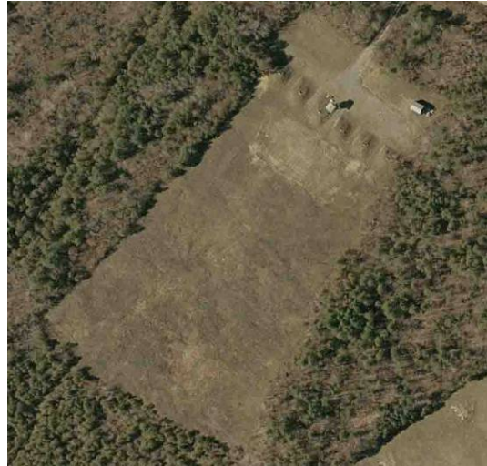
Figure 4-1. Aerial View of T Range before berm/STAPP construction
