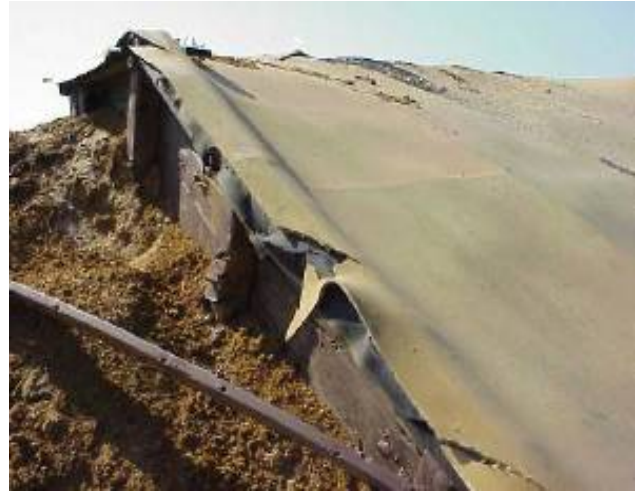
Figure 6-4. Example of Damage to STAPP™ Support Frame
