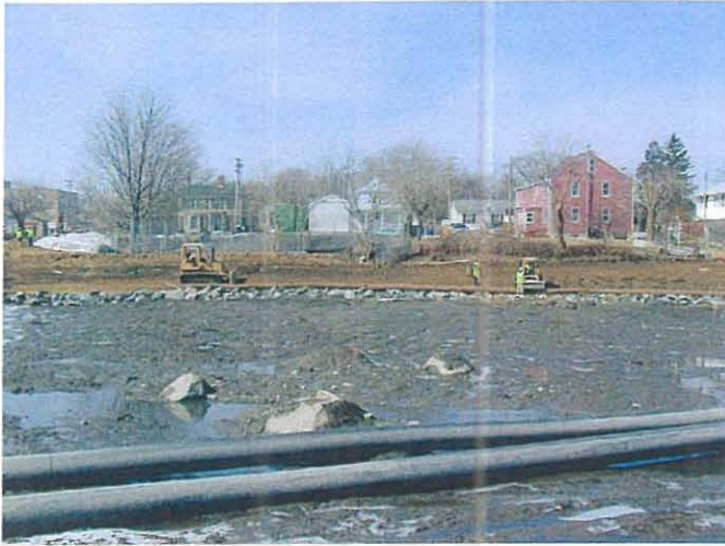
Restoration activities on the western shoreline
