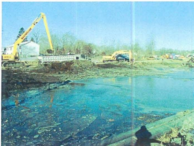
Load-out of vegetation material for off-site transport/disposal
