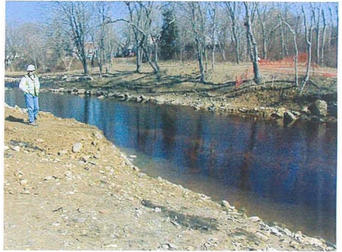
Site conditions following removal of the north berm Photo # WS32401 3/24/03 JPK
