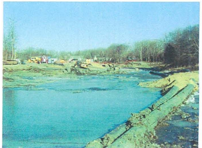
Post-excitation conditions at lumber yard zone
