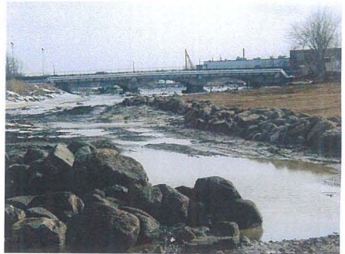
Restoration work at CSO/mudflat zone (W. shore)
