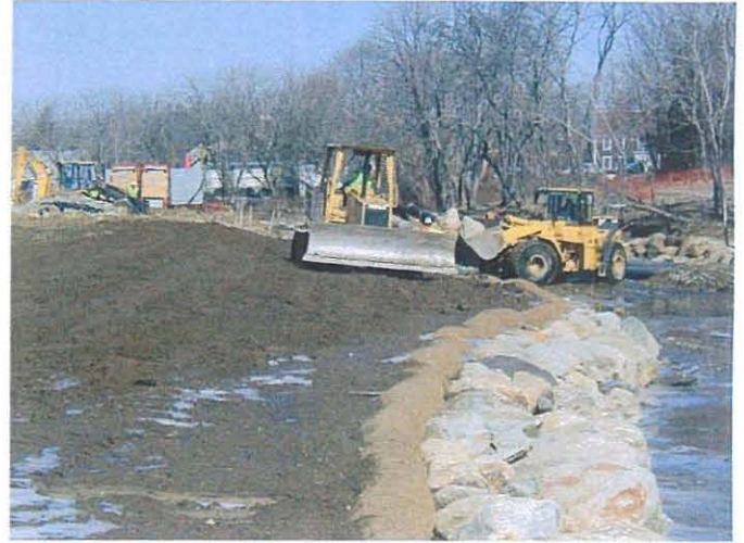
Topsoil grading and compaction at the lumberyard zone Photo # WS31103 3/11/03 JPK
