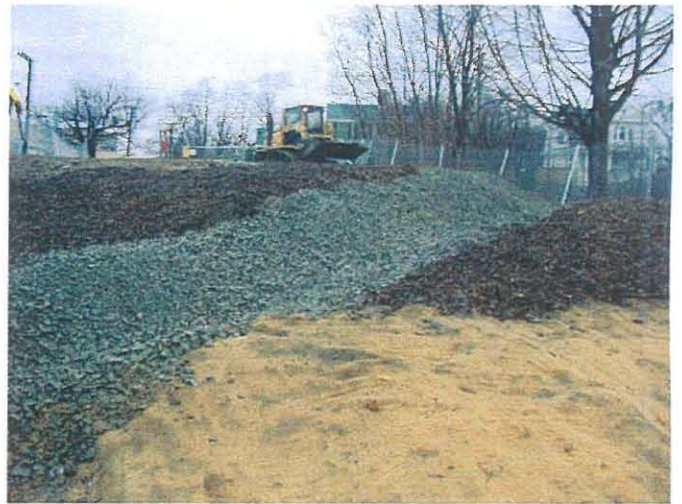
Construction of drainage swale north of bridge/lot grading Photo # WS40903 4/09/03 JPK
