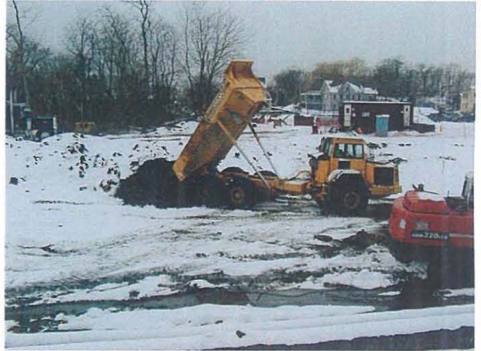
Transfer of excavated material with off-road trucks Photo # WS21003 2/10/03 JPK
