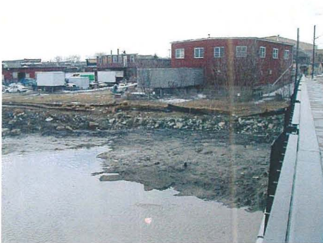
Post-restoration conditions: south zone, western shoreline
