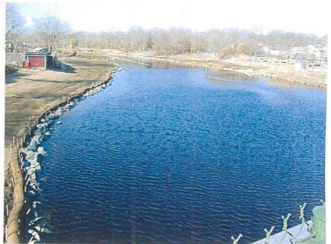
Restored conditions. Note: Water elevation = -0.5ft Photo # WS31907 3/19/03 JPK
