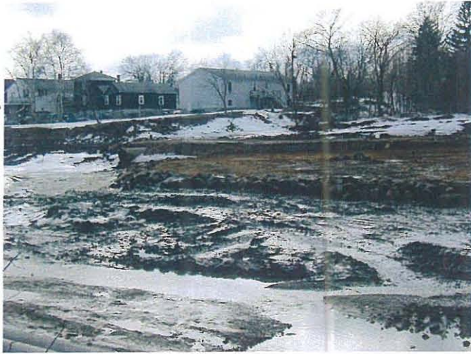
Restoration work at CSO zone Photo # WS30104 3/01/03 JPK
