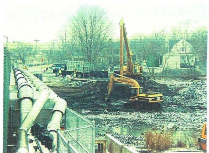
Sediment load-out operations at mudflat zone
