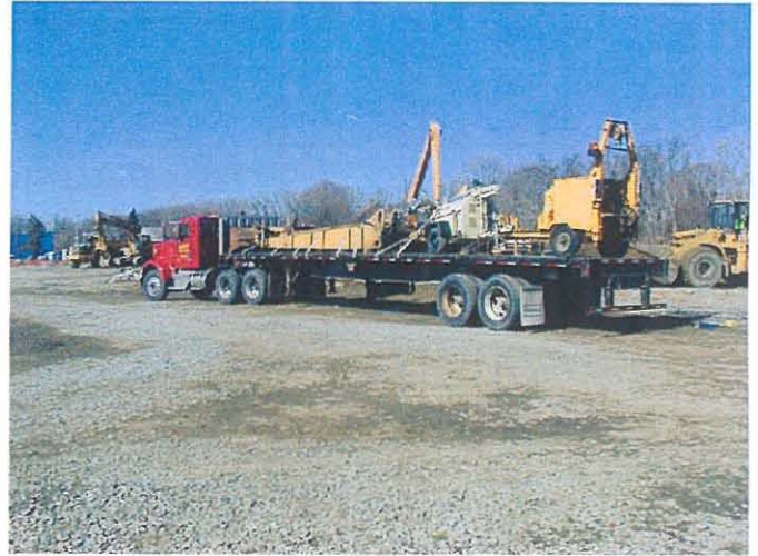
Demobilization of MT equipment from Lumberyard Photo # WS31901 3/19/03 JPK
