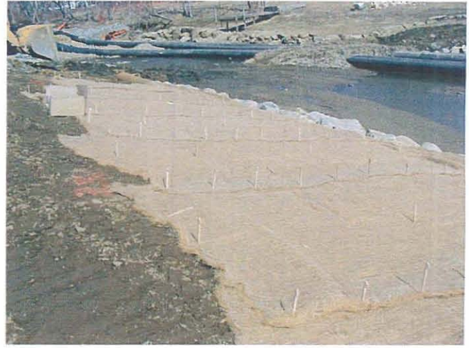
Installation of erosion control blanket at lumberyard zone
