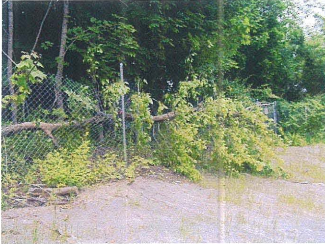
Fallen tree on fence at CSO Photo # WS61109 6/11/03
