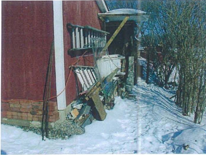
Santos shed – pre-excavation conditions Photo # WS21303 2/13/03 JPK
