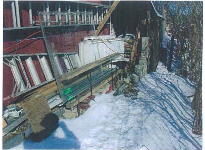
Santos shed – pre-excavation conditions Photo # WS21304 2/13/03 JPK
