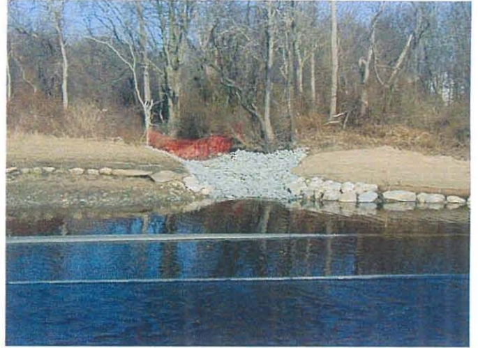
Drainage swale at south end of Braley property Photo # WS31802 3/18/03 JPK
