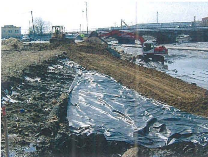
Backfill placement north of Titleist zone
