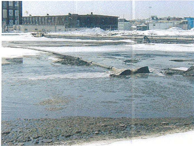
Slurry pipeline discharge in Cell #1 Photo # WS22008 2/20/03 JPK
