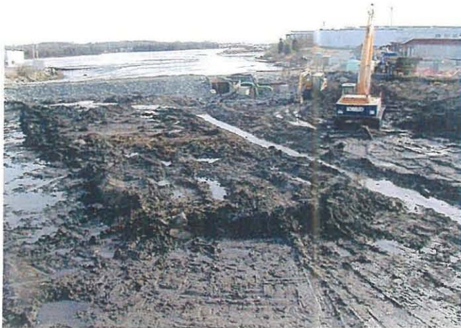
Excavation of the South Zone Photo # WS2301 2/3/03 JPK
