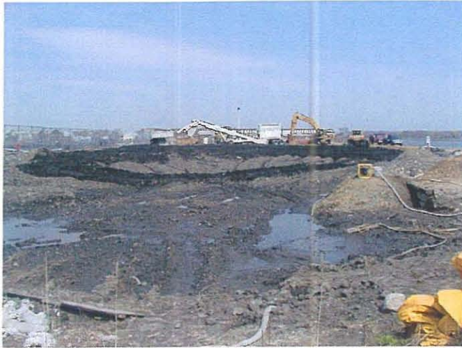
MT grading the Debris Disposal Area (DDA)
