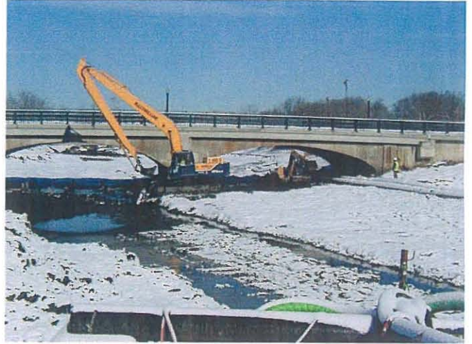
Excavation activities in the south zone
