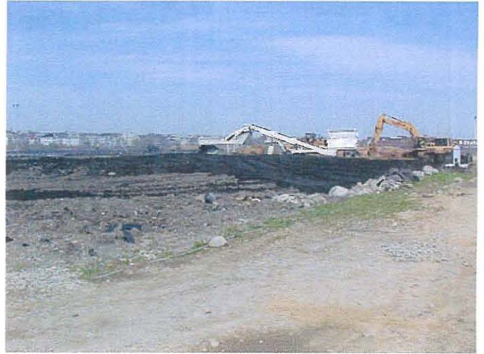
MT grading the Debris Disposal Area (DDA)
