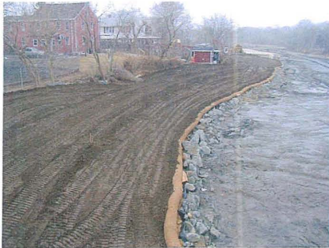
West shoreline: Post topsoil placement conditions
