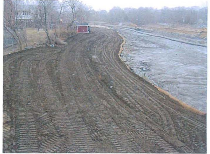
West shoreline: Post topsoil placement conditions
