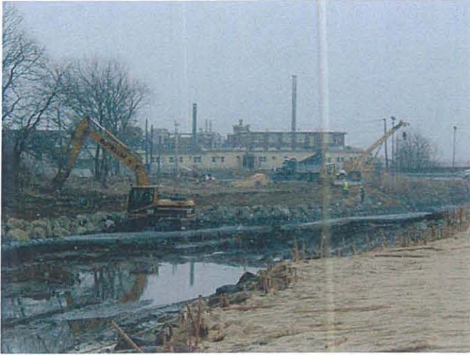
Restoration work underway on the eastern shoreline
