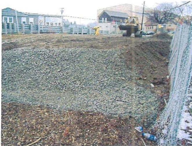
Construction of drainage swale north of bridge/lot grading Photo # WS40902 4/09/03 JPK
