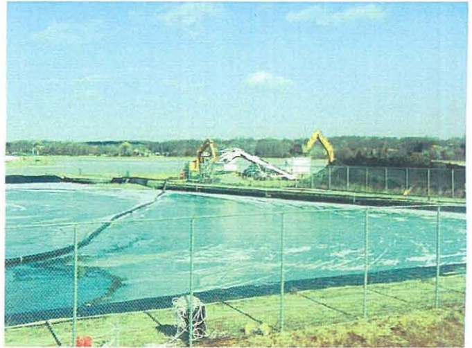
Screening operations at DDA/Cell 1
