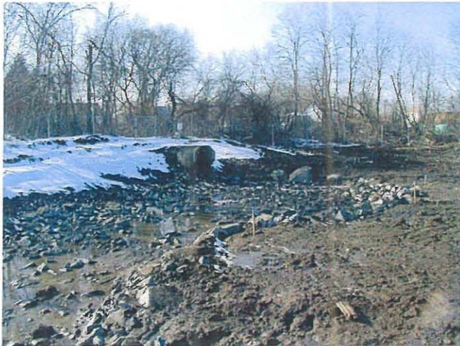
Placement of stone protection at the CSO outlet Photo # WS30805 3/8/02 JPK
