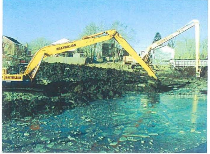
Excavation activities at mudflat zone
