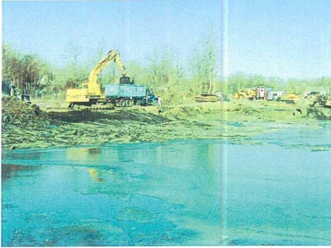
Load-out of sediments into haul truck for transport to DDA
