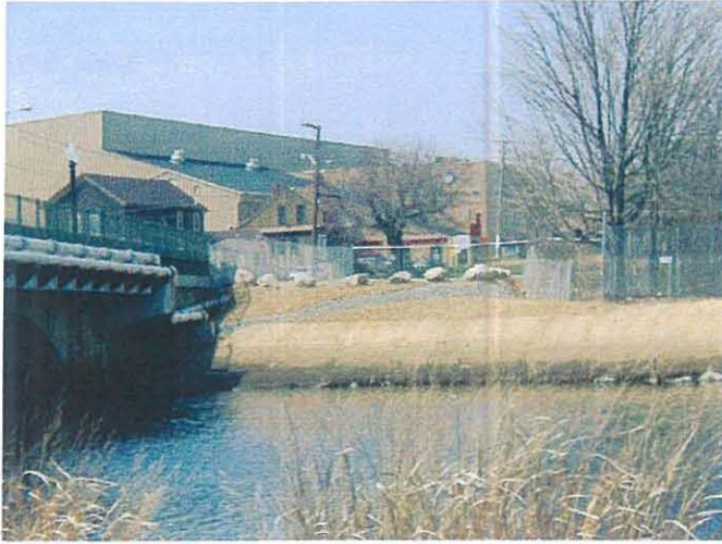
Drainage swale/stone protection at Wood St. access Photo # WS41601 4/16/03 JPK
