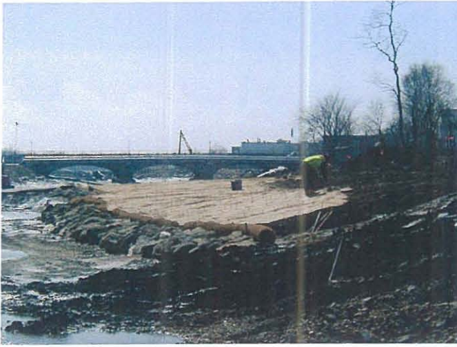
Installation of erosion control blanket at lumberyard zone
