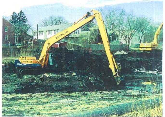
Excavation activities at mudflat zone Photo # WS12305 1/23/03 JPK
