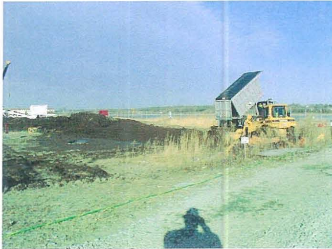
Transportation/disposal of excavated sediments at DDA
