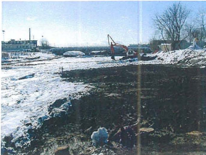
Excavation/removal of West haul road Photo # WS21402 2/14/03 JPK
