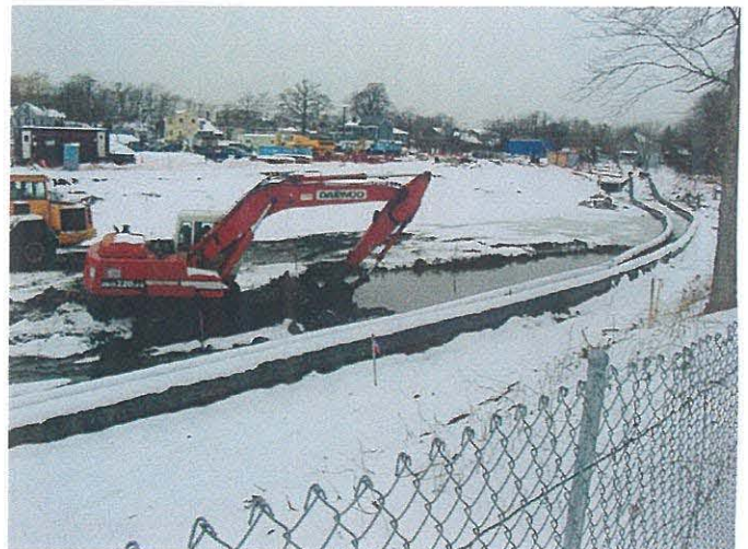
Excavation in lumberyard zone (in-river) Photo # WS21001 2/10/03 JPK
