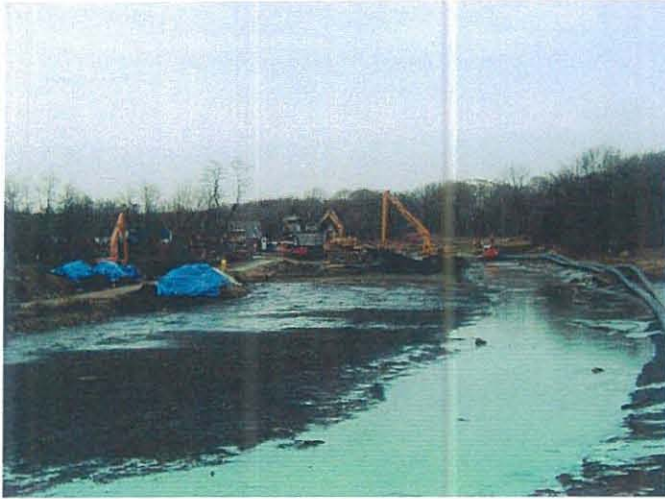
In-river excavation at lumber yard/CSO zone
