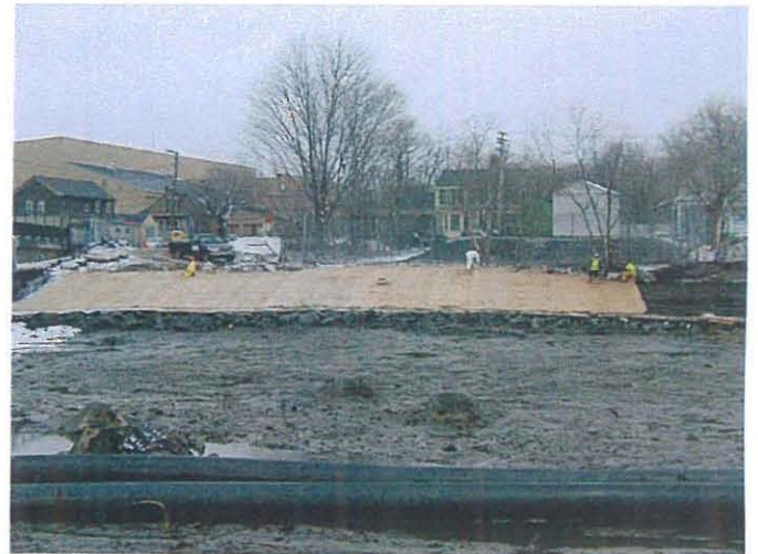
Restoration of western shoreline
