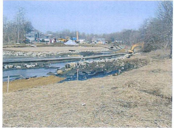
Stone protection/backfill placement on western shoreline
