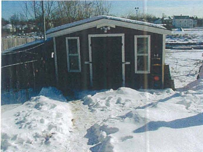
Santos shed – pre-excavation conditions
