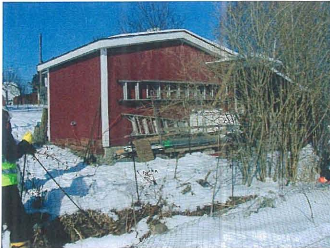
Santos shed – pre-excavation conditions Photo # WS21305 2/13/03 JPK
