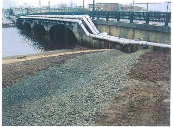
Drainage swale on west shore north of bridge Photo # WS40901 4/09/03 JPK
