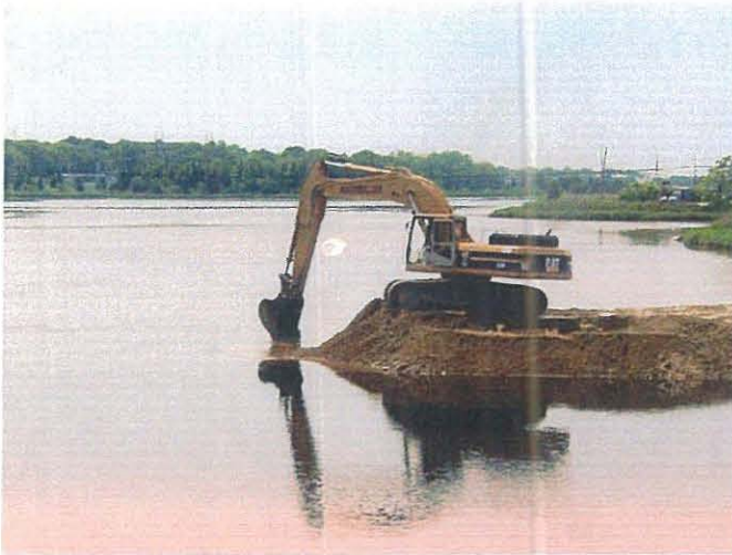
South berm removal Photo # WS62403 6/24/03
