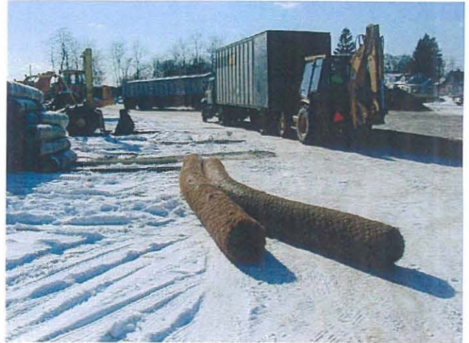
Delivery of coir fascines Photo # WS21401 2/14/03 JPK
