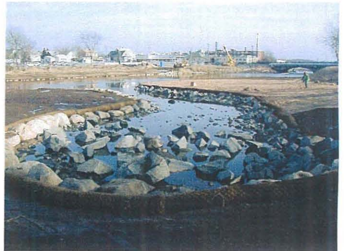
Restoration activities at the CSO zone Photo # WS31804 3/18/03 JPK
