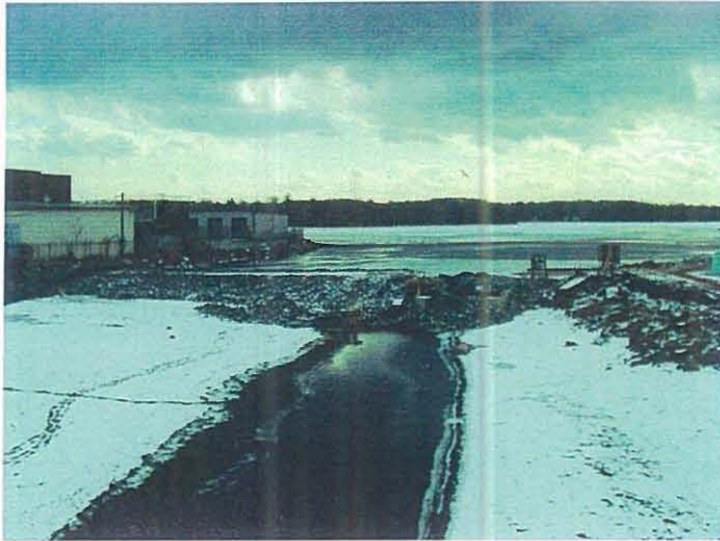
View of south berm from Wood St. bridge
