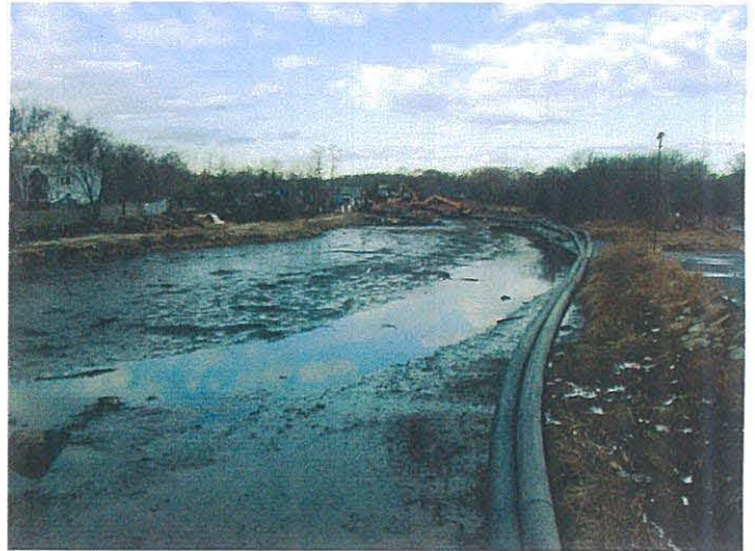
Acushnet River dewatered: Looking north from bridge Photo # WS1904 1/9/03 JPK
