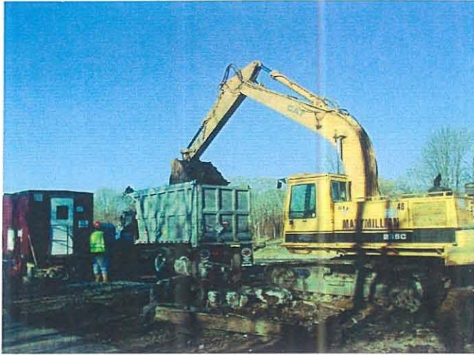
Load-out of sediments into MT haul truck for transport to DDA Photo # WS11504 1/15/03 JPK
