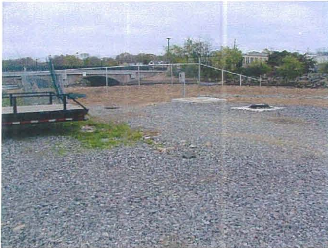
Installation of fencing at South Bern
