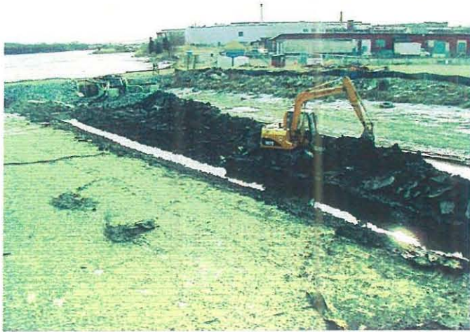
Excavation at the south zone Photo # WS12304 1/23/03 JPK
