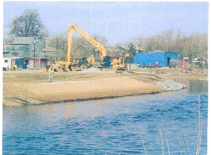
Installation of drainage swale/final grading at Lumberyard Photo # WS41502 4/15/03 JPK
