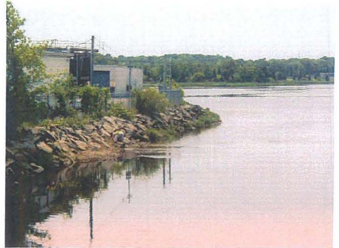
Clearing rip rap wall at south berm Photo # WS62404 6/24/03
