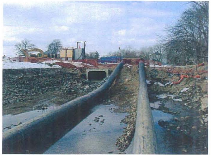
By-pass pumping system at North berm
