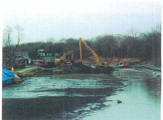
In-river excavation at lumber yard/CSO zone
