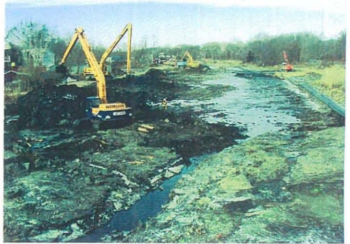
Excavation activities at mudflat zone
