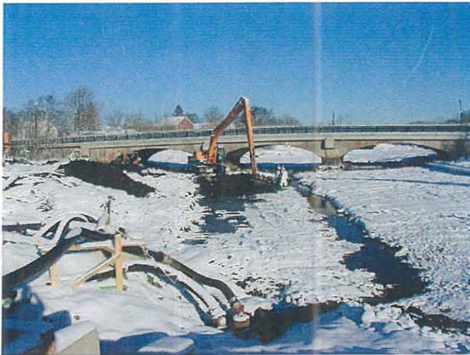
Excavation activities in the south zone Photo # WS21101 2/11/03 JPK
