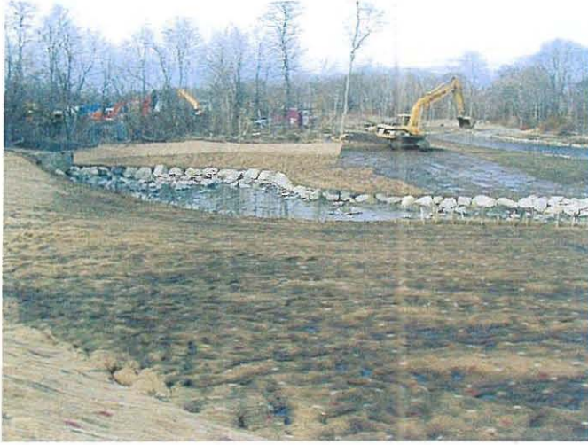
Restoration activities at the CSO zone Photo # WS32008 3/20/03 JPK
