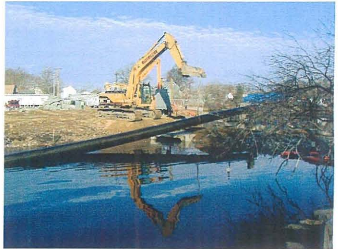
Removal of the by-pass piping from river Photo # WS32007 3/20/03 JPK
