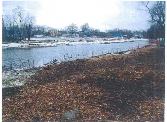
Area south of excavation at Acushnet Park
