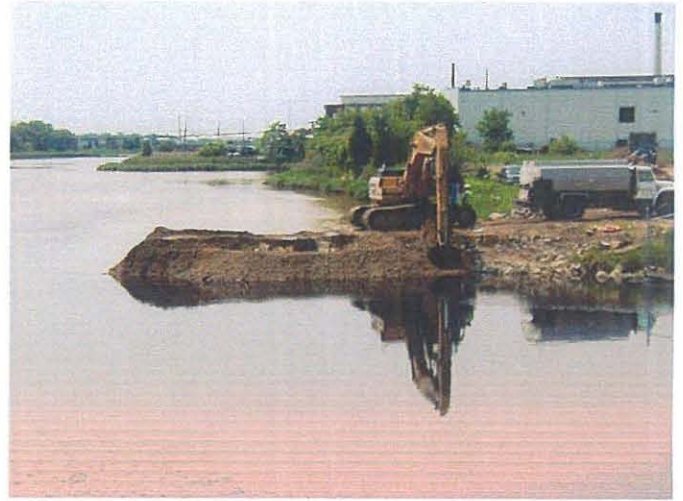
South berm removal Photo # WS62401 6/24/03
