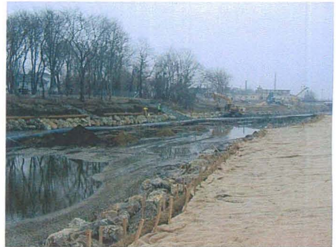
Restoration work underway on the eastern shoreline
