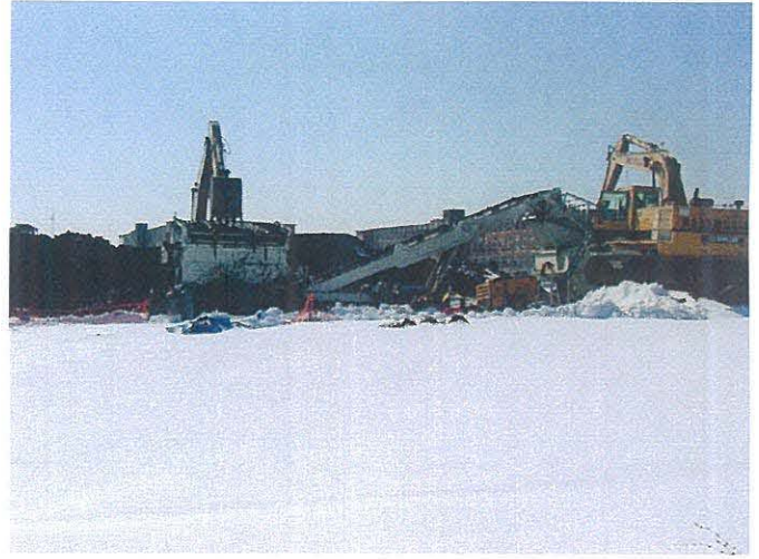
Screening/slurry operations Photo # WS22007 2/20/03 JPK
