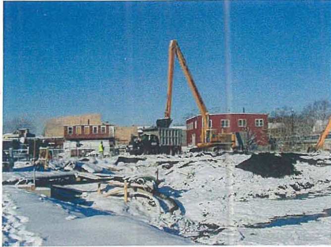
Load out of excavated material in the south zone
