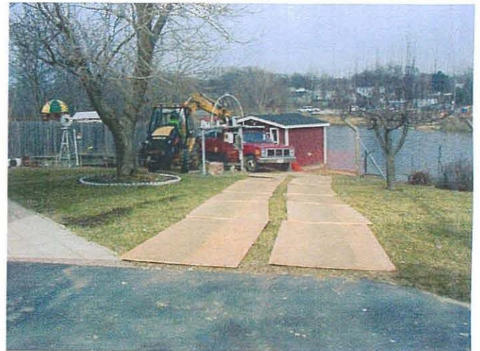
Excavation of the Santos' garden Photo # WS32501 3/25/03 JPK
