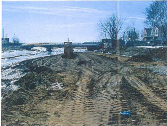
Topsoil grading at the CSO/mudflat zone Photo # WS31104 3/11/02 JPK
