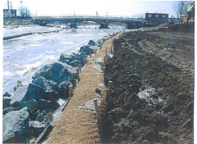
Installation of coir fascine Photo # WS31105 3/11/03 JPK
