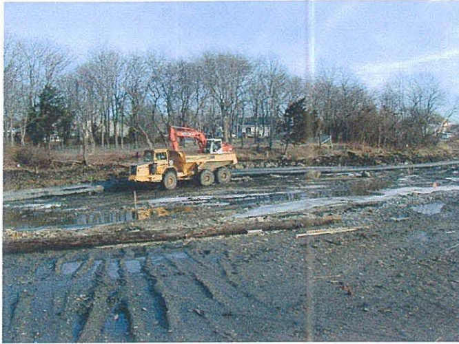
Excavation on the east shore near Acushnet Park Photo # WS2303 2/3/03 JPK
