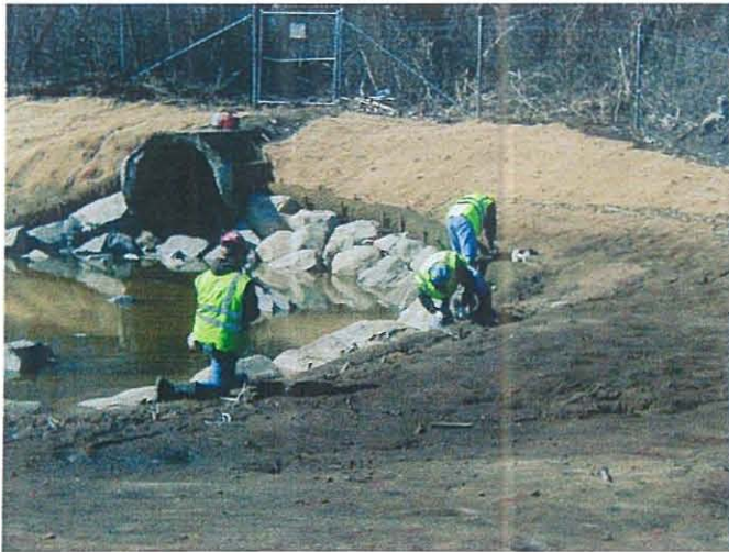
MT employees securing the coir logs Photo # WS32402 3/24/03 JPK
