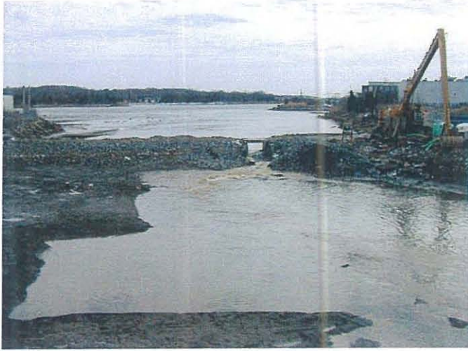
Opening of the south berm channel
