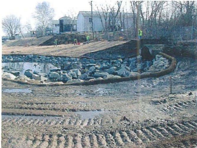
Restoration activities at the CSO zone Photo # WS31803 3/18/03 JPK
