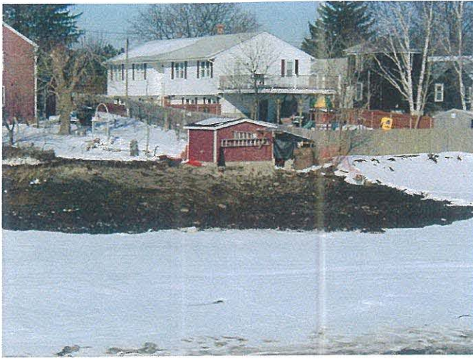
Excavation around the Santos shed/W. haul road Photo # WS22102 2/21/03 JPK
