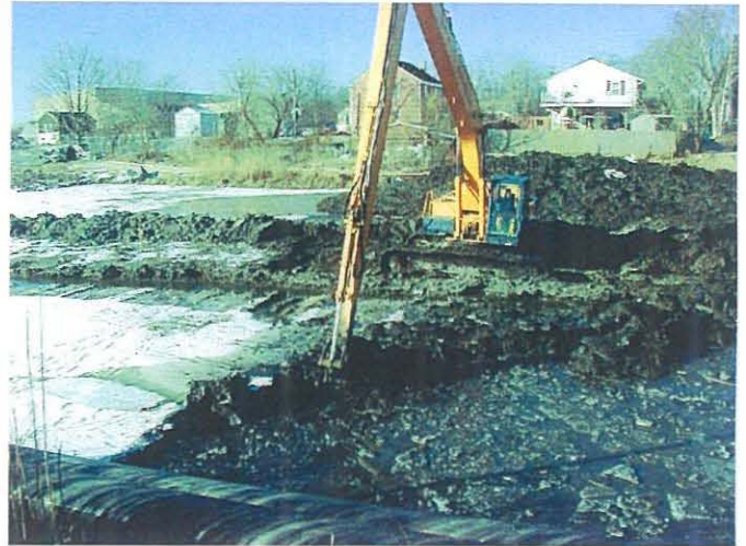
In-river excavation at mudflat zone
