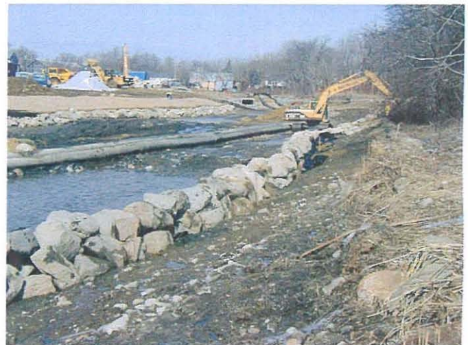
Stone toe placement on eastern shoreline
