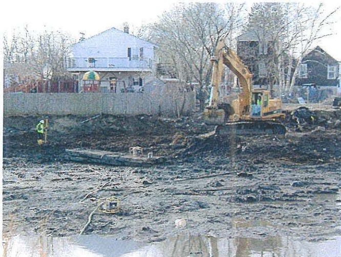
Removal of West haul road Photo # WS2503 2/5/03 JPK
