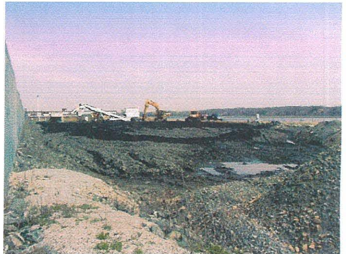
MT grading the Debris Disposal Area (DDA)
