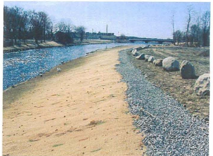
Drainage swale/restored slope at Lumberyard Photo # WS42501 4/25/03 JPK
