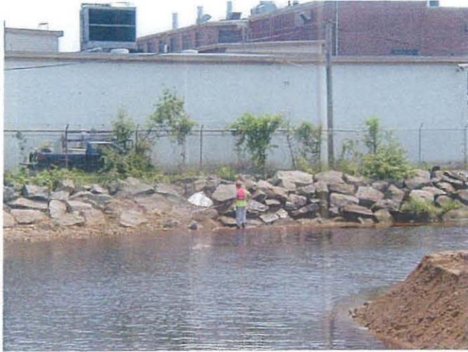
Cleaning rip rap wall at south berm Photo # WS62405 6/24/03
