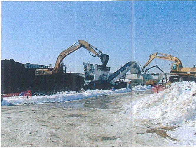
Screening/slurry operations Photo # WS22006 2/20/03 JPK
