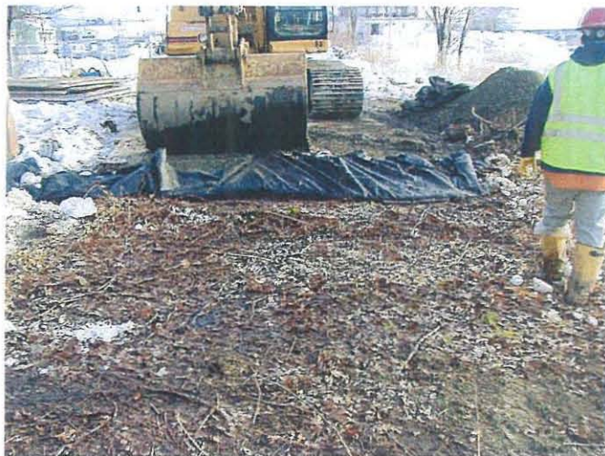
Removal of HDPE mats south of excavation at Acushnet Park Photo # NWS121202 12/12/03 MS
