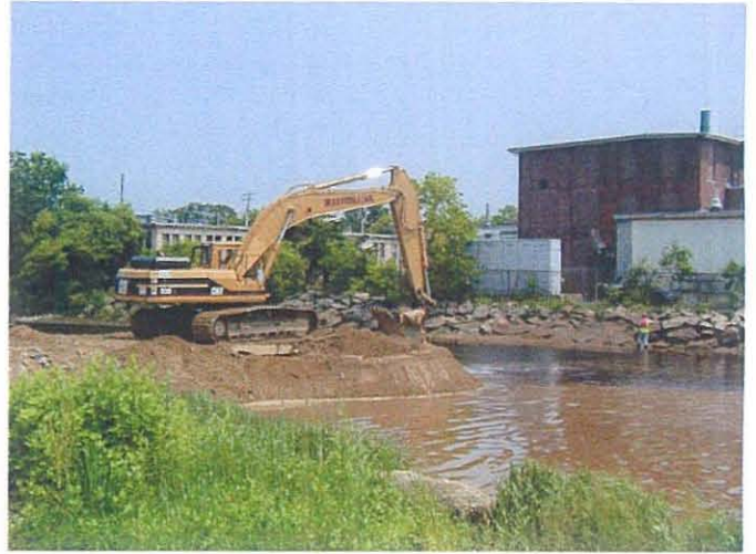
South berm removal Photo # WS62406 6/24/03
