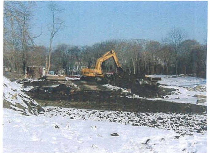
Excavation/removal of the West haul road Photo # WS21306 2/13/03 JPK
