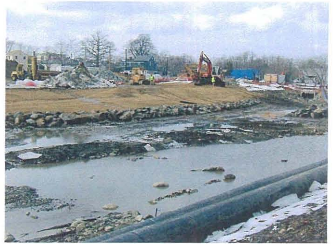
Restoration work at Lumberyard zone (W. shore) Photo # WS30105 3/01/03 JPK
