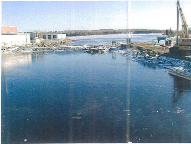
Conditions after berms opened due to heavy rain
