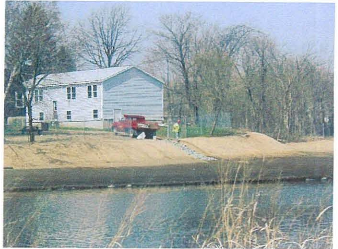
Drainage swale construction behind residences (W. shore) Photo # WS41602 4/16/03 JPK
