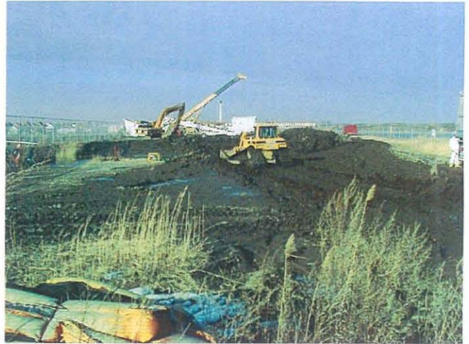
Placement/compaction of excavated sediments at DDA
