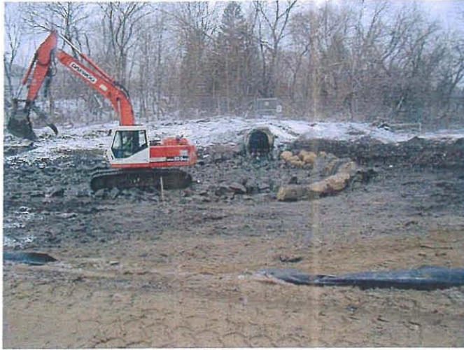
Placement of stone protection at the CSO outlet Photo # WS31306 3/13/03 JPK
