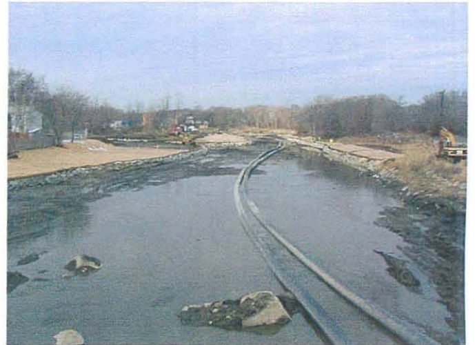
Restoration north of the Wood St. bridge
