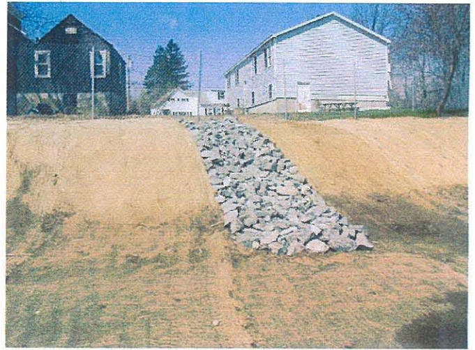
Drainage swale on W. shore, behind residences
