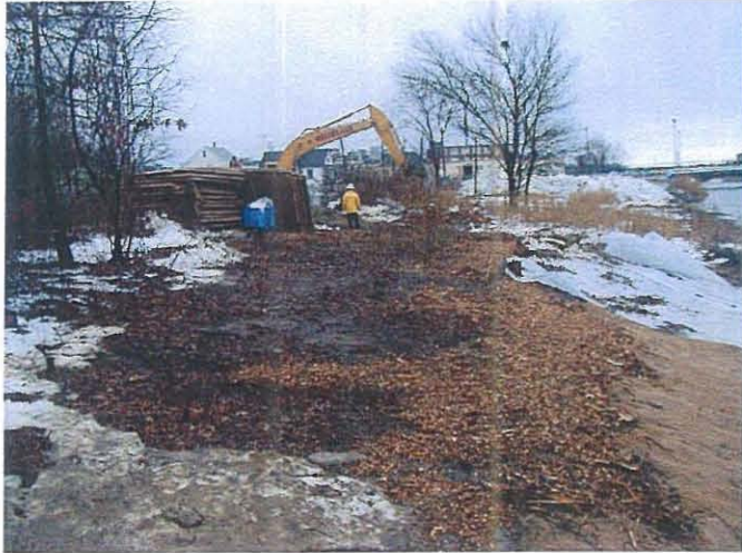
Area south of excavation at Acushnet Park
