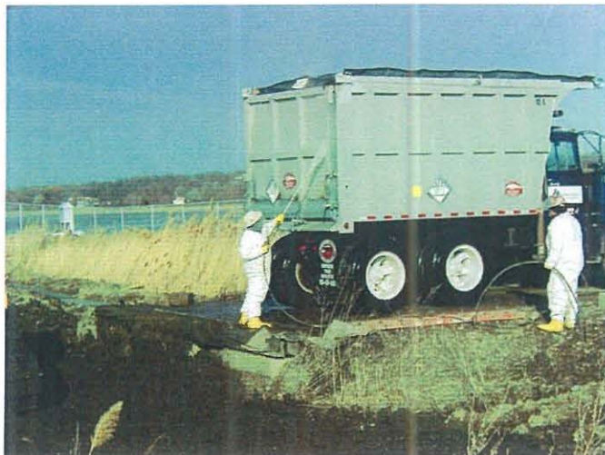
Decontamination of haul vehicle at DDA
