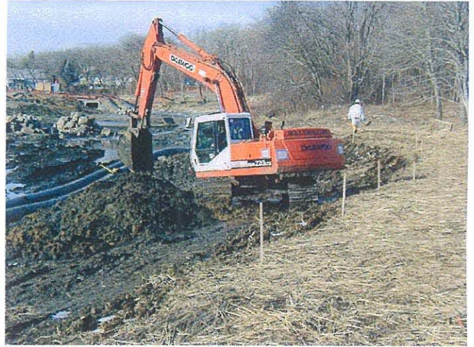
Excavation on the east shore near Titleist lot Photo # WS2502 2/5/03 JPK
