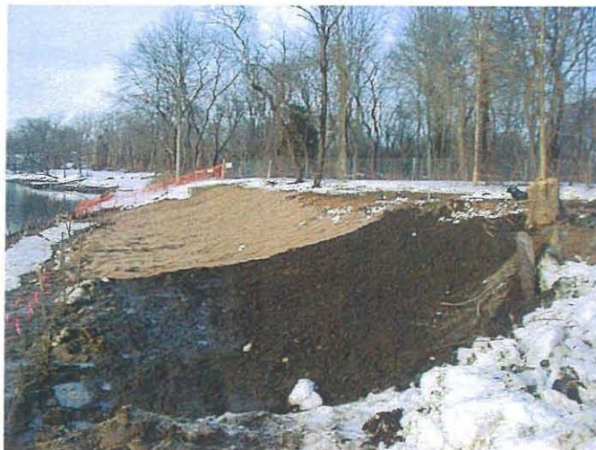
Restoration of the excavation at the Acushnet Park Photo # NWS121204 12/12/03 MS
