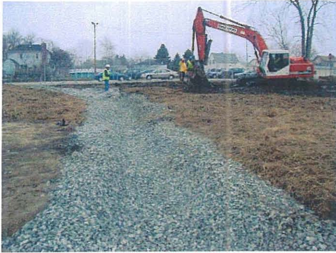
Construction of drainage swale north of Tieleist lot Photo # WS40701 4/07/03 JPK
