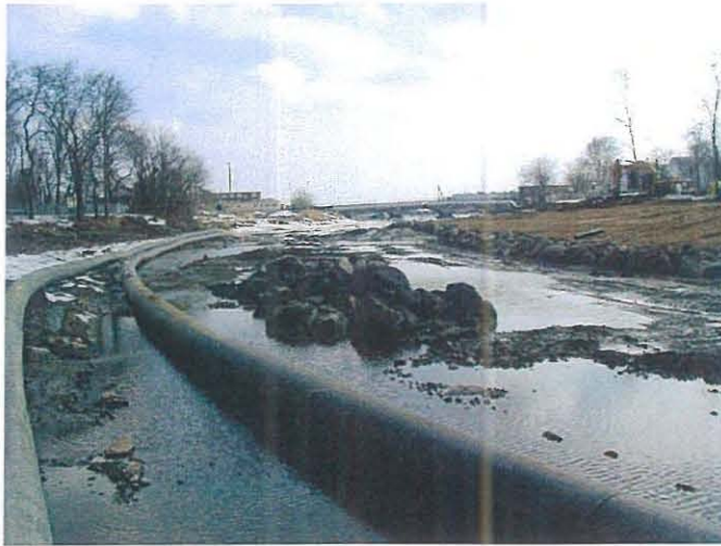
View downstream from N. berm-restoration underway
