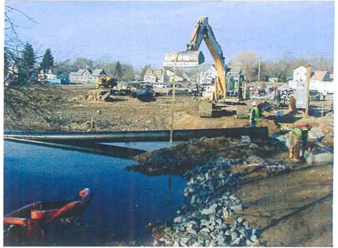
Removal of the by-pass piping from river Photo # WS32005 3/20/03 JPK
