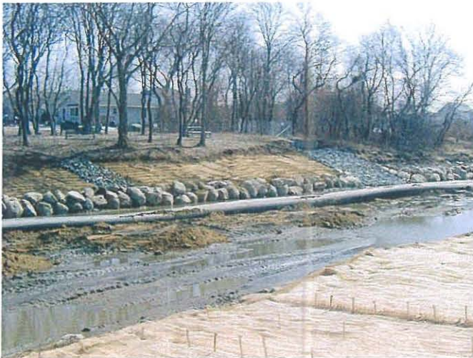
Restoration of eastern shoreline at Acushnet park
