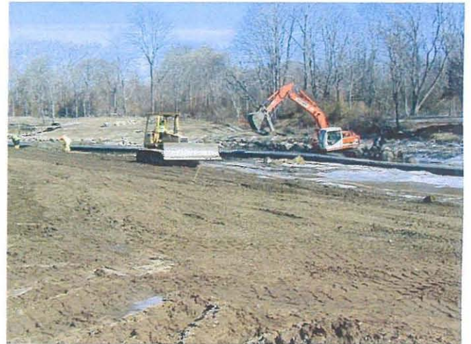
Stone toe/topsoil placement at the lumberyard zone Photo # WS31101 3/11/03 JPK
