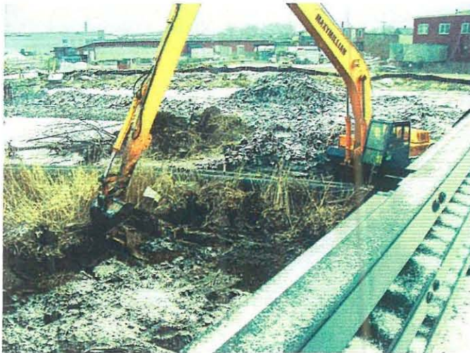
Excavation in south zone near Titleist (east shore)
