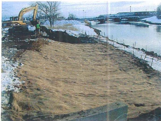
Restoration of the excavation at the Acushnet Park Photo # NWS121203 12/12/03 MS
