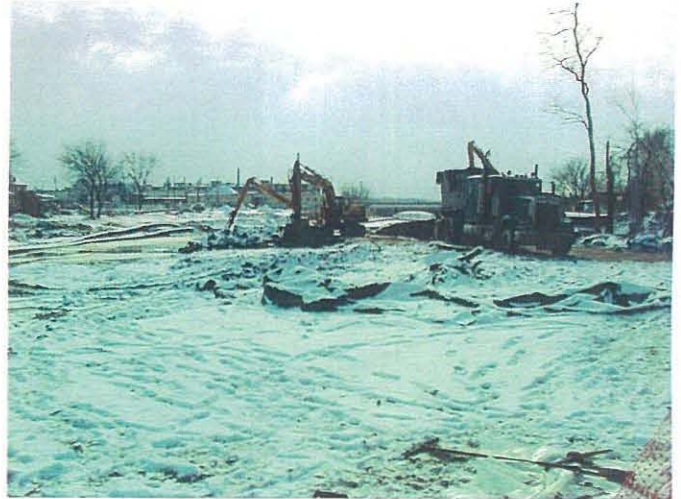
In-river excavation and sediment load-out operations Photo # WS11701 1/17/03 JPK
