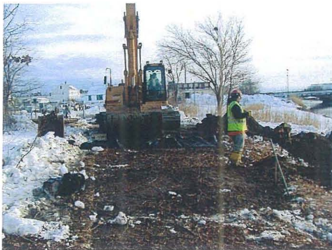
Removal of HDPE mats south of excavation at Acushnet Park Photo # NWS121201 12/12/03 MS
