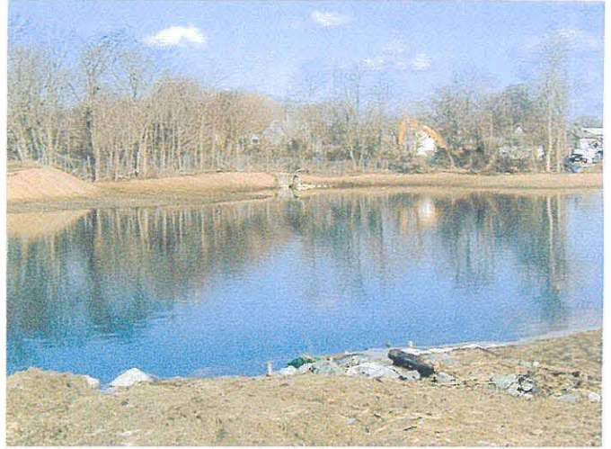
CSO outlet near high tide Photo # WS40101 4/01/03 JPK
