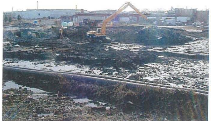
Excavation of the South Zone Photo # WS2302 2/3/03 JPK
