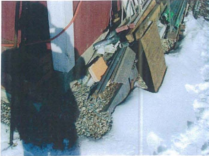
Santos shed – pre-excitation conditions Photo # WS21307 2/13/03 JPK
