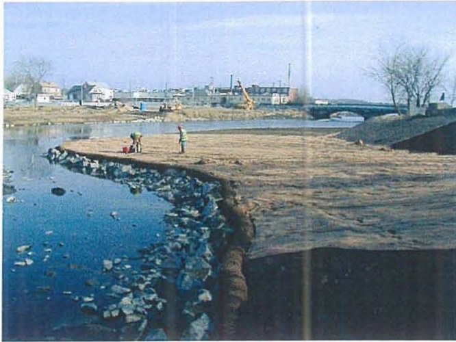
Restoration activities at the CSO zone Photo # WS31805 3/18/03 JPK
