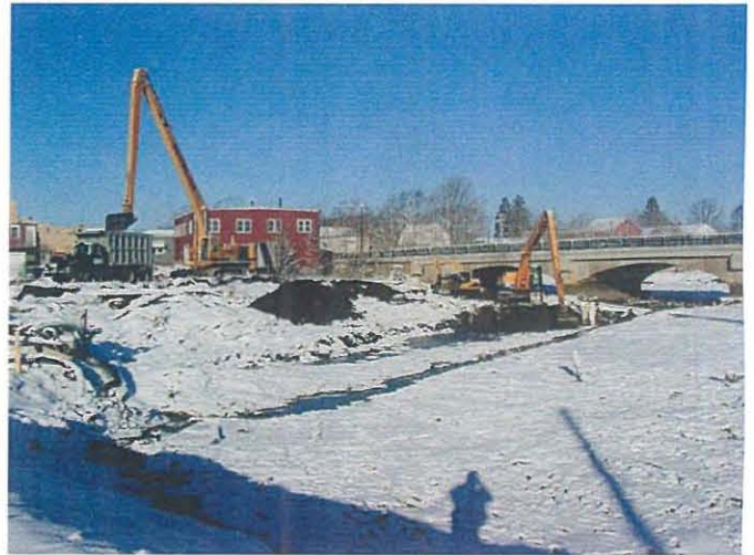
Excavation activities in the south zone Photo # WS21102 2/11/03 JPK
