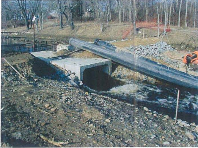
River flowing through the north berm culvert Photo # WS31801 3/18/03 JPK
