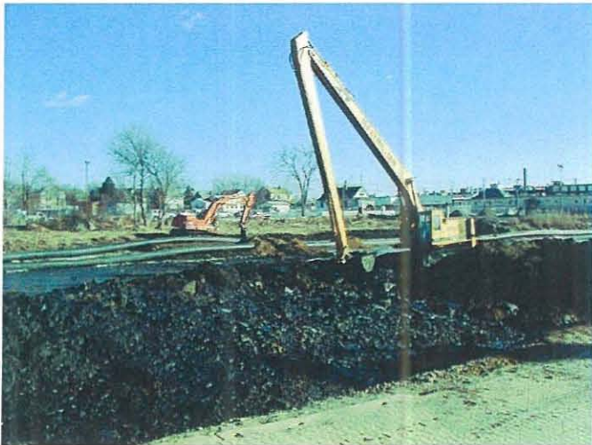
In-river excavation at the CSO/mudflat zone
