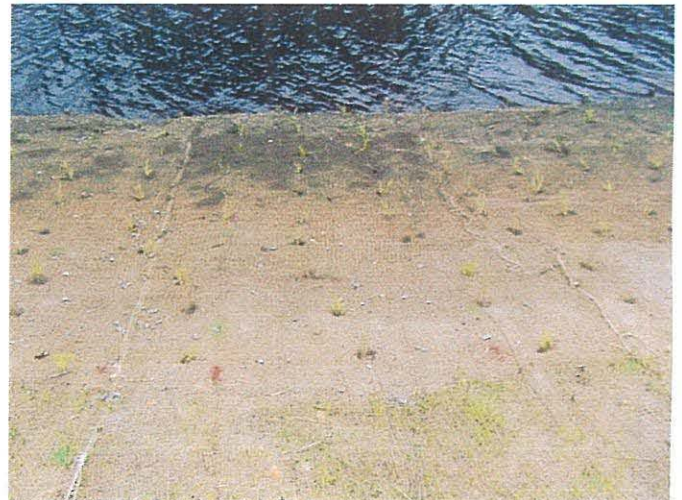
Wetland planting in lumberyard area Photo # WS61113 6/11/03
