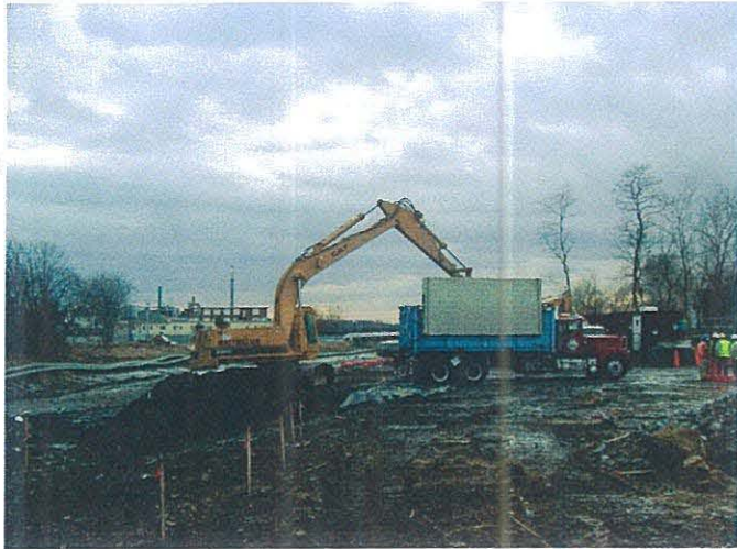
Load-out of sediments into trucks for transport to DDA Photo # WS1903 1/9/03 JPK
