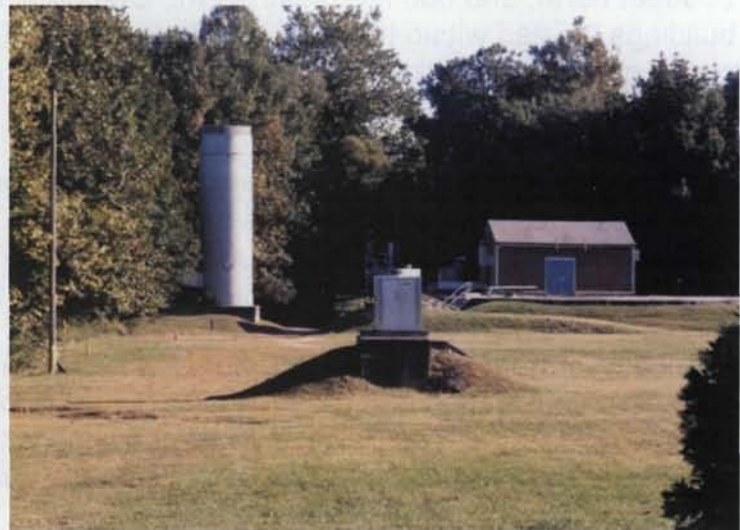
Municipal well field with treatment system
