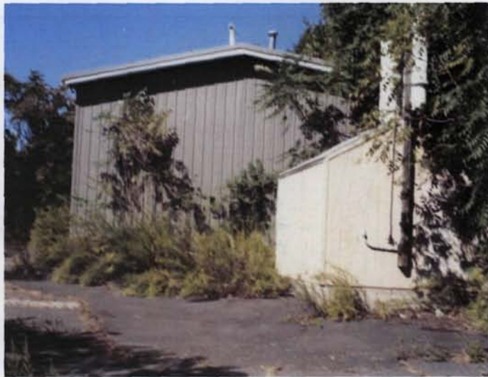
Treatment Building behind Zell Buildings
