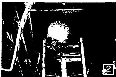
1 – Res. eng. Skip Parker sits in TBM operator's seat before placement of screw conveyor which will protrude from that hole in the middle. 2 – Worker uses torch to cut entryway through sheetpiling of shaft for tunnel boring machine. 3 – Photo looking towards front (cutting end) of TBM during operation shows enclosed screw conveyor, which is carrying muck to rail haul system at rear. 4 – Standing with Akkerman TBM before assembly in shaft are, from left, Joseph Bradshaw, vice president of Bradshaw Contracting, and Richard Michael, project manager for Dufresne-Henry.
